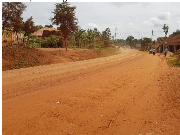
1+700: Gravel section of the road
