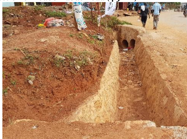
Ch. 0+040: Drainage works
