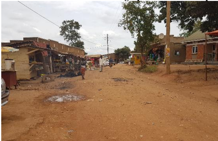
Ch. 0+000: Project information signage at start of road link
