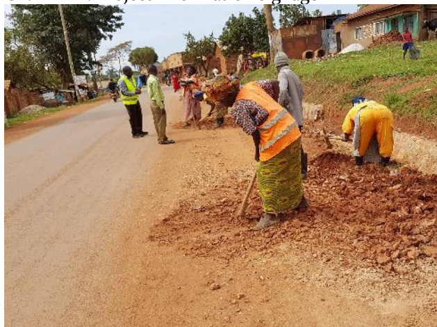
0+600: Active routine manual maintenance and drainage works
