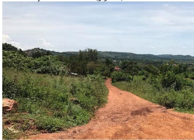
Ch. 2+500: Urgent cross culvert installation required
