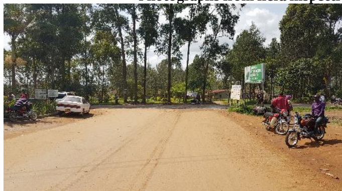
Ch. 0+000: Drainage improvement required via installation of open drift
