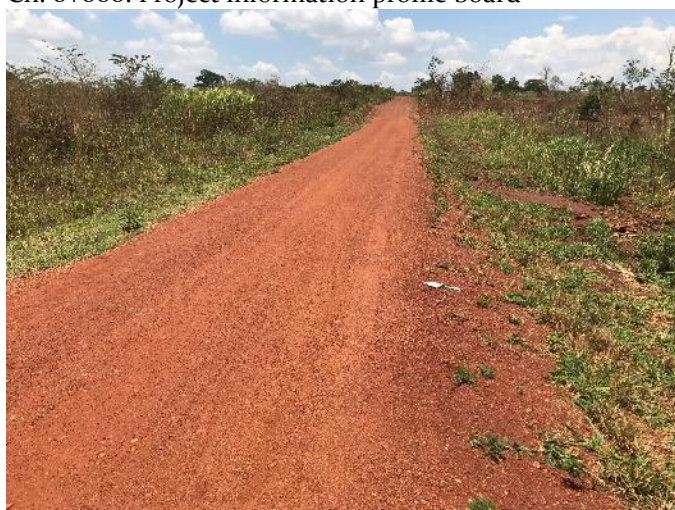
Ch. 2+400: Gravel fill at a swamp
