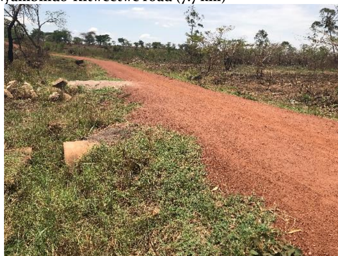
Ch. 1+800: Culvert installation without end structures
