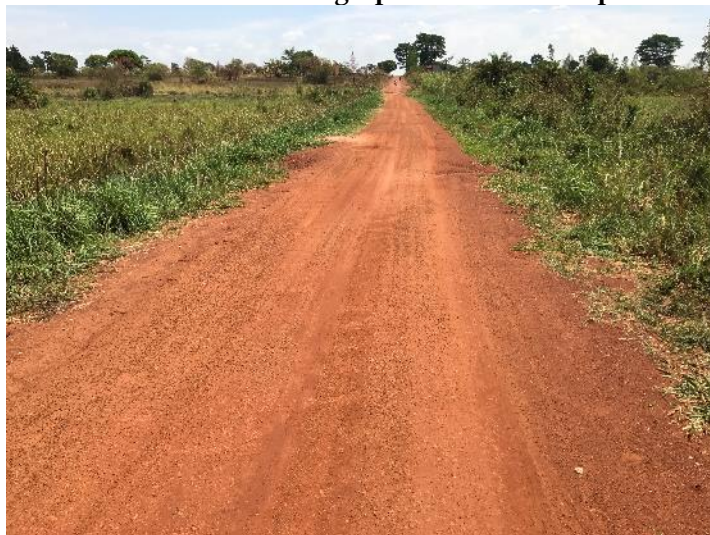
Ch. 4+300: Gravelling earthworks in swamp section
