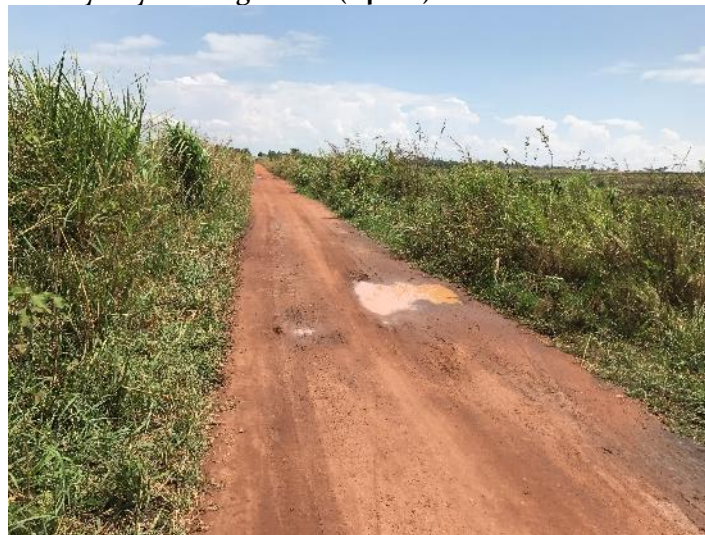
Ch. 9+400: Lack of routine manual maintenance
