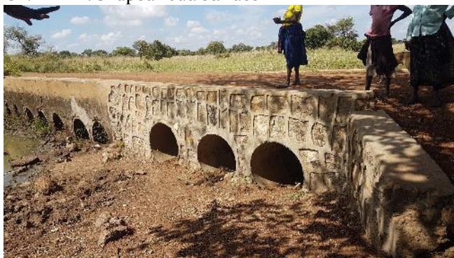
Ch. 10+100: Multiple culvert installations at a stream crossing.
