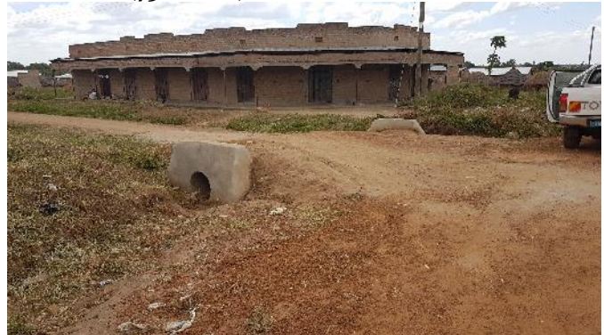
0+400: Access culvert installation with Silty backfill
