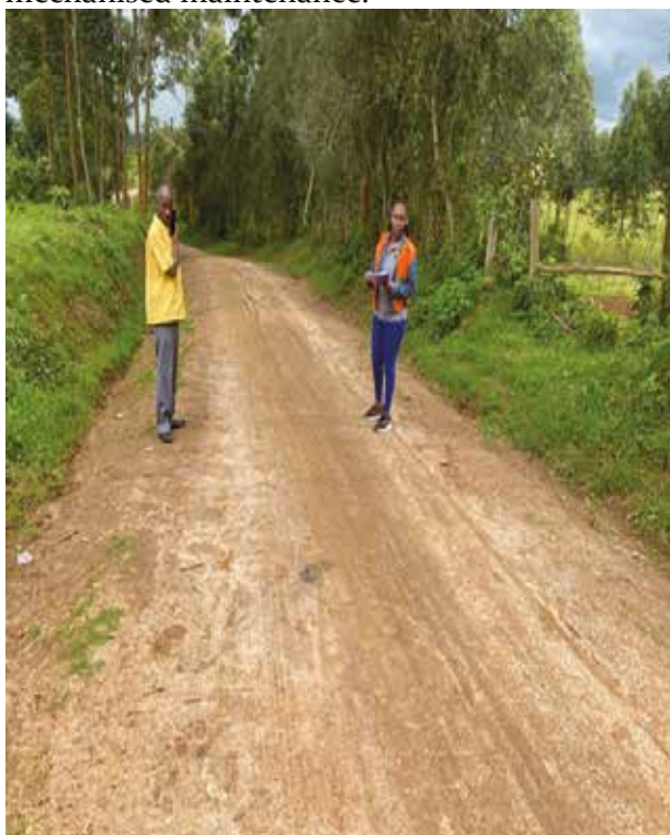
Nyamabaare-Marumba road (2.68 km) underwent heavy grading, shaping, and spot gravelling under routine mechanised maintenance.
