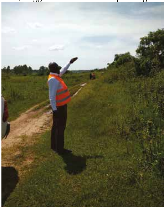
Dokolo district: Beibil – Barlela road –overgrown vegetation forming canopy & narrowing the road; clogged drains and water ponding along the road due to lack of culverts/cross drains.
