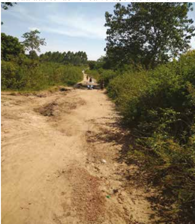
Dokolo district: Beibil – Barlela road –overgrown vegetation forming canopy & narrowing the road; clogged drains and water ponding along the road due to lack of culverts/cross drains.
