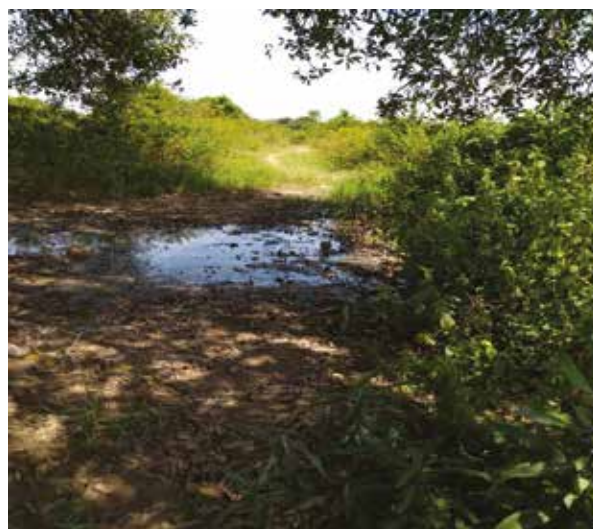
Dokolo district: Beibil – Barlela road –overgrown vegetation forming canopy & narrowing the road; clogged drains and water ponding along the road due to lack of culverts/cross drains.
