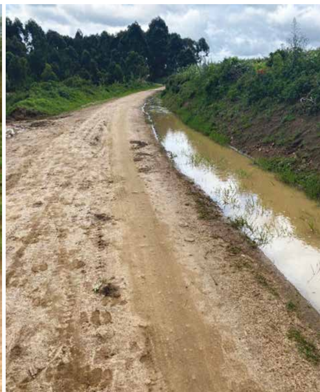
Nyamabaare-Marumba road (2.68 km) underwent heavy grading, shaping, and spot gravelling under routine mechanised maintenance.
