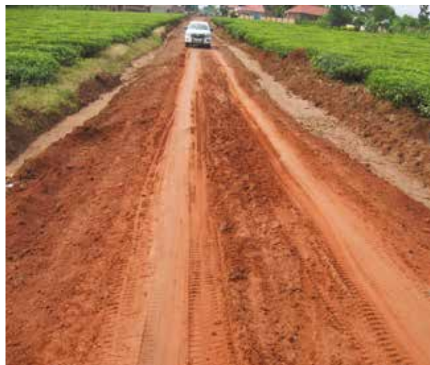
Mukono district: Spot-gravelled section on Kabembe-Nakibano road (9 km) under routine mechanised maintenance.
