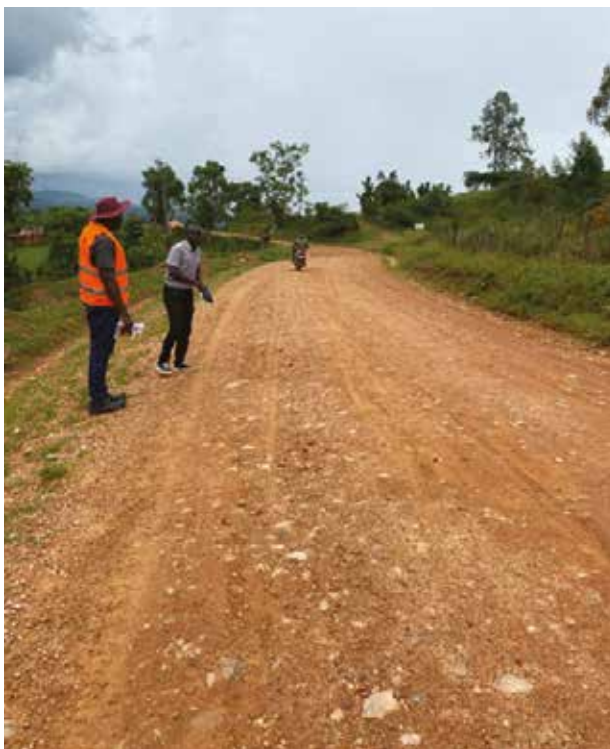
Rukungiri-Mitaano-Kanungu road (44 km) underwent heavy grading for 10 km under routine mechanised maintenance. However, some sections of the road required drainage improvement.
