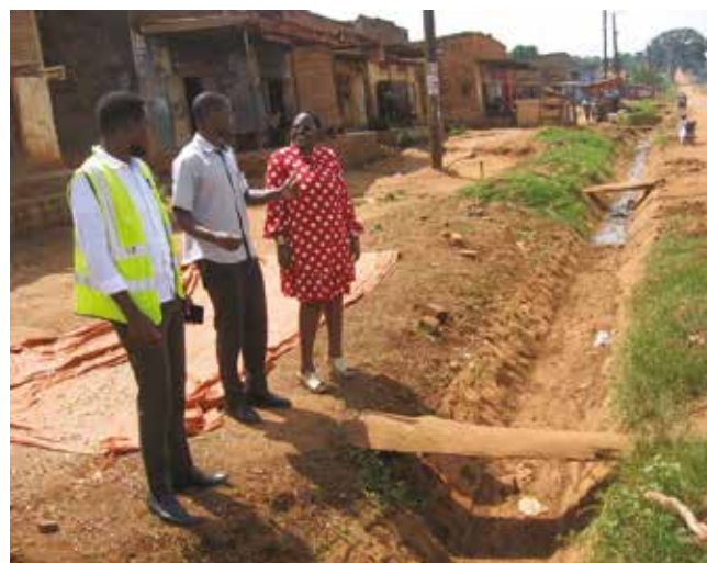
UNRA Mpigi: Side drains cleaned of debris by LBCs on Mitalamaria Loop (4.3 km) under routine manual maintenance.
