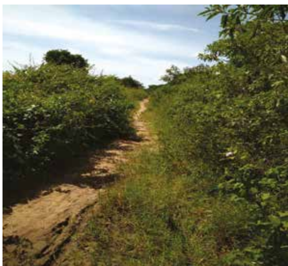
Dokolo district: Beibil – Barlela road –overgrown vegetation forming canopy & narrowing the road; clogged drains and water ponding along the road due to lack of culverts/cross drains.
