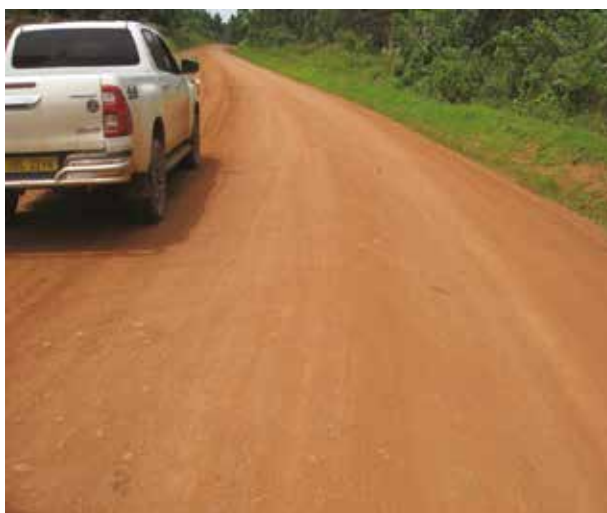
UNRA Mpigi: A graded section on Mitala Maria-Bulo-Kanoni road (29.6 km) under routine mechanised maintenance.
