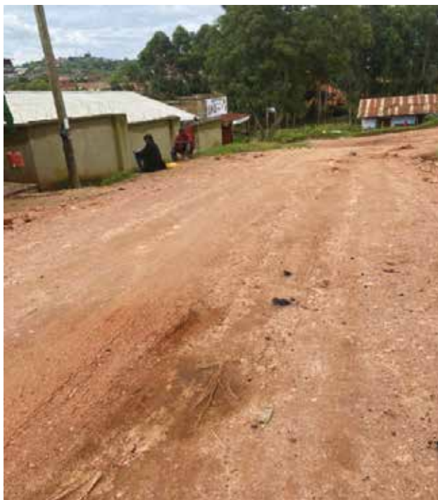
Kayembe road (1.68 km) underwent heavy grading, shaping, and spot gravelling under routine mechanised maintenance.
