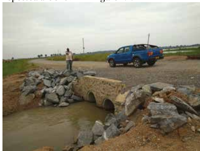
UNRA Arua: Emergency repairs of washout undertaken on the approach to Pakwach bridge on Olwiyo – Pakwach road.
