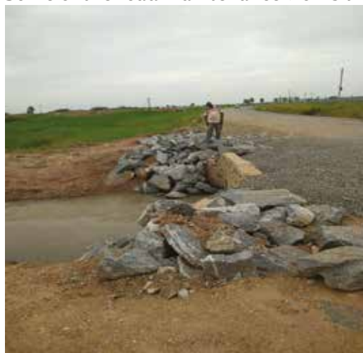
UNRA Arua: Emergency repairs of washout undertaken on the approach to Pakwach bridge on Olwiyo – Pakwach road.
