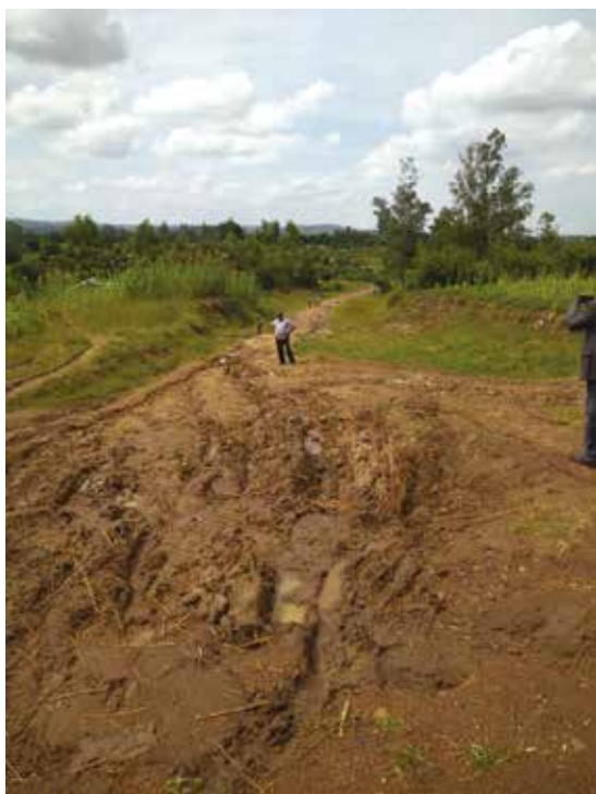
Terego District: Section of Agurua – Alikua road in a poor state and a bottleneck. Failures due to poor drainage in a water-logged area. Catchwater drains and deep side drains
