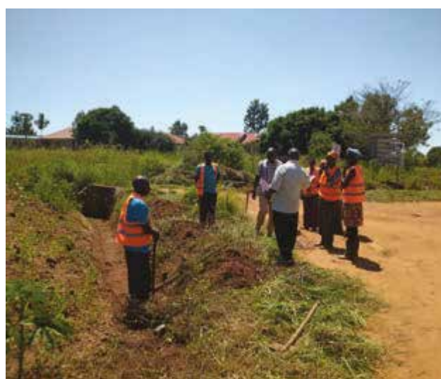
Kitgum MC: Road gangs opening side drains at ch 0+300 along Pandwong road in Pandwong division.
