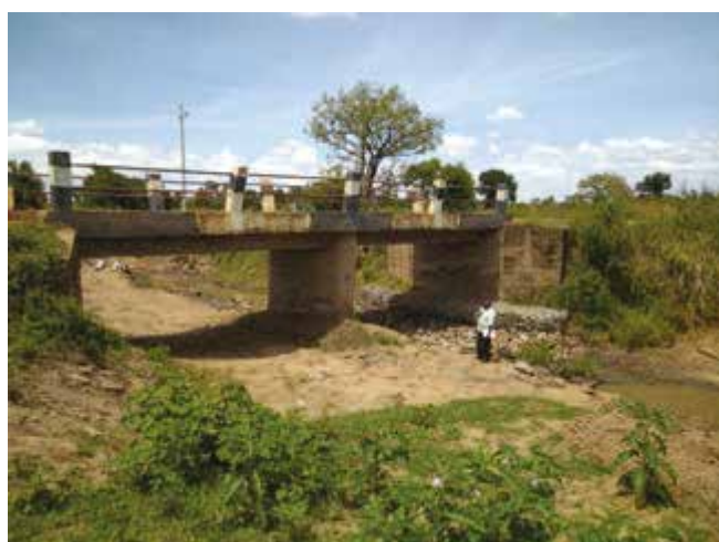
Kitgum district: A composite bridge at ch 4+600 along Ayom – Alune road where gabion protection works were done to prevent undermining of the bridge abutment; river training carried out to re-direct water through the river channel.
