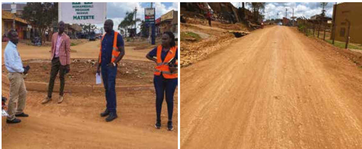
Mateete-Mbirizi road (17.2 km) underwent grading and spot gaveling using framework contracting under routine mechanized maintenance.
