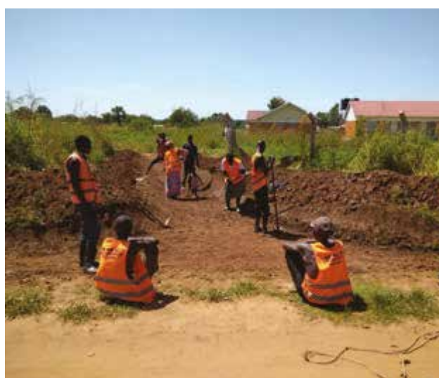
Kitgum MC: Road gangs opening offshoots at ch 0+100 along Abubakar Muhamed road in Pandwong division.
