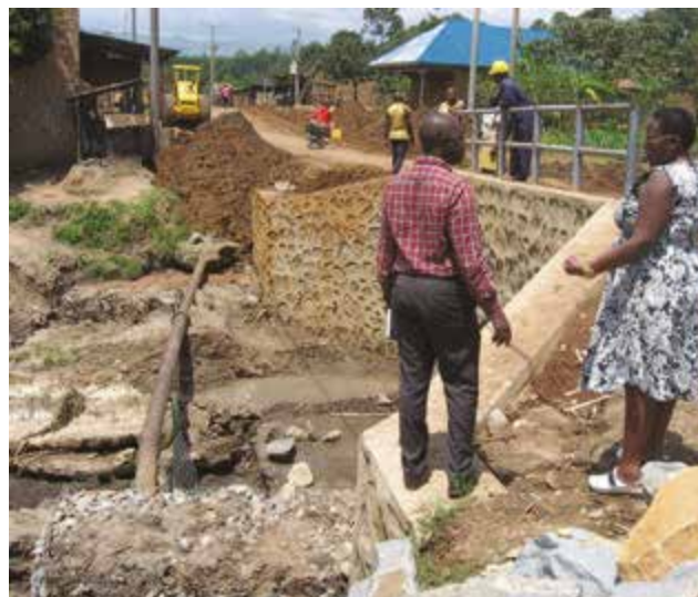
Manafwa district: Construction of a major drainage structure of 3 lines of \Phi 1.8 m steel culverts on Bukhaweka-Butiru road (8.8 km) with retaining structures under periodic maintenance.
