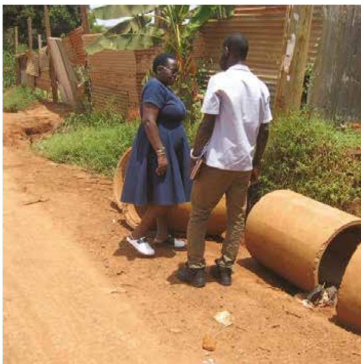
Kira MC: Reinforced concrete culvert rings to be used for installation of a relief cross culvert on Lusirika road (1 km) under periodic maintenance.
