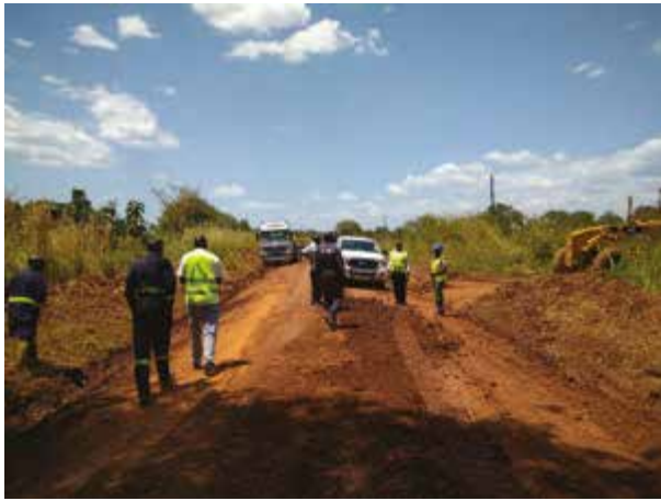
UNRA Kitgum: Grading works and spot gravelling along Matidi-Kalongo-Patongo road (77 km).
