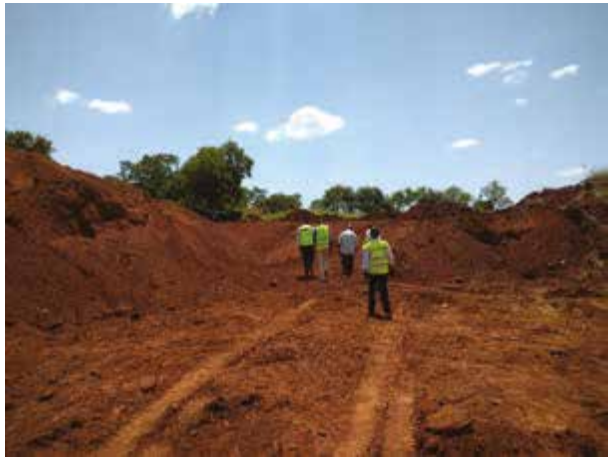
UNRA Kitgum: Excavation and stockpiling of gravel at borrow pit for spot gravelling of Matidi-Kalongo-Patongo road (77 km).
