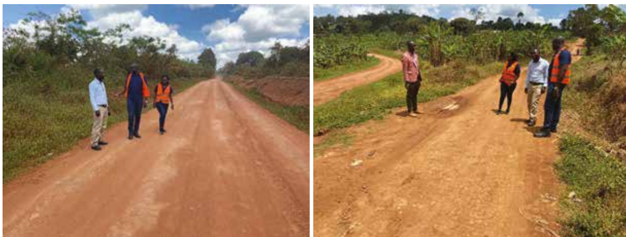
Kyabakuza-Mateete-Kaliro road (70 km) underwent surface grading and spot graveling on 30 km under routine mechanized maintenance. However, one of the sections of the road needed installation of cross culverts.
