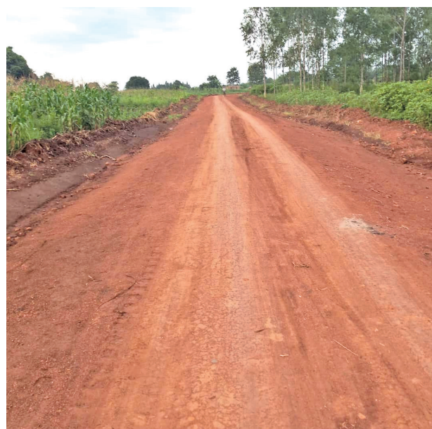
Kole District: Teobia-Widam-Olaka Annex road (7.7 km), Work in progress - Periodic maintenance.
