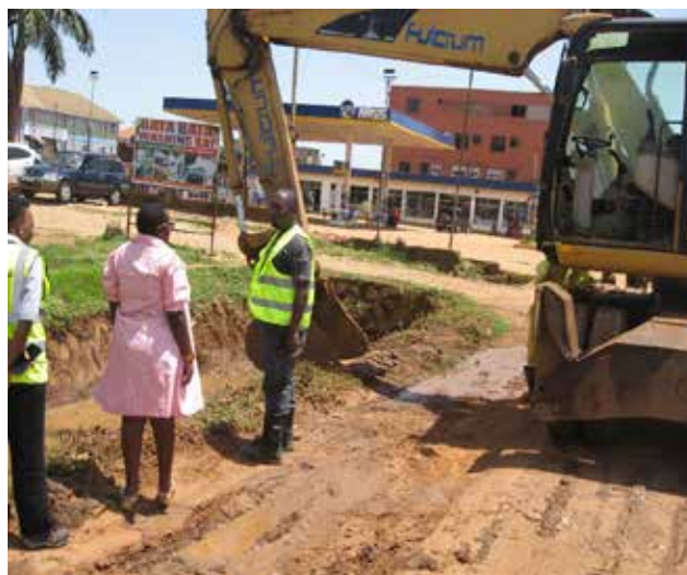
UNRA Kampala: Kibuye-Zana-Mpala road (20 km) under RMeM by framework contracting. Contractor was unclogging side drains using a wheeled excavator.
