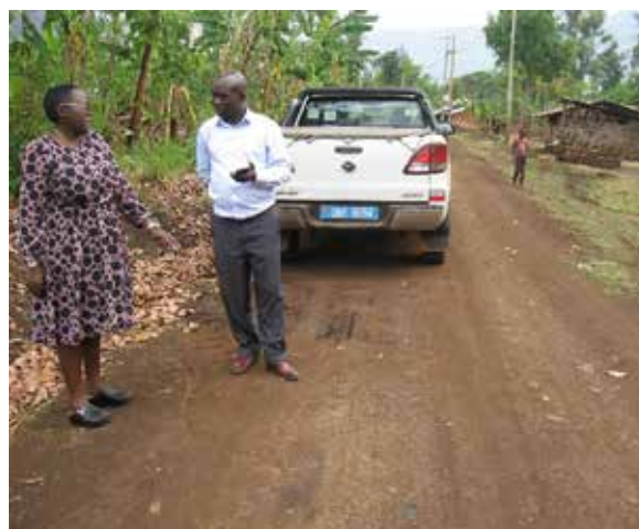
Bulambuli district: Gidoi-Pondo road (3 km) cleared of vegetation and reshaped under routine mechanised maintenance.
