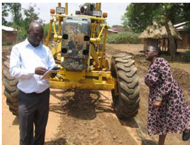
Bulambuli district: Grading of Nabbongo-Buwasheba road (5 km) under routine mechanised maintenance.
