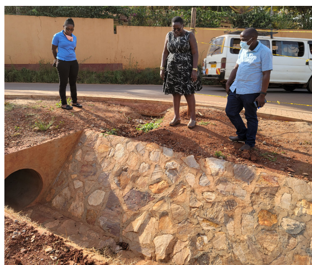
Makindye Ssabagabo MC: Cross-drainage culverts installed on Lubowa Lower Quality road (2.7 km) under extended periodic maintenance.
