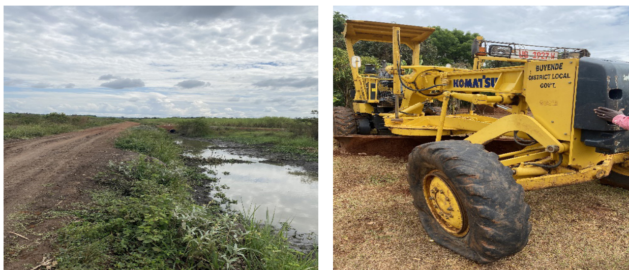
Buyende district: Road embankment built over swamp crossing on Nabitula-Inuula-Kabale road (12 km) and a grader with deflated tyre –broken down along Gwase-Wagawaga-Idome (14 km).
