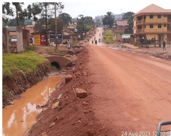
Gravel fill in raised section – Muzito Road
