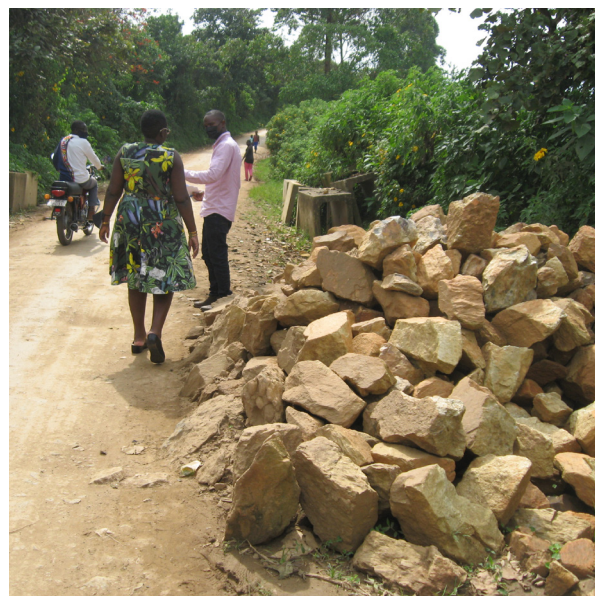
UNRA Fort portal: Stockpiles of materials for Kigarama-Gweri-Harubaho-Verika road (13 km) under RMeM maintenance using FA.
