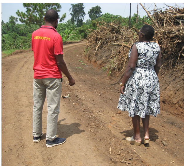
Fort portal City: Bush clearing and grading of Kyaruhaga road (0.5 km) under RMeM maintenance.
