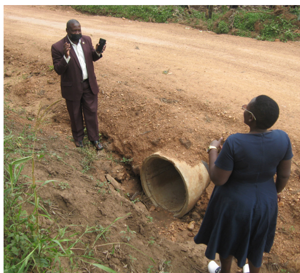
Isingiro district: Cross-drainage culverts being installed on Kagogo-Kigyende road (10 km) under routine mechanised maintenance.
