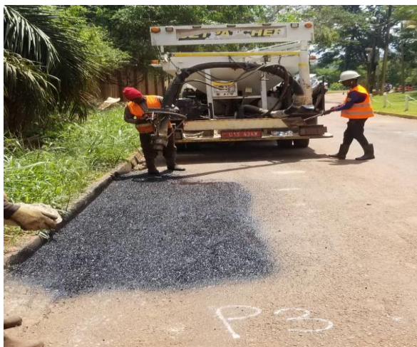
Fig. 3.1.1: Jet patching in progress – Nyonyi Garden's Road
