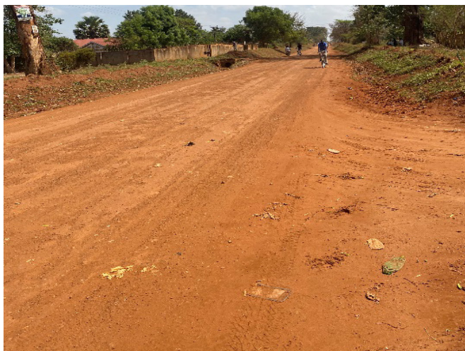
UNRA Soroti: Grading works done along Soroti-Serere road (27 km)
