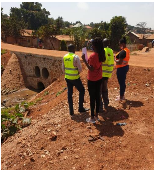
Additional culverts constructed to cope with peak floods – Kizanyiro road.
