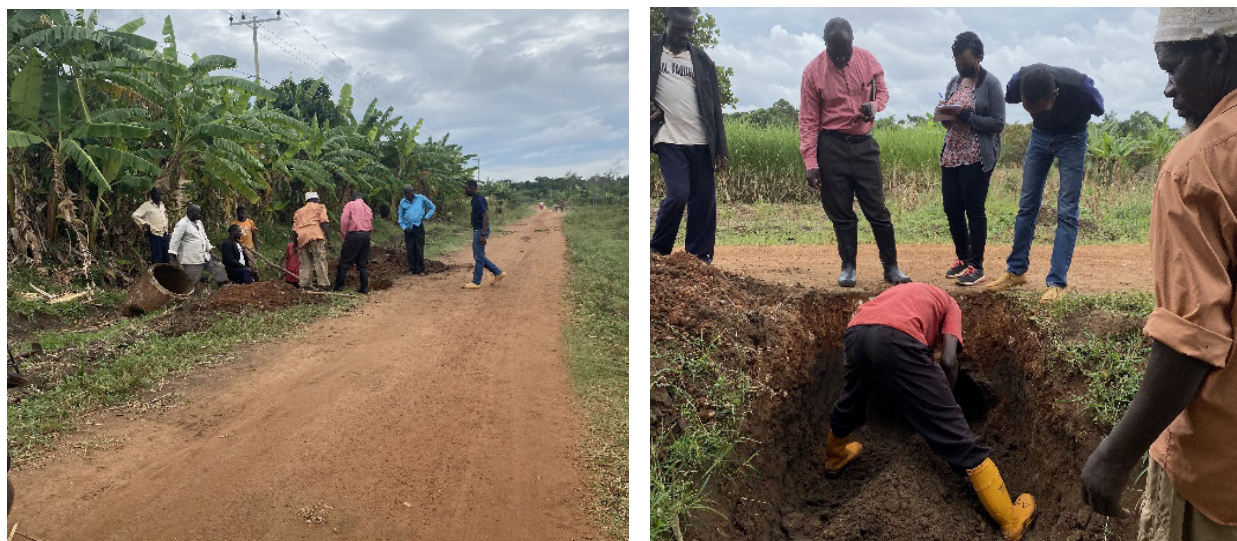
Buyende district: Culvert replacement along Nakabira-Bugaya road (12.5 km) using road gangs.
