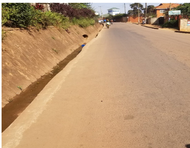
Repaired side drains – Kaweesa Road
