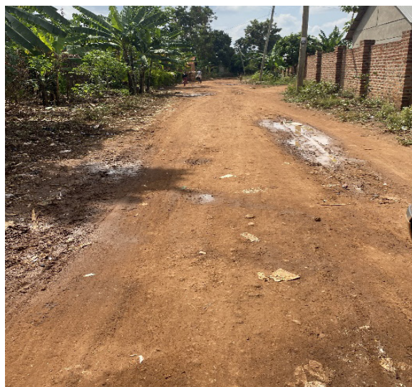
Kaliro Town Council: Shaping and Drainage works needed along Gamutambula road (0.35 km) and Sanya road (1.5 km) in Kaliro TC.
