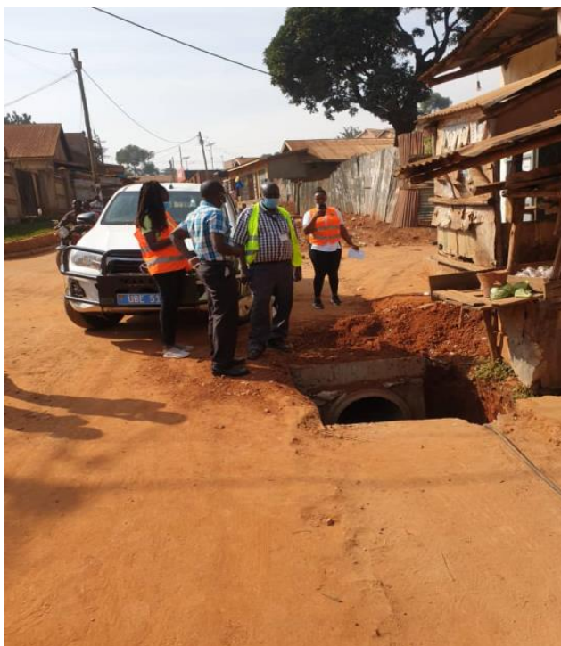
Inspection of manhole under construction – Bibiyana road
