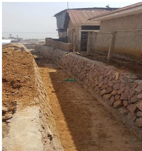
Outflow channel constructed to convey water from Ggaba By-pass road to Lake Victoria
