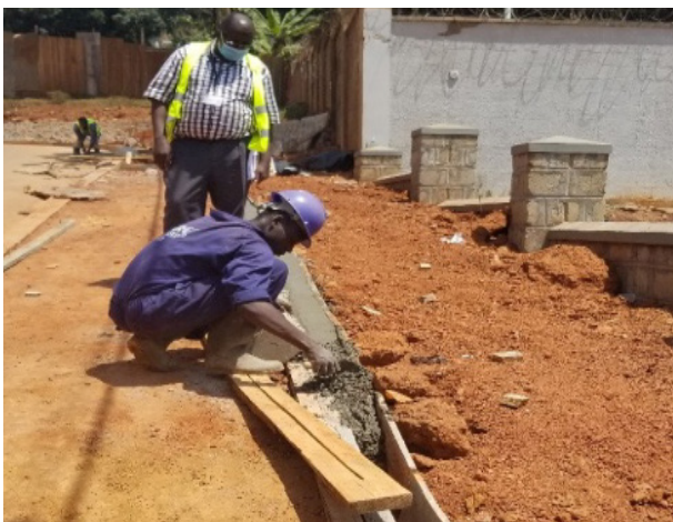
Construction of edge beam for walkways - Naguru Drive Close
