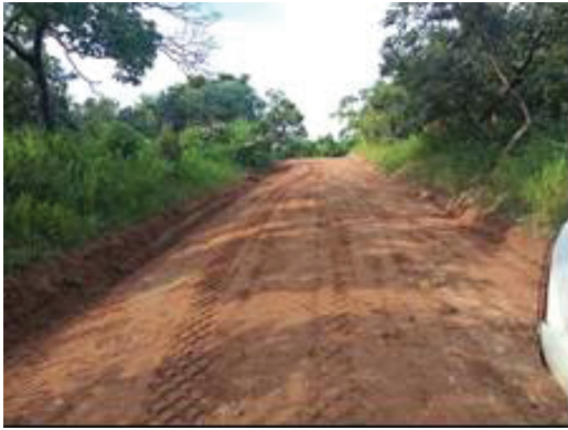
Routine mechanised maintenance (RMeM) of Metu-Goopi Rd (4.54km) involving bush clearing, drainage works, stream training and spot gravelling
