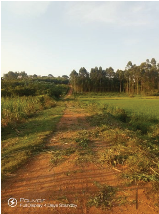
Lwengo district: Nkoni-Nabyewanga road (5 km) - During grass cutting, desilting, and pothole filling under routine manual maintenance.
