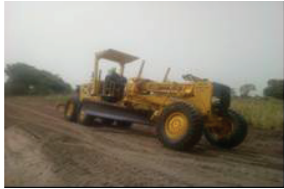
RMeM of Ebgwea – Lereze – Kolokolo Rd (6.1km) involving bush clearing and road formation, drainage works, filling of approach to box culvert and spot gravelling works.
