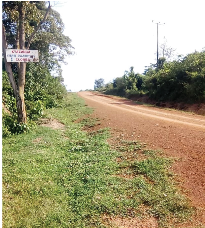
Lwengo district: Nkoni-Nabyewanga road (5 km) - After grass cutting, desilting, and pothole filling under routine manual maintenance.
