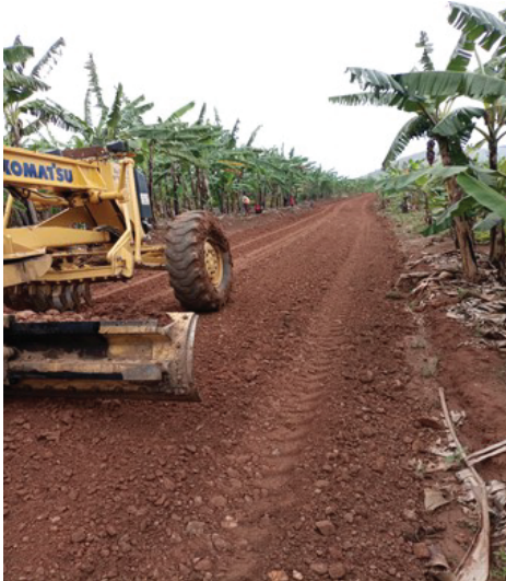
Mbarara district: Regravelling a section on Bwizibwera-Mabira-Kitookye-Rwenshaku road (19 km) under RMeM.
