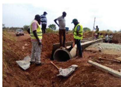
Culvert installation along Adjumani-Mungula - Amuru (88km)
