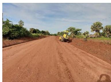
Final compaction along Moyo - Yumbe Road (66km)
