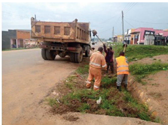
UNRA Ibanda: Desilting of side drainage system of Nyakahita-Kazo-Ibanda road (68 km) under routine maintenance.
