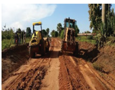
Grading works along Ure - Kulikulinga - Yumbe Road (25km)
