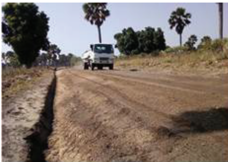
Routine mechanised maintenance (RMeM) of Metu-Goopi Rd (4.54km) involving bush clearing, drainage works, stream training and spot gravelling
