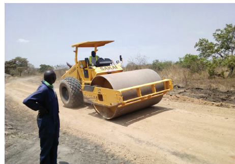
Routine Mechanised maintenance of Lefori – Chinyi Rd (12km) and Lefori – Kali Rd (7km) involving involving bush clearance and formation, drainage works, stream training and spot gravelling
