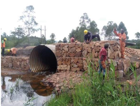
UNRA Ibanda: Emergency culvert installation including fill and gabion works on Ruhumba-Byanamira-Kaswa road (31.3 km).
