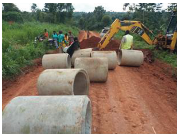
Mityana MC: Culvert installation on a section on Bukoma-Nalule road (3.7 km) under emergency works.
