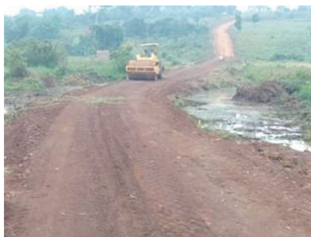
Mityana MC: A swamp section raised and well compacted on Mitimboje-Kilungu-Jingo-Kambuzi road (5.6 km) under emergency works.
