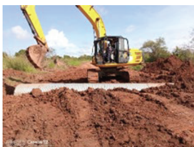
Culvert installation along Obongi - Kulikulinga Road (45km)
