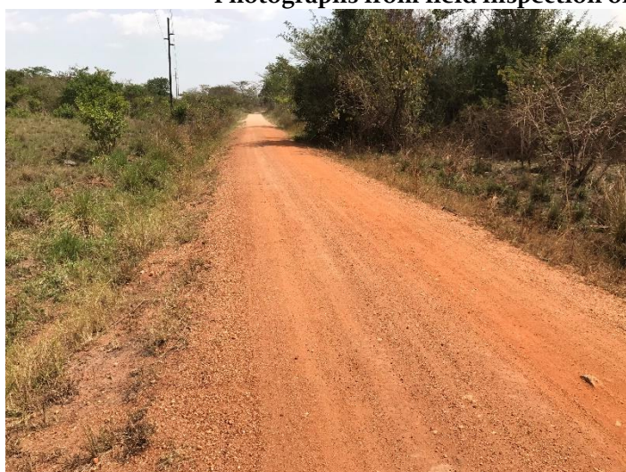
Ch. 2+200: A spot gravelled section
