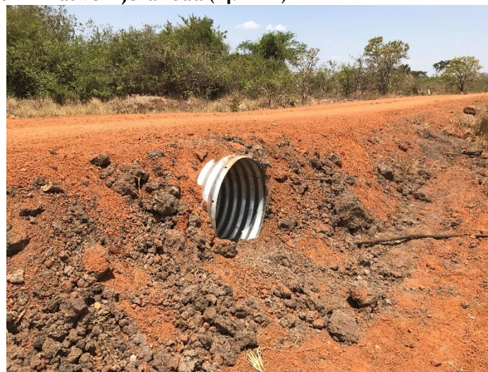
Ch. 8+200: Failure to construct headwalls on the installed Armco cross culverts
