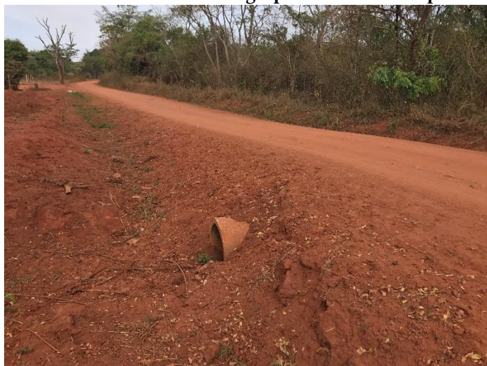
Ch. 4+400: Failure to construct headwalls on the installed cross culverts
