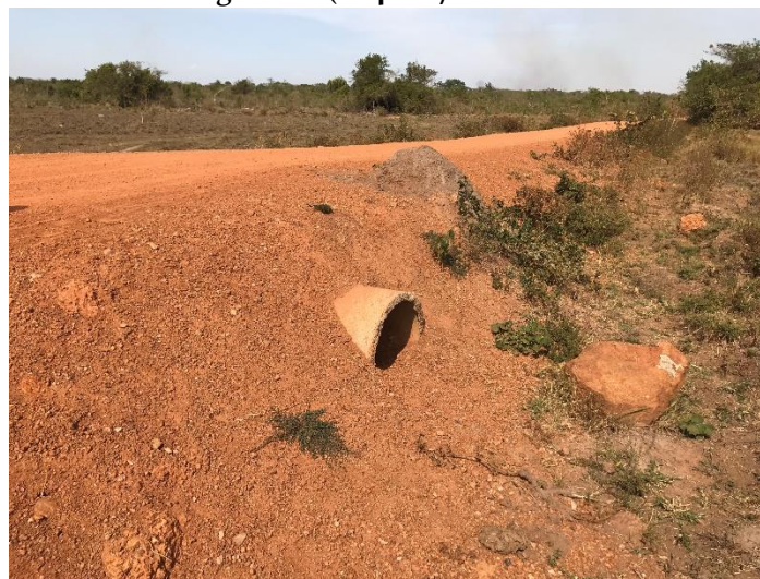
Ch. 8+900: Failure to construct headwalls on the installed cross culverts
