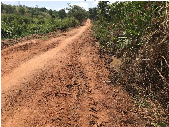
Ch. 0+900: A low-lying swampy area requiring drainage improvement via multiple culvert installation and fill earthworks
