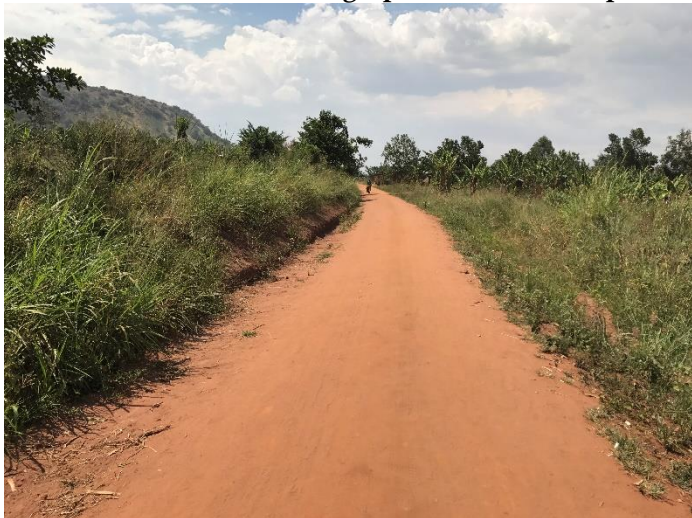
Ch. 8+100: A shaped section without mitre drain provisions
