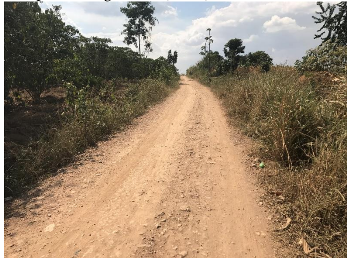
Ch. 14+400: Spot gravelled section with overly grown vegetation as a result of inadequate routine manual maintenance
