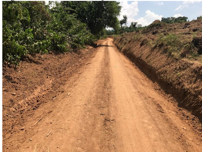
Ch. 2+200: A shaped section without mitre drain provisions
