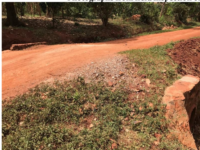
Ch. 2+600: Inadequately compacted inferior culvert backfill material
