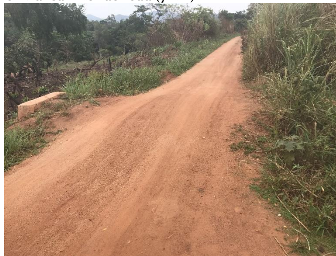
Ch. 3+200: Poor compaction of culvert backfill and lack of routine manual maintenance
