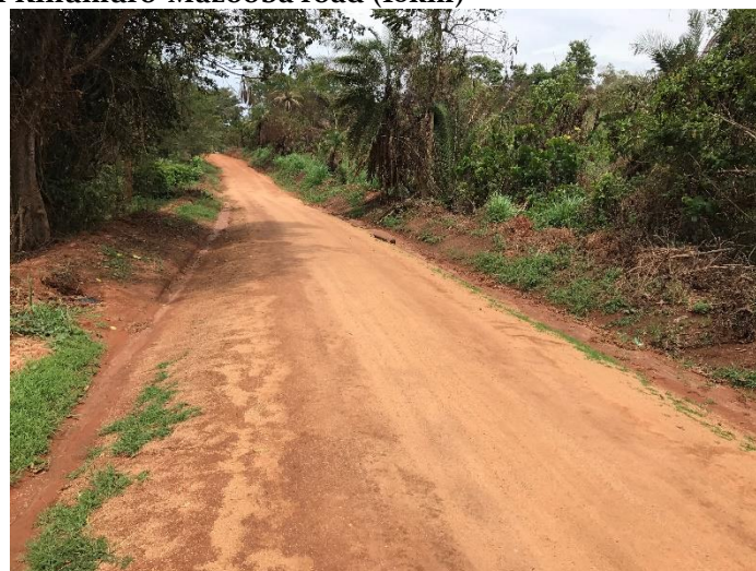
Ch. 6+300: Lack of drainage offshoots
