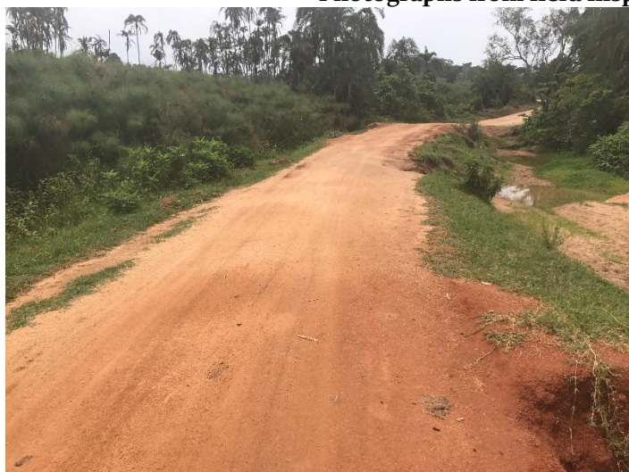
Fill material along the approach road
