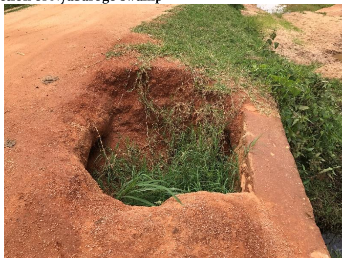
Broken culvert piece
