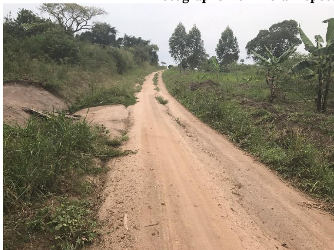
Ch. 1+400: Gullies as a result of inadequate drainage provisions
