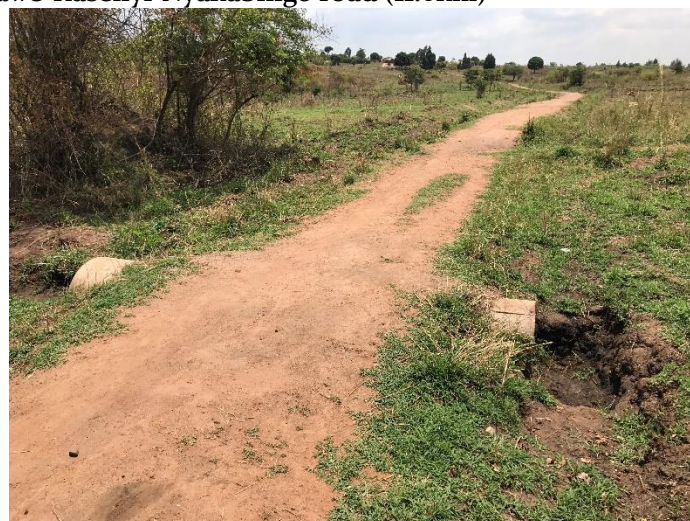
Ch. 5+200: Culvert installation with end structures and narrow carriageway
