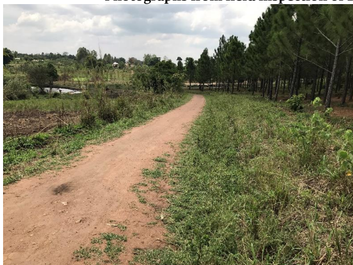
Ch. 3+400: A previously shaped section with overly grown vegetation as a result of inadequate routine manual maintenance
