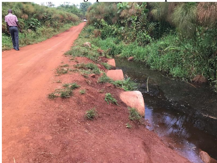
Installed concrete culverts without end structures
