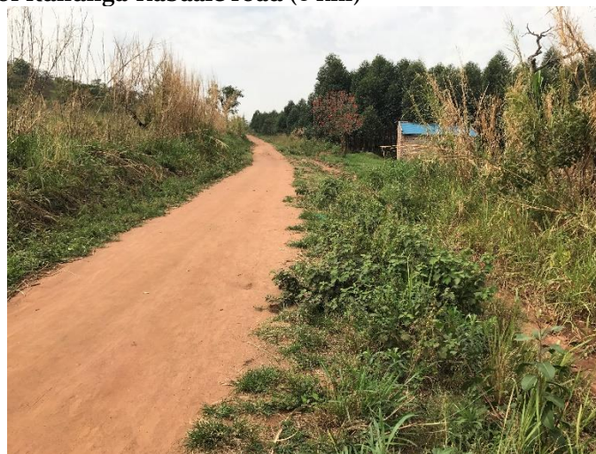
Ch. 5+500: Lack of offshoots over long stretches
