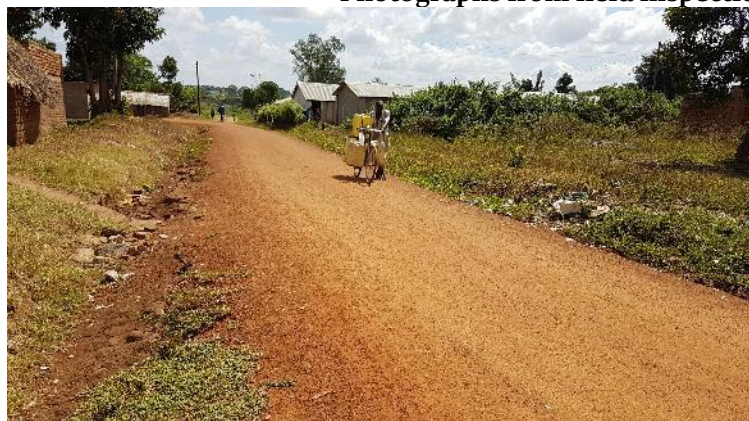
Ch. 0+050: Stone pitching required for side drains
