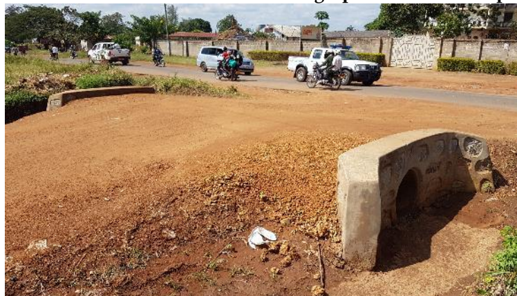
Ch. 0+000: Access culvert installation
