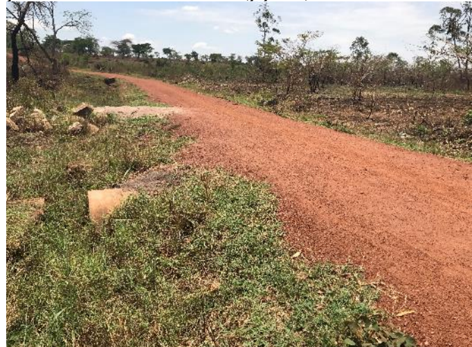
Ch. 1+800: Culvert installation without end structures
