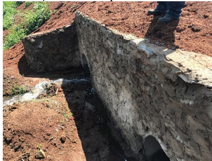
Poorly constructed splash aprons
