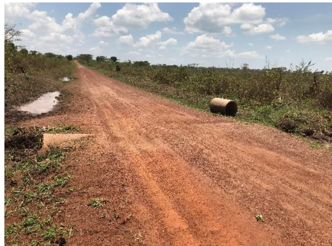
Ch. 6+200: Culvert installation without end structures, inadequate backfill and idle culvert pieces
