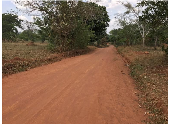
Ch. 3+700: Inadequate provision of mitre drains
