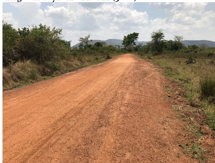
Ch. 4+900: A low-lying area susceptible to flooding requiring improvement by filling
