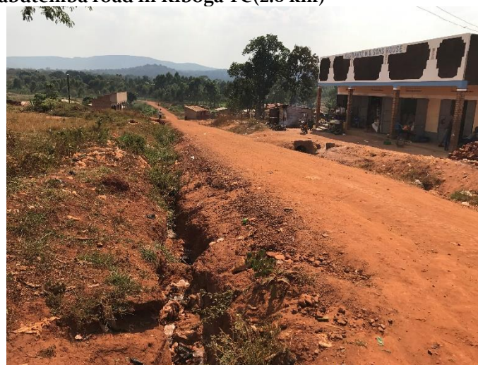
Ch. 0+150: Side drains requiring urgent stone pitching
