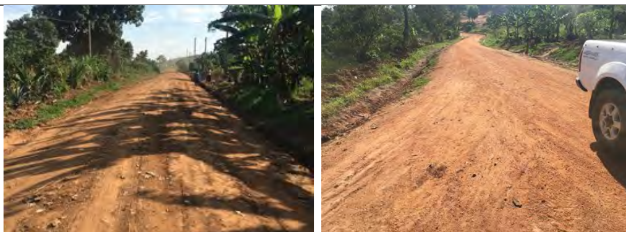
Namilali –Ssembwa district road under routine mechanised maintenance. Ongoing works included grading, spot gravelling and swamp filling.
