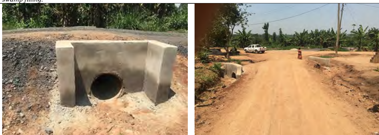
2 lines of concrete culverts with headwalls were installed on SDA Kambugu road and Nkonkonjeru-Kijaguzo road in Semuto Town Council
