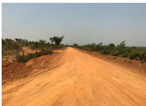
Mulonzi – Nakitoma Rd. was the only district road to receive mechanised maintenance in the period. Works involve grading, spot gravel and swamp raising (approx. 1.5km) as well as drainage works (opening of side drains and culvert installation)
