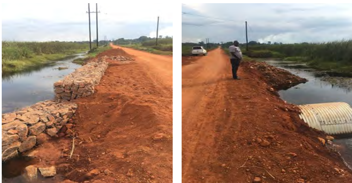
Kapeka – Butalangu (17km) underwent grading and spot improvement using Force Account. The section above (CH16+10) underwent swamp raising involving installation of 2 lines of 1.8m diameter metallic culverts, gabion works and backfill.
