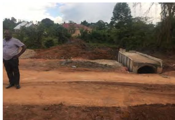
Installation of crossculvert at CH03+10 on Katikamu Kikyusa road by Networld (U) Ltd. The contract involves grading, gravel and drainage improvement.
