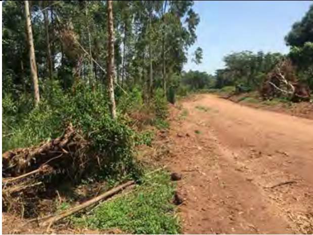
Bakuri Road (1km) and Ssozi Road (1.2km) in Kiwoko Town Council underwent periodic maintenance including widening footpaths, tree removal, grading and compaction
