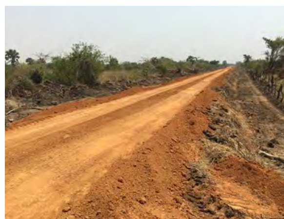
Mulonzi – Nakitoma Rd. was the only district road to receive mechanised maintenance in the period. Works involve grading, spot gravel and swamp raising (approx. 1.5km) as well as drainage works (opening of side drains and culvert installation)
