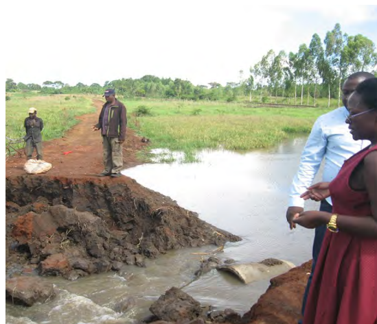
Bugiri district: A bottleneck after stream culverts were washed away by heavy rains on Buwuni - Ntawula road (15.4 km).
