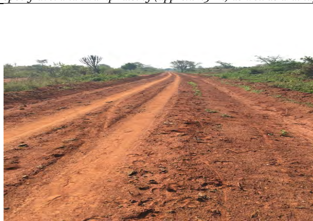
Mulonzi – Nakitoma Rd. was the only district road to receive mechanised maintenance in the period. Works involve grading, spot gravel and swamp raising (approx. 1.5km) as well as drainage works (opening of side drains and culvert installation)
