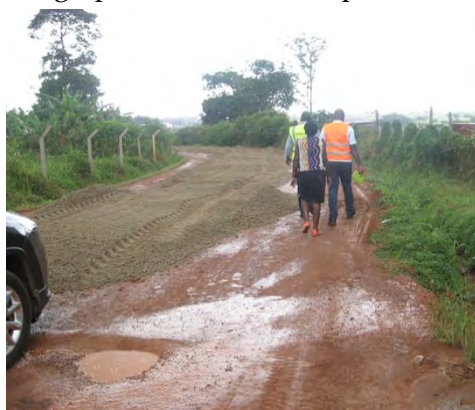
UNRA Kampala: Base course construction on Lweza-Kigo road (5.8 km) under periodic maintenance using a low cost seal.
