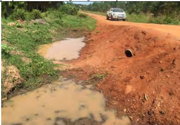
Programme adjustment on Kiwoko –Kasambya to address road washout at CH016+00. Activities including brick making, firewood and sand piles were common along the road due to unclear policy on road reserves.
