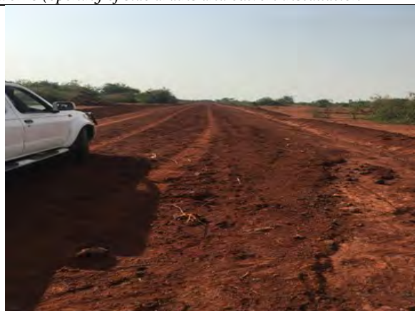
Mulonzi – Nakitoma Rd. was the only district road to receive mechanised maintenance in the period. Works involve grading, spot gravel and swamp raising (approx. 1.5km) as well as drainage works (opening of side drains and culvert installation)
