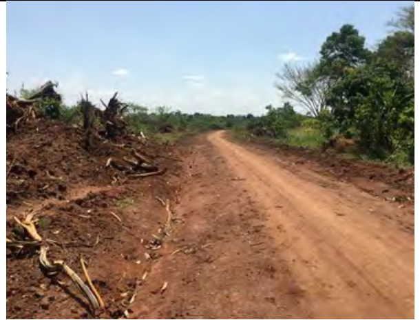
Bakuri Road (1km) and Ssozi Road (1.2km) in Kiwoko Town Council underwent periodic maintenance including widening footpaths, tree removal, grading and compaction
