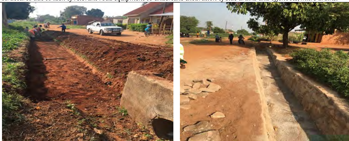
Ongoing routine manual maintenance and stone pitching of side drains along Kiwewa Rd in Migeera Town Council
