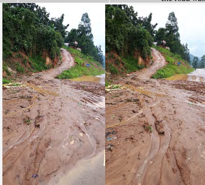
Typical Section of Silting Observed on Kabale – Katuna Road
