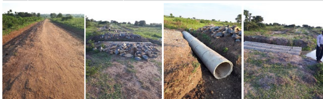
Kumi DLG: Emergency works on Atutur – Ongopo – Kamaca road where culverting was underway
