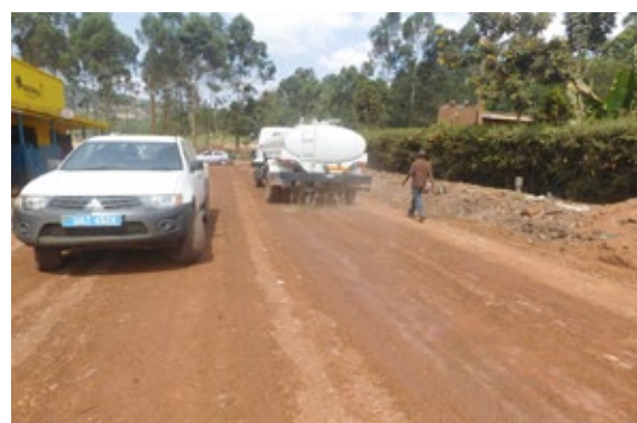
Laying of base layer on Kazoba Road (0.44km) as part of planned resealing under Q4 FY2017/18 programme. Implementation was delayed due to encroachment by residents.
