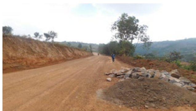
Rushoroza Rd (1.67km) received RMeM (widening, grading and gravelling) in Q4 FY2017/18. The road is one of the roads for tarmacking as part of the presidential pledges.
