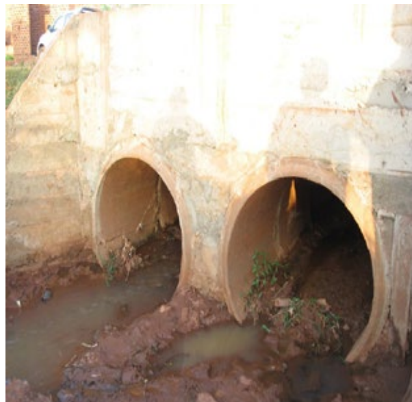
Makindye Ssabagabo MC: A double line of 1.2m diameter culverts installed at a swamp crossing on Municipal-Gang road
