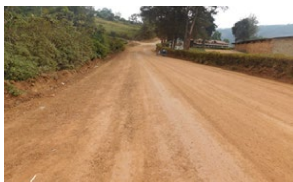
Rushoroza Rd (1.67km) received RMeM (widening, grading and gravelling) in Q4 FY2017/18. The road is one of the roads for tarmacking as part of the presidential pledges.
