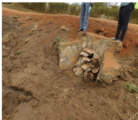
A section of the road received spot gravelling and culvert installation at CQ1-47+50. Community practices such as blocking culverts and offshoots remain a challenge.
