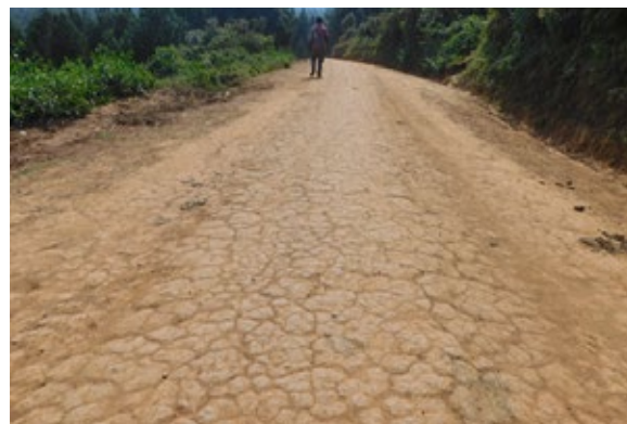
Kilwa-Hornby-Rugarama was graded but did not undergo gravelling due to breakdown of equipment.
