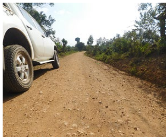
Bugarama – Rutooro – Burebane Rd (6.8Km) received grading and spot gravelling in Q3 FY2017/18. The road was in good motorable condition.
