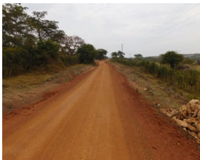
A section of the road received spot gravelling and culvert installation at CQ1-47+50. Community practices such as blocking culverts and offshoots remain a challenge.
