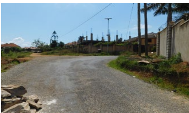
Kiwafu Road underwent surface dressing and installation of solar street lights under Periodic Maintenance. Drainage works were ongoing at the time of the site visit
