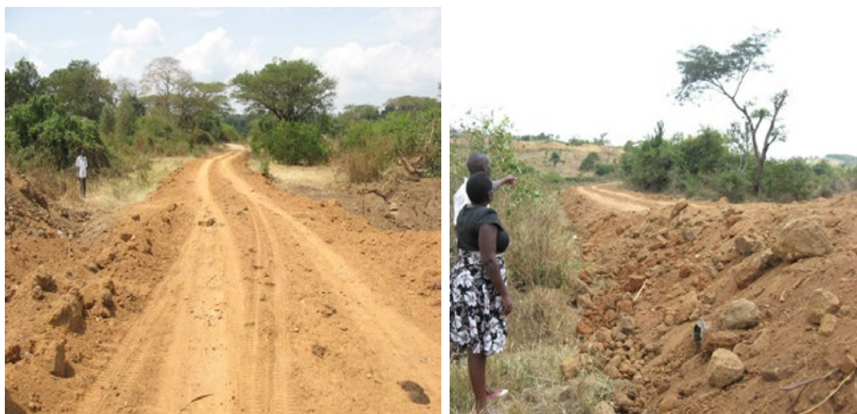
Mubende district: A section on Kanyegaramire-Lwengabi-Butengeza road (12km) that was undergoing embankment raising prior to spot regravelling under RMeM.
