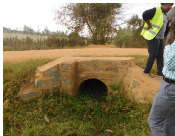
Inspecting a 900mm diameter concrete culvert installed at CH7+600, a low lying section.
