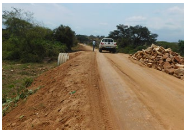
Installation of 200mm diameter culvert at CH2+700 station due to failure to procure the required cement in Q4 FY2017/18
