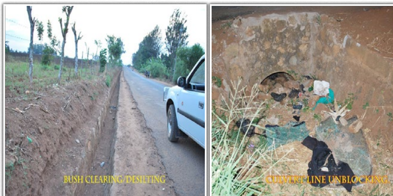
Mbale MC: Bush clearing and desilting of side drains Mbale MC: Culvert line unblocking
