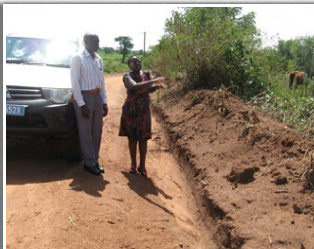
Kamuli district: A section on Nakibungulya-Bulopa road (7km) that received bush clearing and grading under periodic maintenance.
