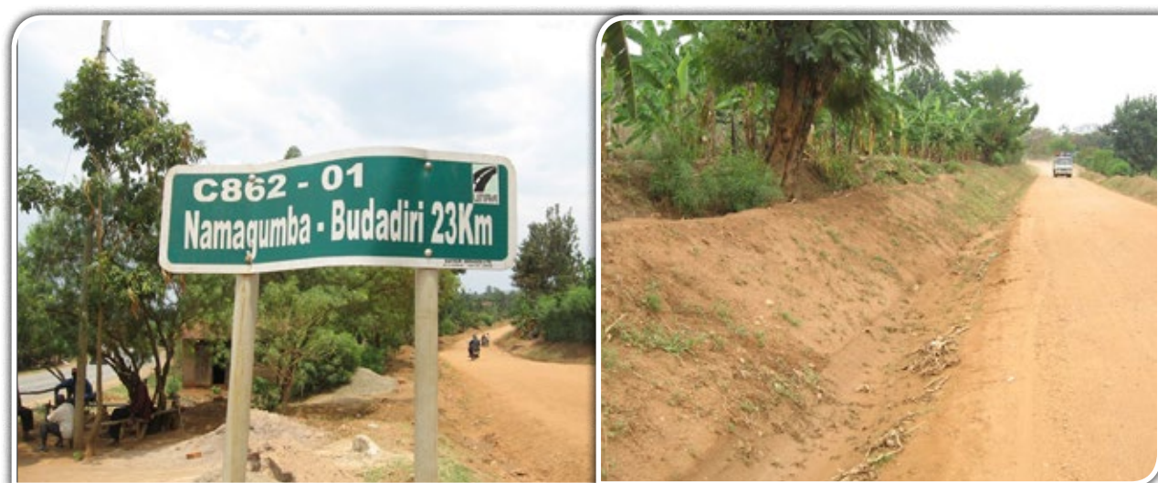
UNRA Mbale: Namagumba-Budadiri road (23km) fully graded and spot-regravelled under force account routine mechanised maintenance.
