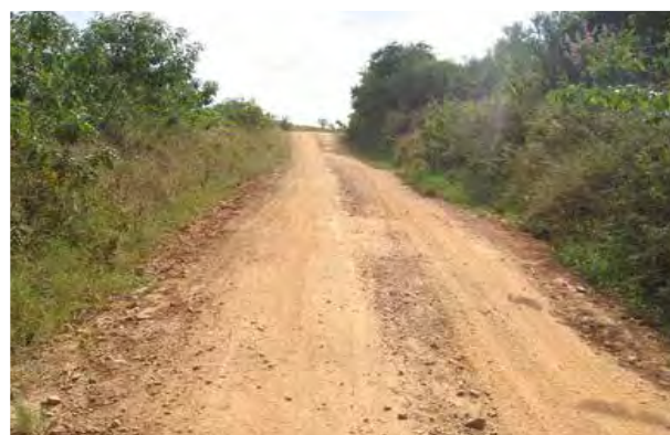
Rukungiri district: A section on Rukungiri-Rubabo-Nyarushanje road (27.8km) that was spot gravelled under RMeM.
