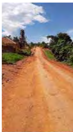
Kira MC: Sections of Kito - Nsasa road, which had been graded and spot graveled in selected sections
