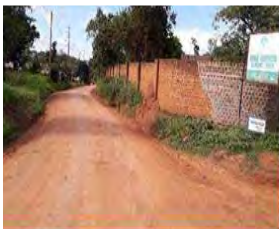
Kira MC: Sections of Kito - Nsasa road, which had been graded and spot graveled in selected sections
