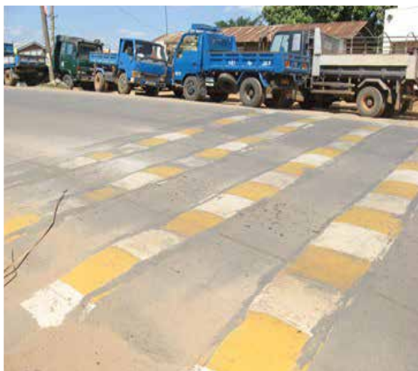
UNRA Mbarara: Newly repaired and painted rumble strips on Mbarara-Ntungamo road (60km) under routine mechanised maintenance
