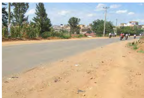
Mbarara MC: Ntare road (3.2km) that had received RMeM involving shoulder repair, pothole patching, and desilting culverts
