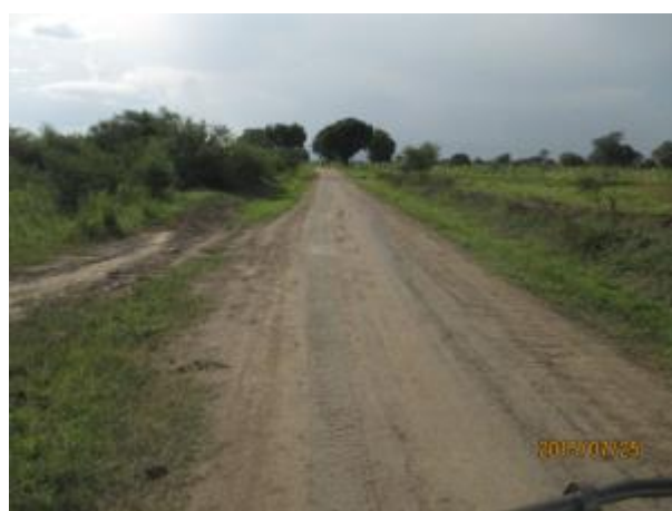
Moyo UNRA: Dzaipi-Tete-Nimule-Bibia, 35 km; Bad spots raised, but require gravelling.
