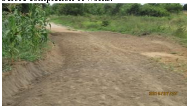
Moyo DLG: Achimali – Otubanga Landing site CAR, 3km, in Aliba Sub County; grubbing works by road gangs.
