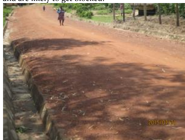
Arua MC: Dr. Charles Adriko road, 700 m; Well gravelled road and with lined side drains.
