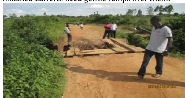
Arua DLG: Ajono – Andelizo road, 8.5 km; Broken timber deck bridge.
