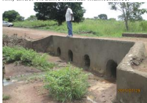
Yumbe DLG: Improved Ijosi swamp crossing in Kuru sub county.
