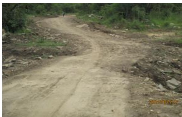
Moyo DLG: Lama – Gbalala road, 4.6 km; Culverts need extension before gravelling works.
