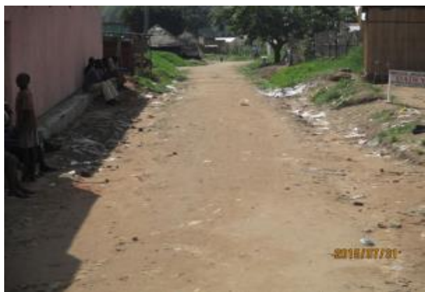
Arua MC: Jubale lane, 200 m; Graded but not compacted, narrow because of road reserve encroachment
