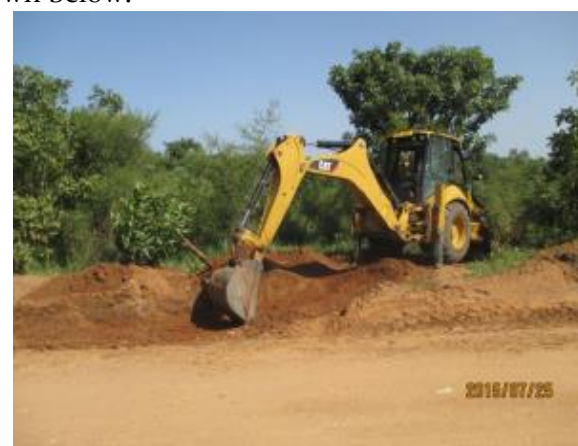
Moyo UNRA: Moyo – Yumbe, 69 km; Term maintenance contractor excavating off shoots.
