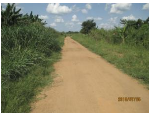
Moyo UNRA: Adjumani-Sinyanya, 35 km: RMM should be intensified and many sections require gravelling.
