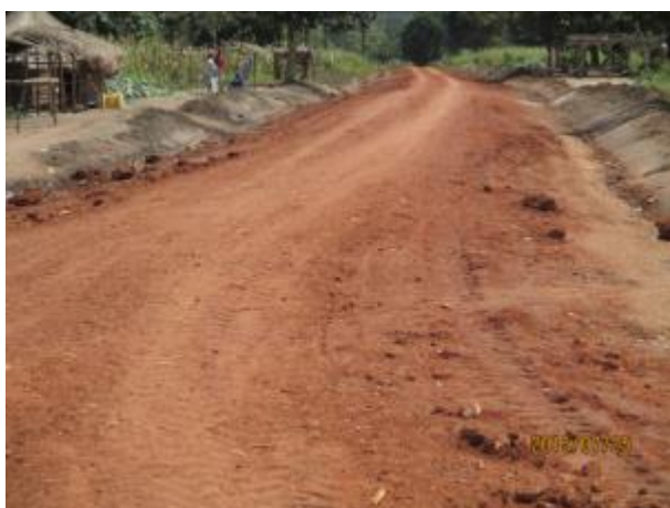
Moyo UNRA: Sper – Kei, 12 km: Gravel need compaction.
