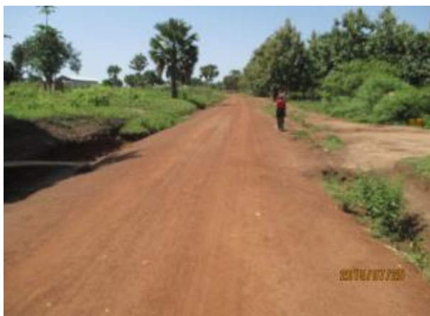
Moyo UNRA: Kerila – Midigo – Kerwa – Kenda, 43 km: Road well shaped under force account, but drains need scour checks to control erosion.
