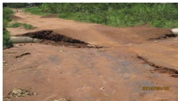
Arua DLG: Odupi - Invepi - Lugbari road, 20 km; Installed culverts need gentle ramps over them.
