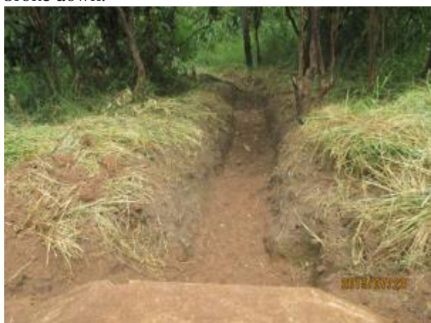
Amuru DLG: Otwee - Mutema - Okungedi road, 16.3 km; well executed culvert channel cleaning.
