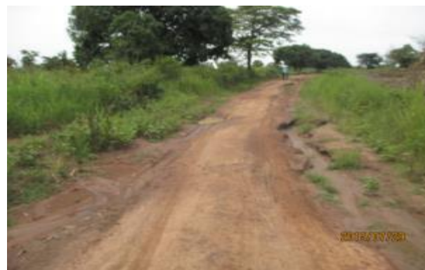
Yumbe DLG: Kuru – Lobe road shall require periodic maintenance after missing out on routine mechanised maintenance because of the drift collapse.
