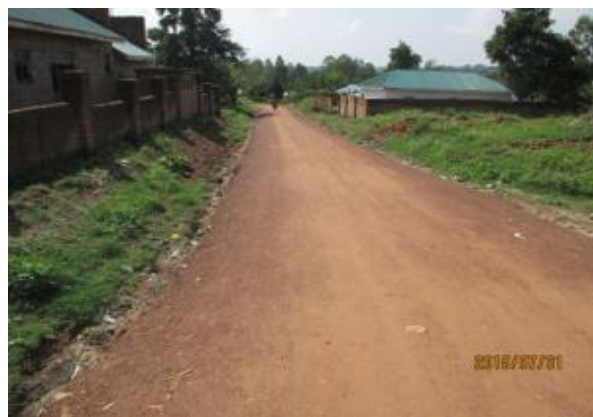
Arua MC: Abraham – Riji, 400 m; Gravelled road, require drainage interconnectivity.
