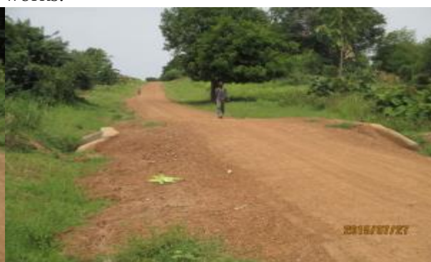
Moyo DLG: Obongi – Itipa road, 9 km; well installed culverts.
