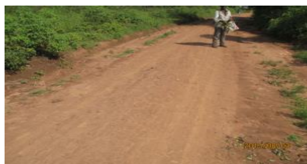
Arua DLG: Aripezu – Andelizo CAR, 2 km in Adumi sub county; Road worked on by road gang opening drains by grubbing
