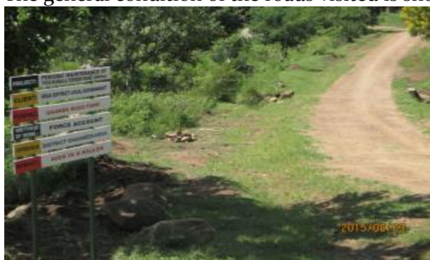
Arua DLG: Yivu – Kubala road, 4.0 km; Well graded road though not compacted but awaiting spot gravelling
