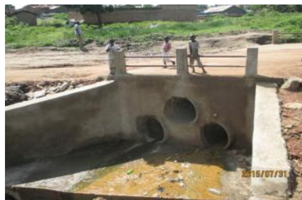
Arua MC: School road, 1.2 km; seem inadequate and are likely to get blocked.
