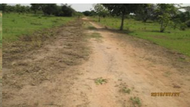
Moyo DLG: Dongo – Morobi CAR, 12 km in Itula sub county; grubbing works by road gangs.
