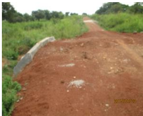
Amuru DLG: Amuru TC roads; culverts installed and approaches being improved.
