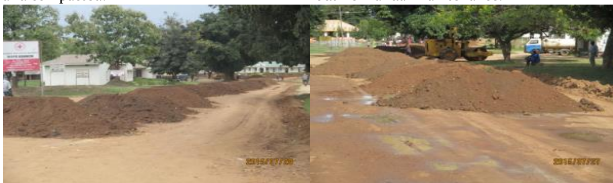
Moyo DLG: Moyo TC roads; Laying base course material for road to be tarmacked.
