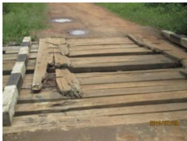
Yumbe DLG: Oya timber bridge on Tala – Lodonga road requiring urgent repairs.
