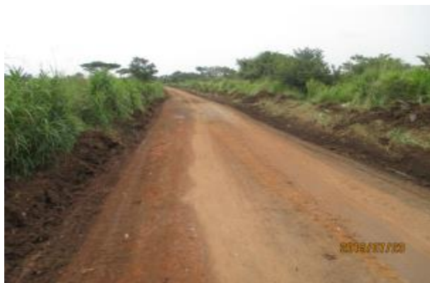
Amuru DLG: Otwee - Mutema - Okungedi road, 16.3 km; grading works but without roller.
