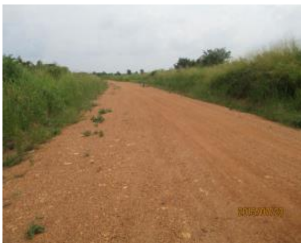
Amuru DLG: Amuru TC roads; well graded, gravelled and compacted.
