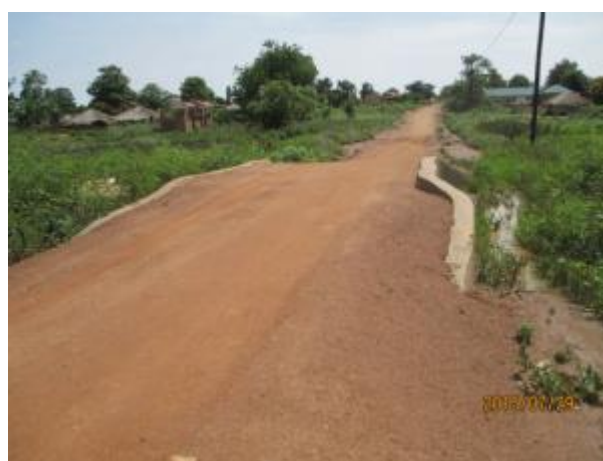
Yumbe DLG: Yumbe TC roads graded, spot gravelled and drainage improved.
