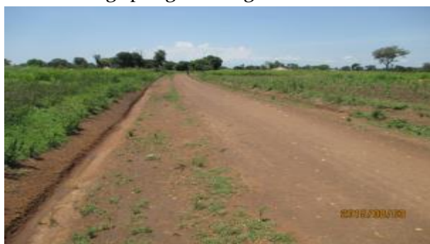
Arua DLG: Odupi - Invepi - Lugbari road, 20 km; Graded road but no compaction.
