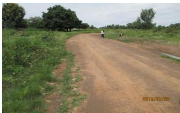
Yumbe DLG: Lodonga – Adibo road, 7.8, graded but not compacted.
