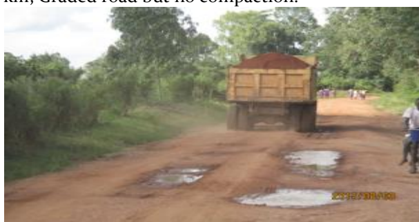
Arua DLG: Ajono – Andelizo road, 8.5 km; Road worked on but grossly damaged by M/s CICO trucks
