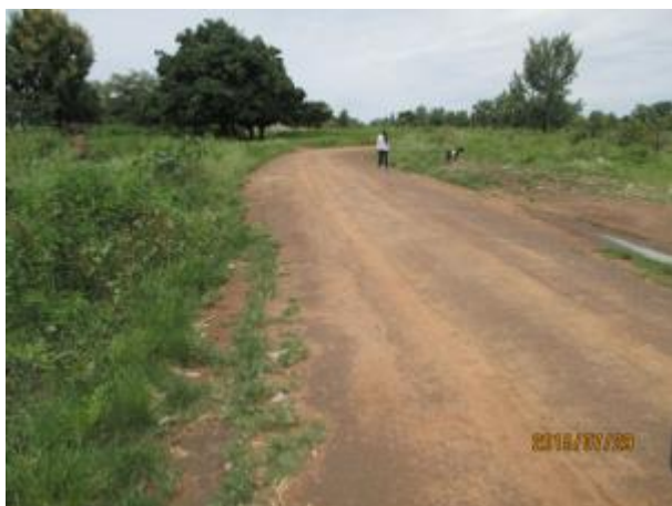
Yumbe DLG: Driambu – Orichaku CAR, 7 km in Kei sub count, that was graded but not compacted.
