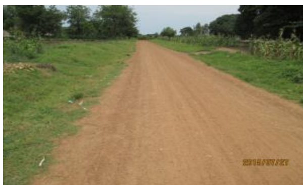
Moyo DLG: Obongi – Itipa road, 9 km; well graded, gravelled and compacted road.
