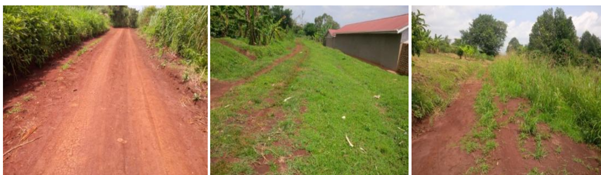
Katooke TC: Sections of Nyakana – Kaheru road, which was planned for periodic maintenance but was only opened and graded without compaction.
