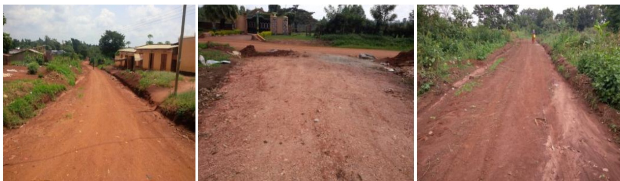
Katooke TC: A section of Irumba – Banura road (L); and Sections of Market Street (C) & (R) which were only graded without compaction.
