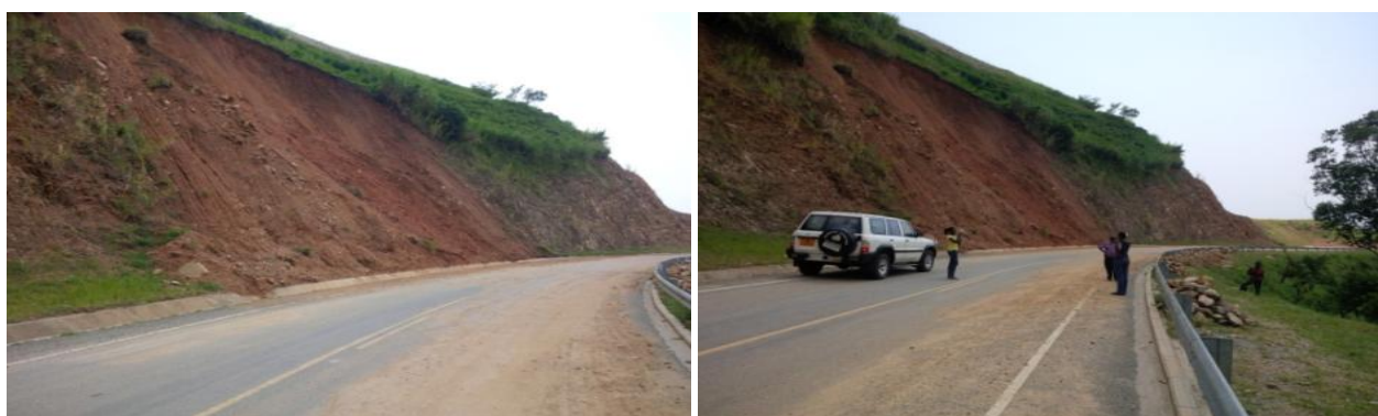
UNRA Fort Portal: Sections of Fort Portal - Bundibugyo road, which experienced landslides that were removed using a mix of contracting and force account
