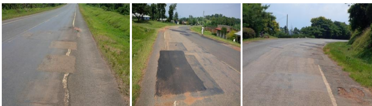
UNRA Fort Portal: Sections of Fort Portal – Rwimi road, which was patched using force account.
