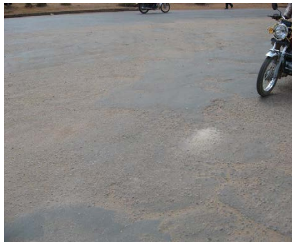
Masaka MC: A section on Elgin Street road (0.7km) that had received pothole patching under routine mechanized maintenance
