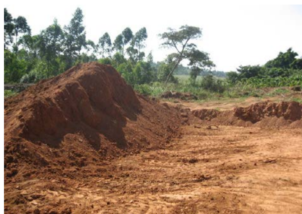
Kalungu District: A gravel borrow pit for swamp filling of an 800m section on Kaliro-Nabutangwa-Bwasandeku road (11.4km)
