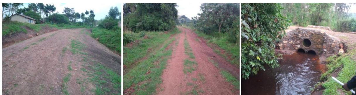
Kyenjojo DLG: Sections of Kaiganga – Nyakisi road, which received routine mechanized maintenance, not the planned periodic maintenance
