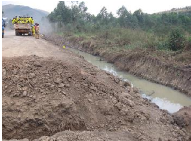
UNRA Masaka: Raising of 2km of low lying areas on Lyantonde-Ntuusi road (58km) under routine mechanized maintenance using term contracts
