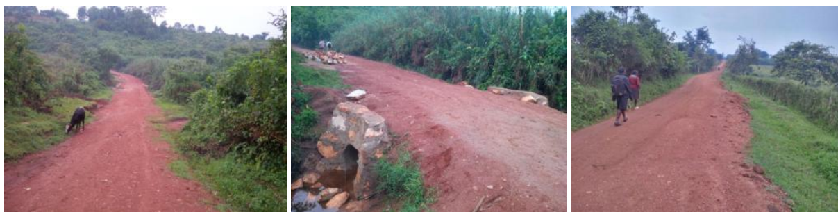
KyenjojoTC: Works on Kijumaji Swamp where raising and culverts installation was done (L) & (C); and partially spread gravel on Kikwete road.
