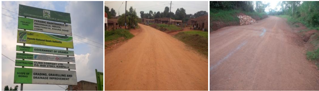
UNRA Fort Portal: Sections of Rwamwanja - Kihura road which received periodic maintenance. (R) is a typical example of the sunken backfill on several of the culverts. The road was under defects liability period.
