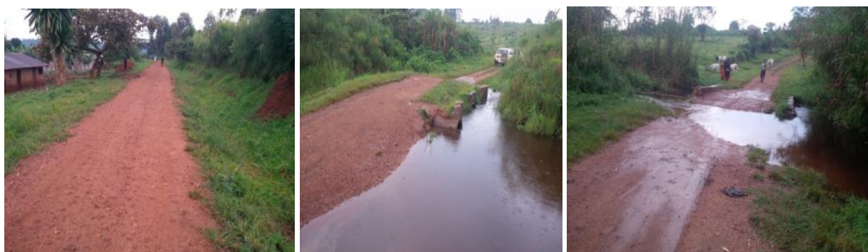
Kyenjojo DLG: Sections of Nyakisi – Rubayo – Haikona road (10.5Km), which received routine mechanized maintenance. Bottlenecks in swamps at Km6.6 (C) and Km7.6 (R) where water was passing across the road surface.
