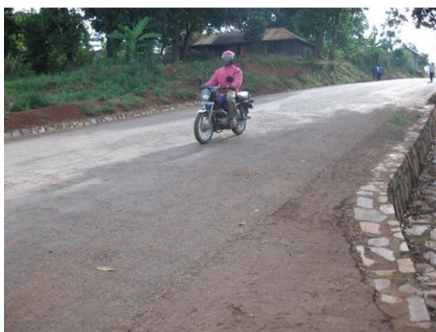
Entebbe MC: A 1km section on Sewabuga road (2km) that had been resealed (single surface dressing) under periodic maintenance
