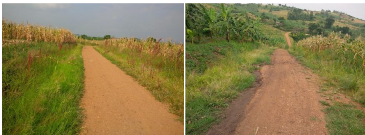
Rwimi TC: Sections of Kyeibumba – Nyabwina road which received periodic maintenance but was deteriorating fast due to poor routine maintenance
