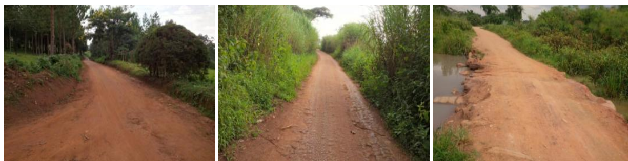
Kyegegwa DLG: Sections of Wekomire – Bulingo – Bukere road, which received routine mechanized maintenance
