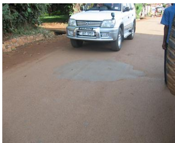
Entebbe MC: Kitoro road (1km) that had received pothole patching under routine mechanized maintenance
