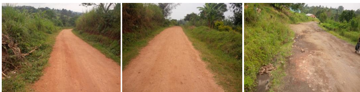
Kabarole DLG: Graded Sections of Kichwamba – Kiburara road (L) and (C); and A section of Nyabukara – Harugongo road (R) which had developed a deep galley across the road
