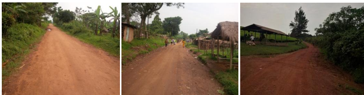
Kabarole DLG: Graded sections of Kahangi - Mbagani road (L); and Graded Sections of Kiburara – Orubanza road (C) and (R)
