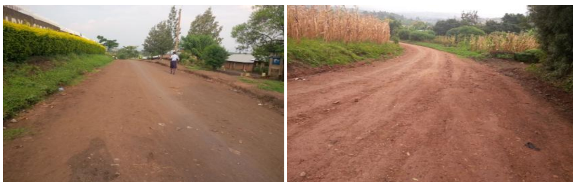
Rwimi TC: Sections of the graded and spot gravelled Excel – Kitebe road.
