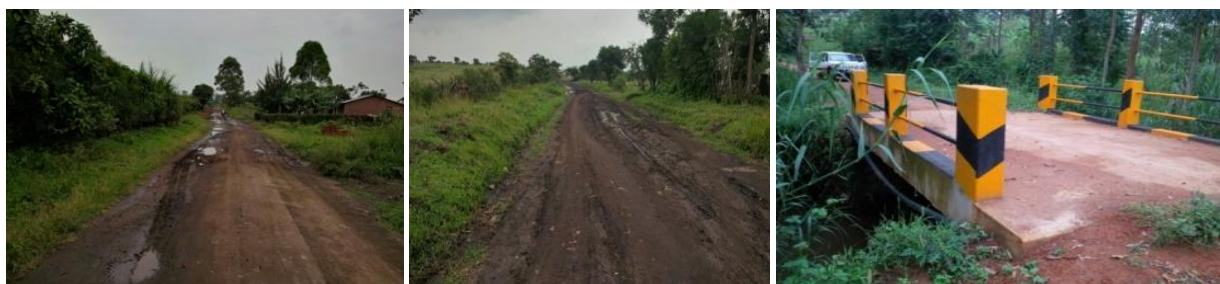
Kabarole DLG: Graded sections of Nyabukara – Harugongo road which had been damaged by rain due to poor drainage along the road (L) and (C); and (R) newly constructed bridge decking and guardrails on Wakaberege Bridge.
