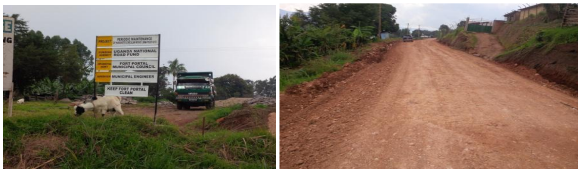
Fort Portal MC: A Section of Harukoto Circular Road, where regravelling was in progress
