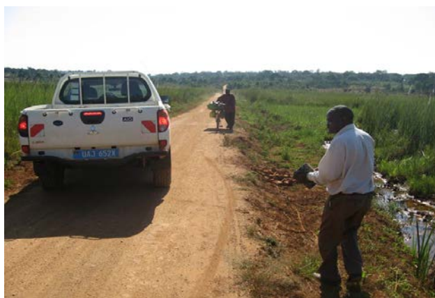
Kalungu District: Kaliro-Nabutangwa-Bwasandeku road (11.4km) that underwent Swamp filling on an 800m section under routine mechanized maintenance
