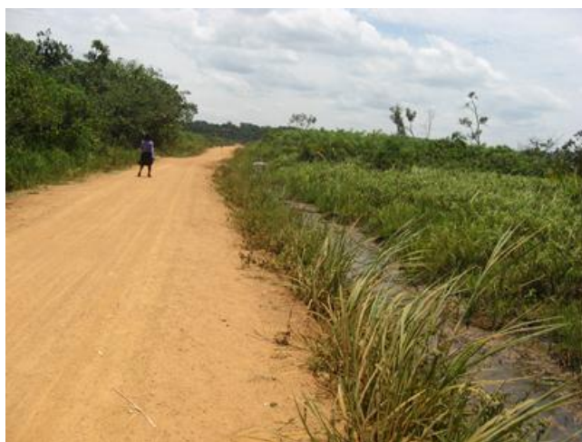
Mpigi District: A 1km swamp section on Mbizzinya-Kumbya-Jajamba road (7km) that had been filled as an emergency
