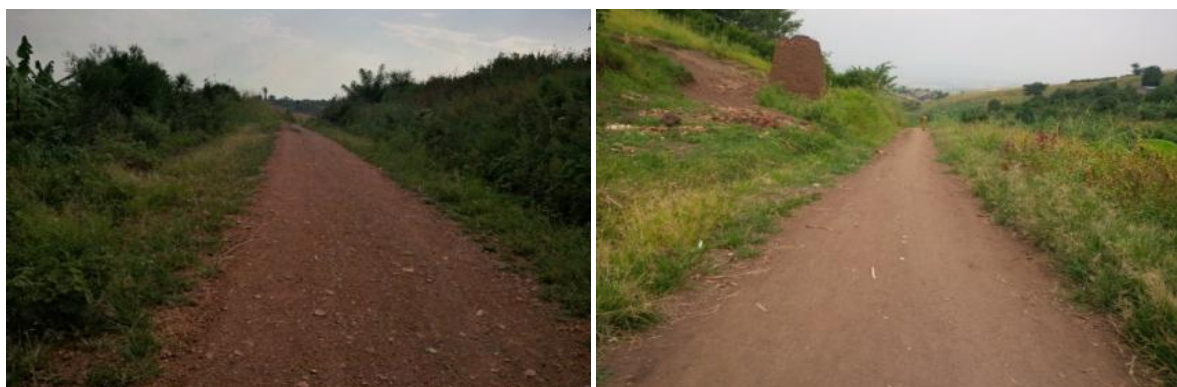
Rwimi TC: Sections of Gatyanga II road which received grading and spot gravelling. The shoulders had overgrown grass.
