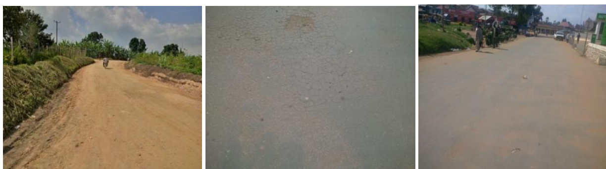
Fort Portal MC: A Section of Nyabukara - Harugongo road: (L) Surface failures on newly surfaced Winyi – Kasaijja road (C) and (R)
