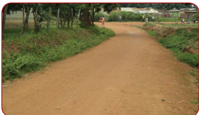
Arua MC: Marijan road, 1.5Km; Road well graded and drains desilted.
