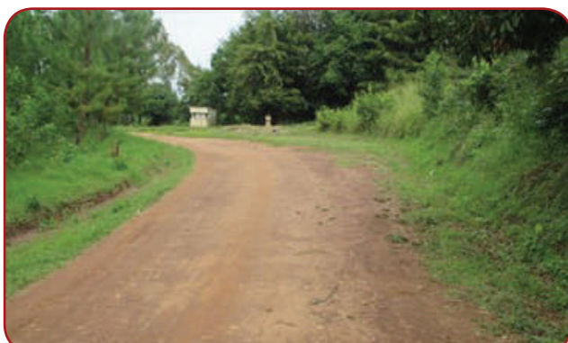
Zombo DLG: Warr – Alanyi road, 11Km; Road graded but with almost flat camber.
