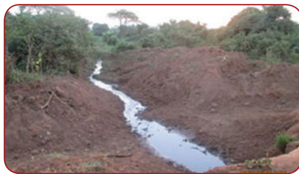
Lira UNRA: Ngetta – Kitgum Bdr, 21 Km; Opened culvert outflow channels by Force Account.
