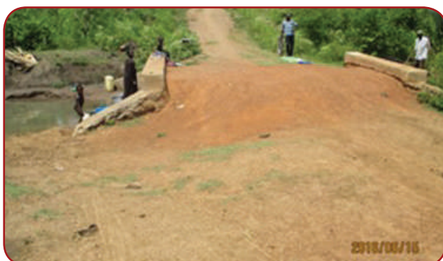
Koboko DLG: Nyai – Lodonga road, 8 Km; Culvert need smoothed approaches.
