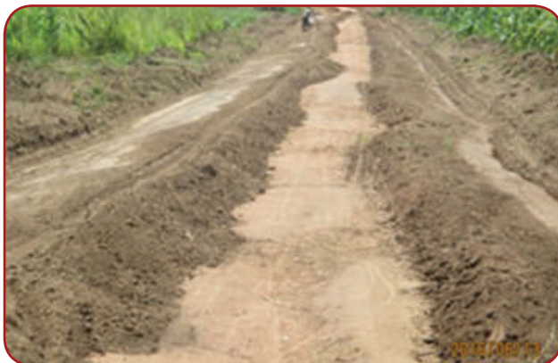
Adjumani DLG: Openzinzi – Obilokongo road, 9 Km; Ongoing grading works but without a water bowser.
