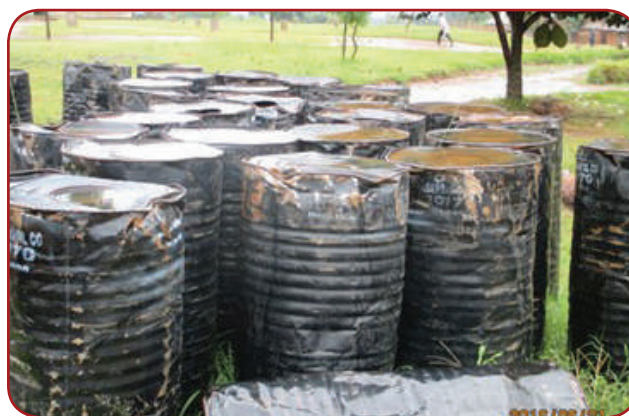
Paidha TC: Olarker road, 2.4 Km; 30 drums of bitumen in preparation for tarmacking works.
