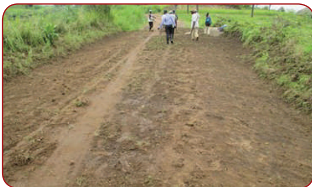
Zombo DLG: Zombo – Atyak – Warr road, 10.3Km; Grubbing works by road gang.
