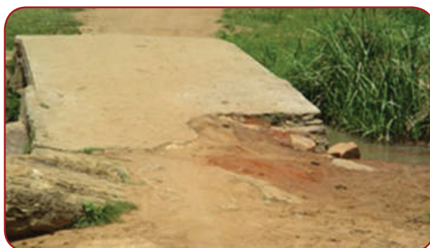
Maracha DLG: Oniba - Lurua, 5.4 Km; The ford should be repaired by carrying out river training, placement of safety pillars/barriers and repairs of approaches.
