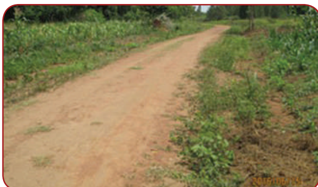
Koboko DLG: Uganda Congo Bdr road, 14 Km; Road surface good but getting overgrown especially in the drainage.
