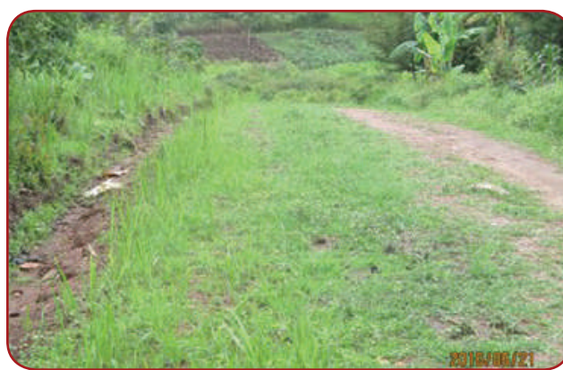
Zombo TC: New town roads opened but not compacted and require good drainage.
