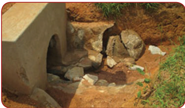
Maracha DLG: Etoko – DRC Border road, 5.2 Km; Failing culvert end structures that should urgently be repaired.
