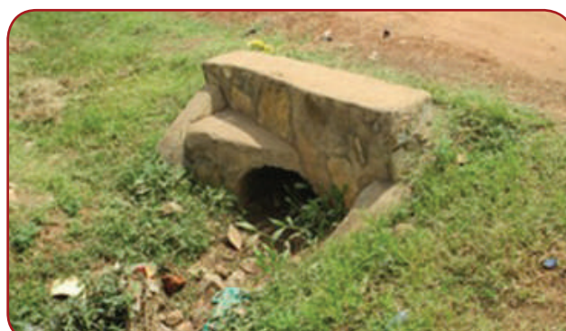
Koboko DLG: Keri – Nyai road, 16.7 Km; Road drainage need cleaning.
