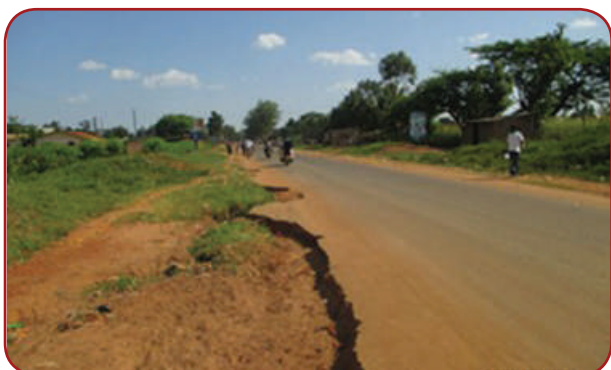
Lira UNRA: Lira – Ngetta 8km; Broken road edges due to absence of side drain.
