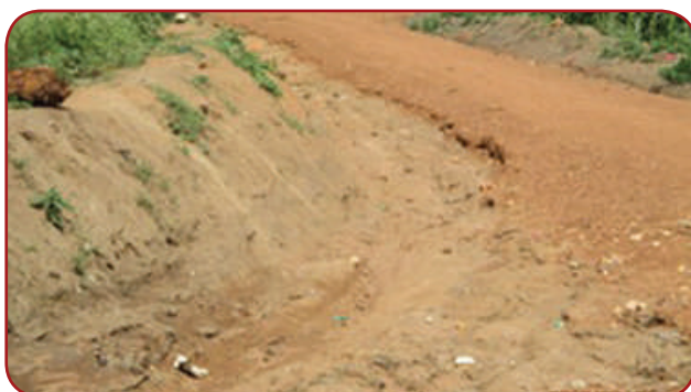
Koboko Town Council: Cross culverts need to be installed as to control flooding and erosion
