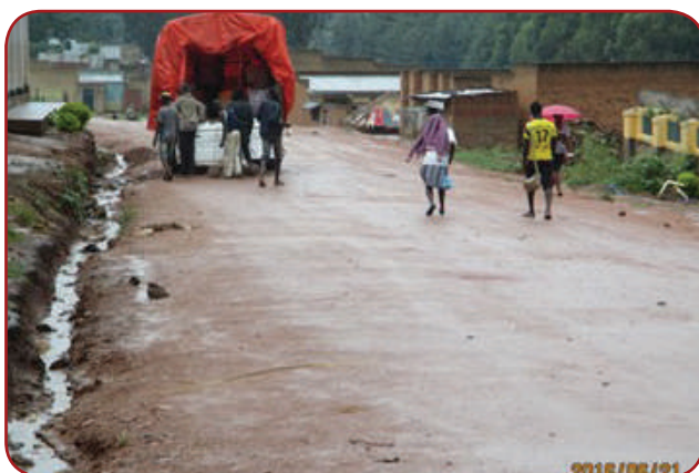
Paidha TC: Olarker road, 2.4 Km; Lime stabilized base of road undergoing upgrading.
