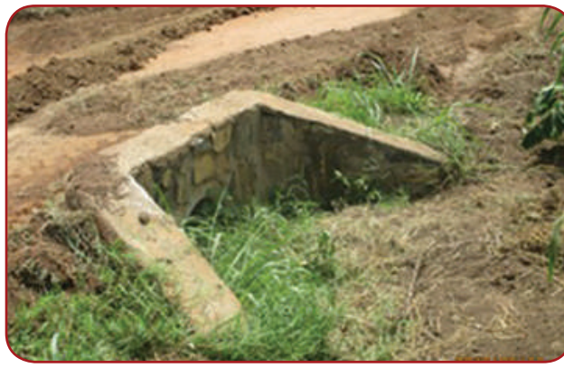
Adjumani DLG: Openzinzi – Obilokongo road, 9 Km; Drainage maintenance including cleaning of culverts required.
