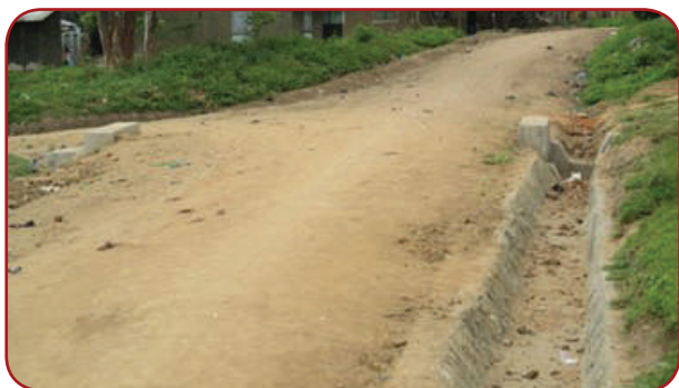
Arua MC: Dr. Eric Adriko road, 0.5Km; Road graded and drains lined awaiting gravelling
