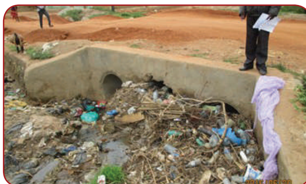
Arua MC: Adrua road, 1.5Km; Garbage management required as to keep drains functioning well.
