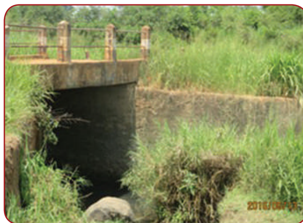
Adjumani DLG: Openzinzi – Obilokongo road, 9 Km; Maintenance works needed at the bridge and include; placement of warning signs, river training and painting.
