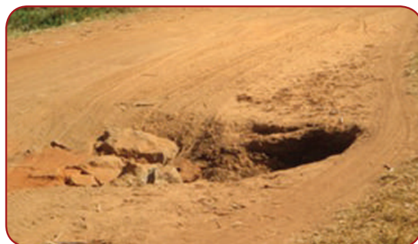
Lira UNRA: Apala – Adwari, 27 Km; Broken culvert that would have been replaced if maintenance intervention had been carried out at programmed time.
