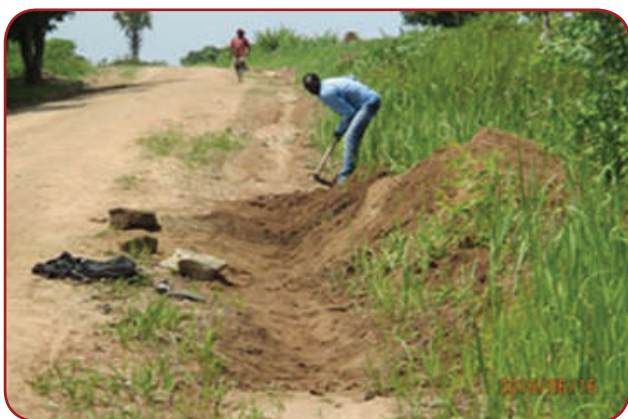
Maracha DLG: Gbulua - Anyambia road, 12.6 Km; Desilting of road side drain.
