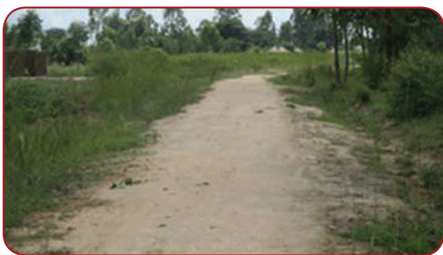
Maracha DLG: Oniba - Lurua, 5.4 Km; Road graded though not compacted, requiring opening of offshoots.
