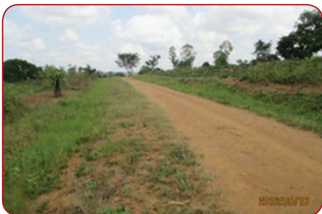
Maracha DLG: Odrua – Midiowa – Abara CAR, 5 Km; Grass cut, pothole filled by road gangs.
