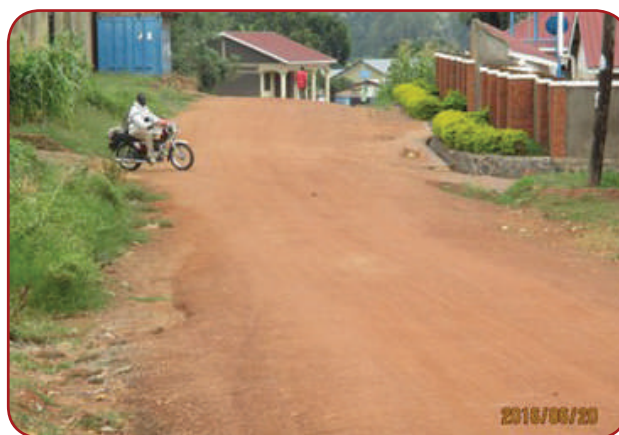
Arua MC: Awindri Crescent, 1Km; Silted drain causing wash away of gravel.
