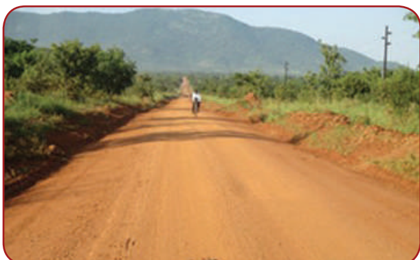
Lira UNRA: Adwari – Olilim, 45 Km; Grading and spot gravelling carried out by Force Account.
