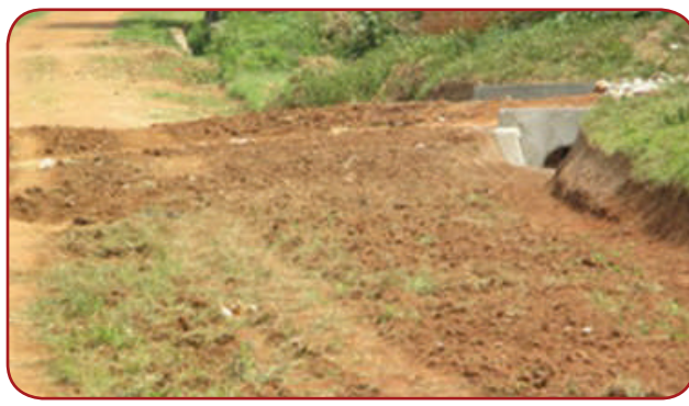
Maracha Town Council: Oluma road, 2Km; Grubbing and drainage opening by road gang.
