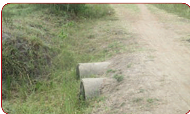
Adjumani DLG: Kuleku – Amelo road, 5 Km; Culverts in need of adequate cover and building of end structures.
