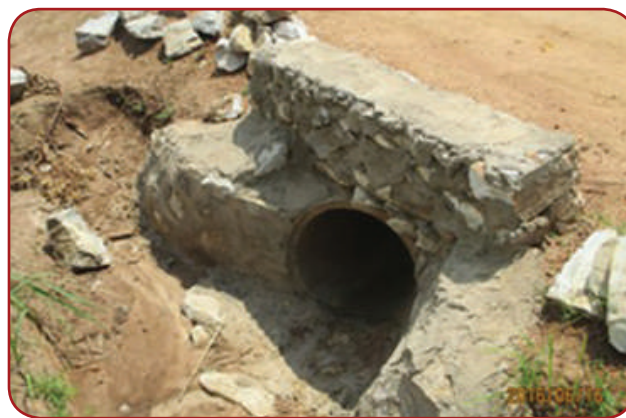
Maracha DLG: Gbulua - Anyambia road, 12.6 Km; Building of culvert end structures.
