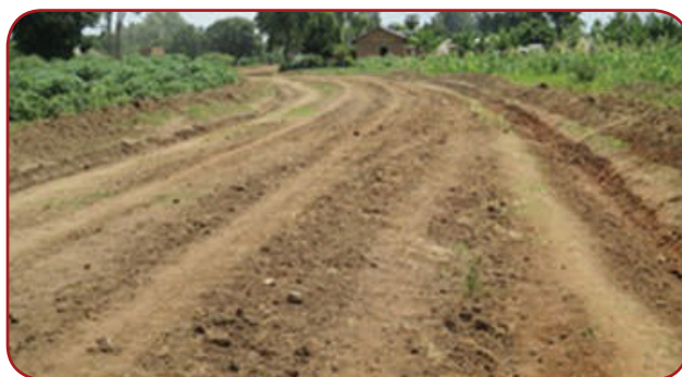
Maracha DLG: Arimbe, 1.3 Km; Road graded but not well shaped to camber and no compaction.
