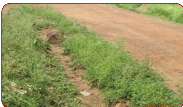
Koboko DLG: Keri – Nyai road, 16.7 Km; Road getting bushy due to absence of road gangs though road surface good.
