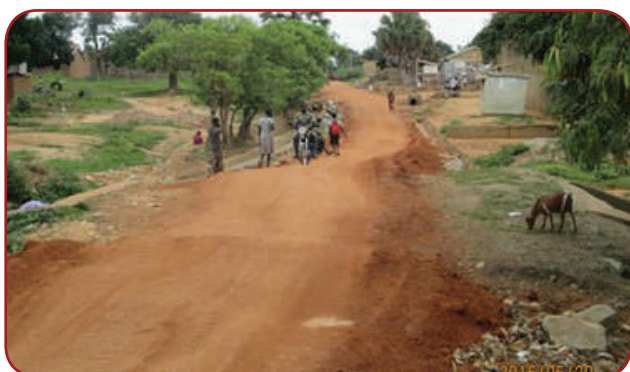
Arua MC: Adrua road, 1.5Km; Back filling works at the installed culvert crossing
