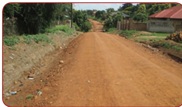
Koboko Town Council: 150 mm layer of gravel placed under periodic maintenance.
