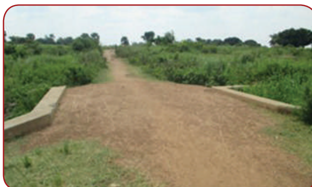
Adjumani DLG: Kuleku – Amelo road, 5 Km; Safety barriers which were vandalized need replacement.
