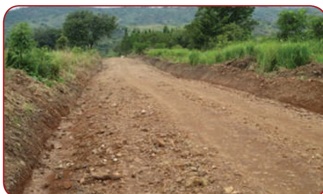
Zombo DLG: Nyandima – Atyak road, 11.5Km; Road graded but not compacted neither offshoots opened.
