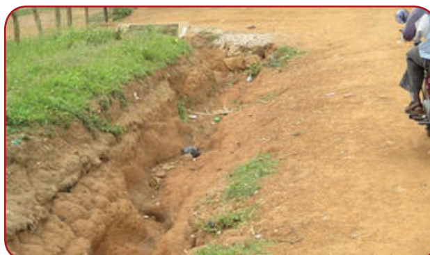
Arua MC: Marijan road, 1.5Km and Josephine Kagwa road, 0.2Km; Drains need lining because of huge volume of storm water from town.
