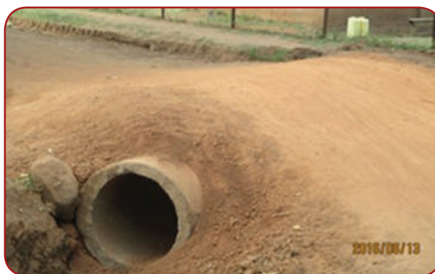
Adjumani Town Council: Installed culverts require smooth ramps over them as well as building end structures.
