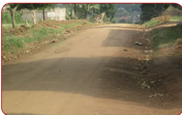
Adjumani Town Council: Well graded roads though not sufficiently compacted.
