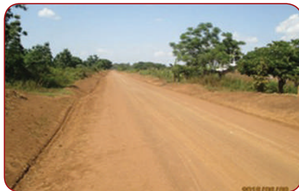
Lira UNRA: Dokolo – Namasale, 88 Km; Spot grading works under term maintenance.
