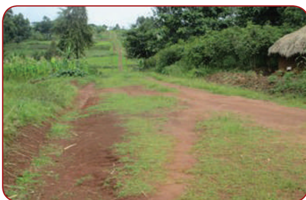
Zombo TC: New town roads opened but not compacted; they also require good drainage.
