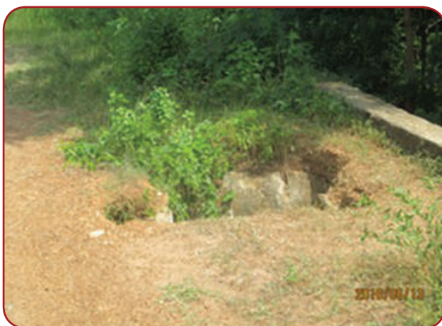
Adjumani DLG: Magburu – Loa CAR (3 Km; Culvert need repair, otherwise road can easily get cut off.
