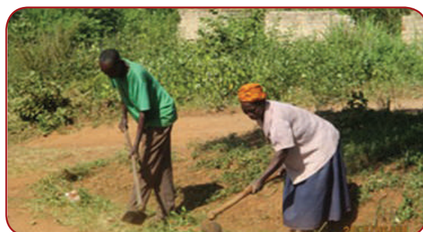
Lira UNRA: Alooi – Dokolo, 42.6 Km; Labour Based Contractors cleaning side drain.
