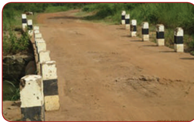
Adjumani DLG: Dzaipi – Magara road, 7 Km; Drift deck at Ch. 3.2 Km need to be repaired given that reinforcement is getting exposed.
