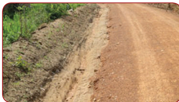
Koboko Town Council: Steep road sections should have the side drain lined.
