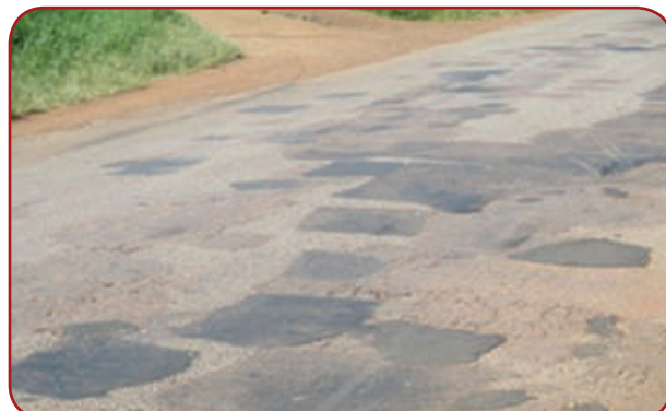
Lira UNRA: Lira – Kamdini, 70 Km; Road in need of major rehabilitation works in the wake of such sections which have been over-patched.
