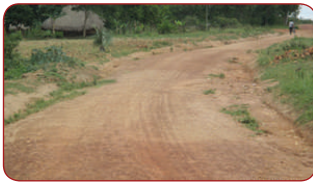
Maracha DLG: Etoko – DRC Border road, 5.2 Km; Graded road but requiring opening of offshoots as to avoid surface runoff and silting of side drains.
