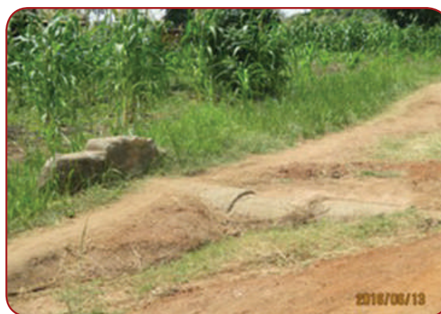
Adjumani DLG: Ciforo – Magburu road, 5 Km; Road grossly eroded, culverts broken and silted.
