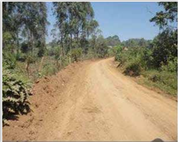
Masaka DLG: Sharp corners on the graded and shaped sections of Bulayi- Kigaato- Kiyimba road (5km) lacking road safety signposts.
