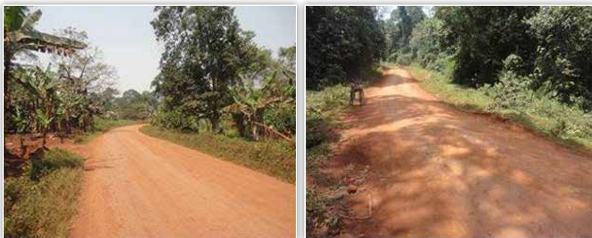
Buikwe DLG: Sharp corners on the graded and shaped sections of Kawomya- Senyi road (9.8km) lacking road safety signposts completed in Q1- 15/16.
