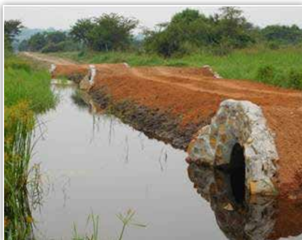
Lwengo district: Culvert crossings on swampy section of Bunyere-Kiryangoma-Nkunyu Rd.
