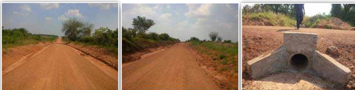
UNRA Arua: Sections of Wandī – Rhino Camp road which received full regravelling using term maintenance contracts.
