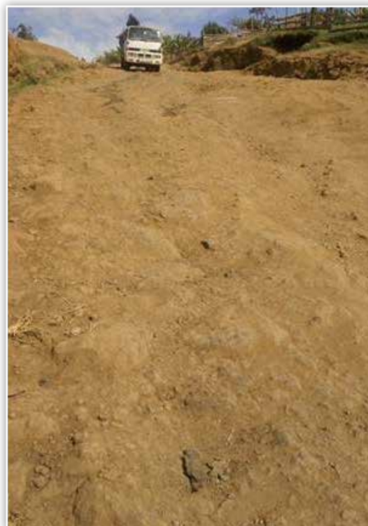
Mbale UNRA: Inspection of rock outcrop sections along Kapchorwa – Suam Road which render it impassable despite the fact that the rest of the road link is in a very good condition.
