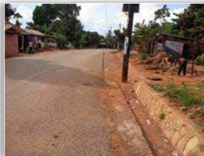
Entebbe MC: Sections of Sewabuga road, which received resealing and lining of side drains. Surface failures were seen (L) and (C) at start of the road.
