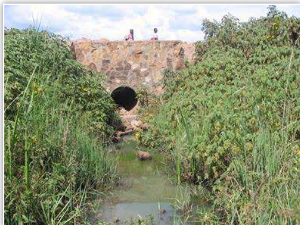
UNRA Tororo: A headwall constructed to retain the backfill at a culvert crossing on Tororo-Nagongera road (19.6km) under routine mechanized maintenance using term contracts
