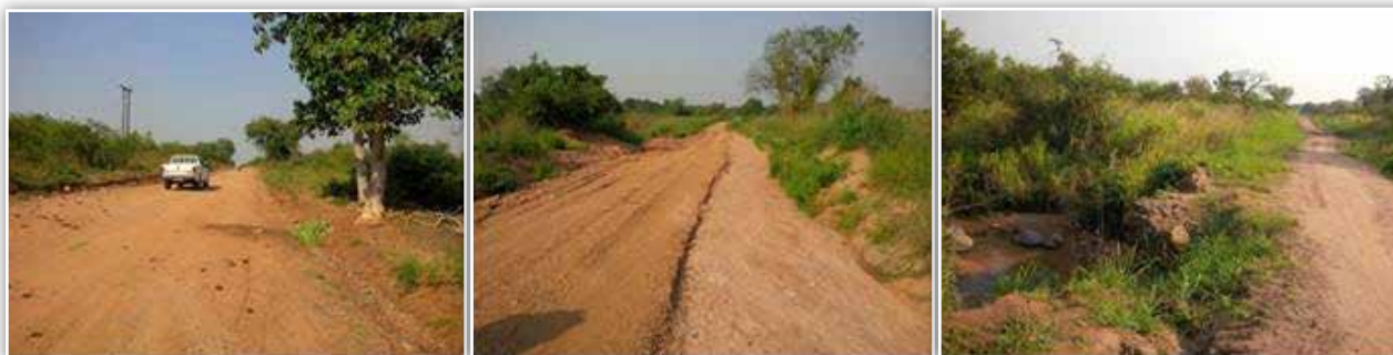
UNRA Arua: Sections of Okollo – Inde road, which was worked on using force account. (C) A typical silted side drain along the road. (R) A typical collapsed Headwall.
