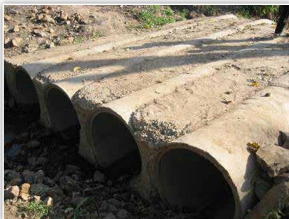
Tororo MC: Installation of a 4-line stream culvert crossing on Civic road (1.1km) that was being widened.
