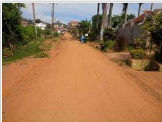
Entebbe MC: Sections of Kiwafu Close, which received routine mechanised maintenance – essentially grading.
