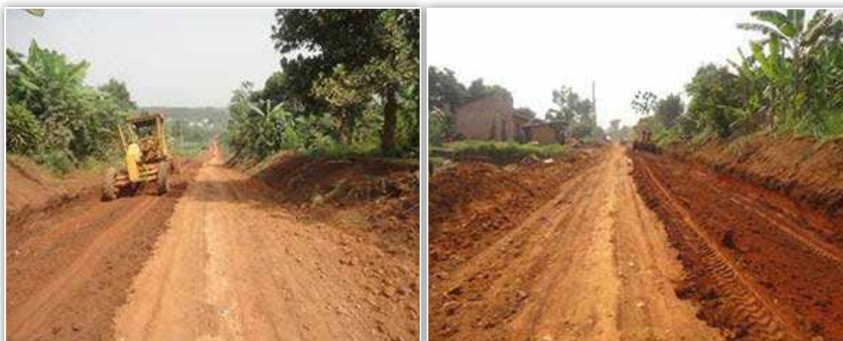
Mukono DLG: Routine mechanised maintenance works in progress on Kigombya- Seeta- Sezibwa road (14 km)
