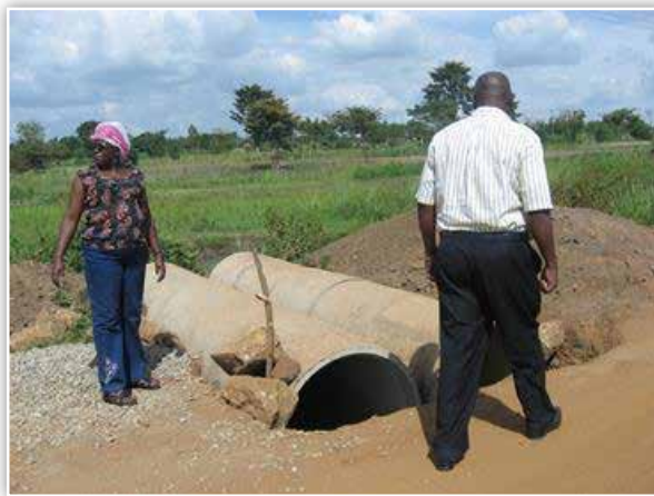
UNRA Tororo: Culvert installation at a swamp crossing on Tororo-Nagongera road (19.6km) under routine mechanized maintenance using term contracts
