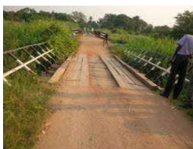
UNRA Arua: A Section of Manibe - Wandu road (L) and Ora Bridges I & II where the timber decks had been replaced in Q1 FY 2015/16
