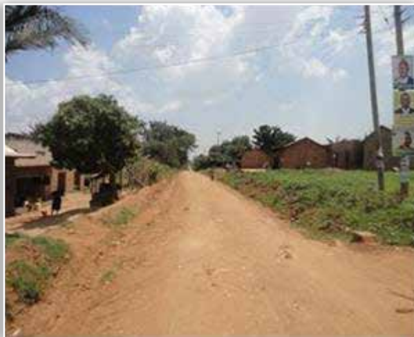
Masaka DLG: Graded and shaped sections on Kyanamukaaka– Buyaga road (11km) completed in Q2- 2015/16.
