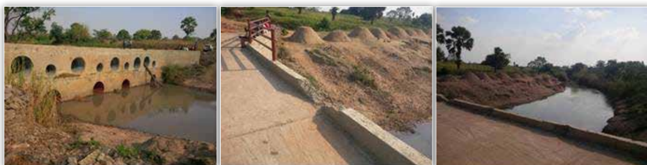
Yumbe DLG: Sections of Kochi Vented Drift Bridge showing the works that had been done before being destroyed by flash floods.
