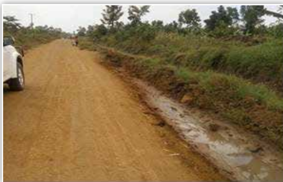
Mbale UNRA: Sections along Budadiri – Nalugugu Road with no offshoots leading to rainwater ponding on the road. The team leader discussing with the UNRA Station Manager on proposed remedies.
