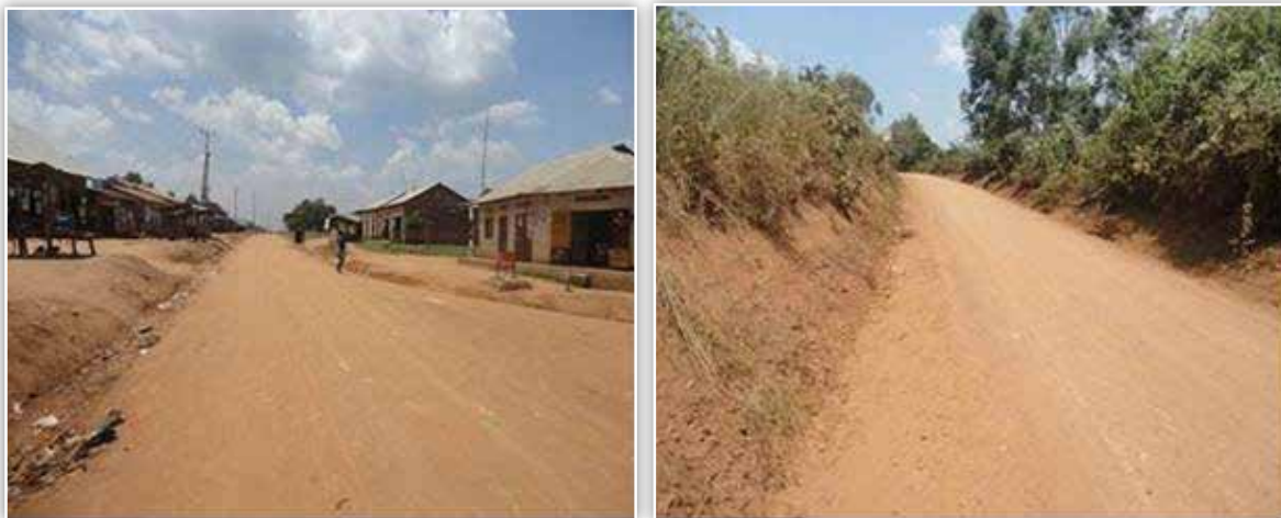
Masaka DLG: Graded sections on Kyanamukaaka- Bukunda road (8km) completed in Q2- FY 2015/16.
