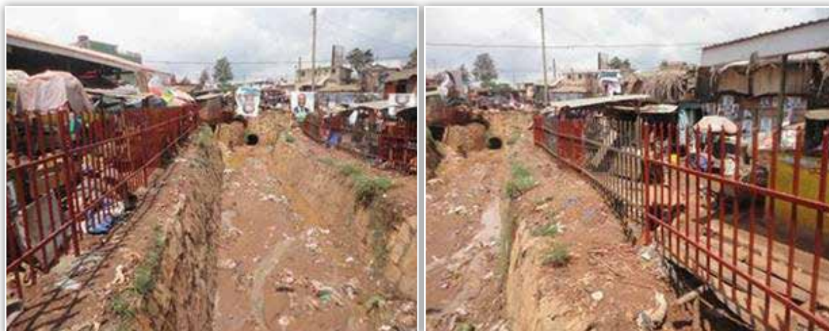
Mukono MC: Stone pitching and guard rails installed on Kame valley road drainage channels
