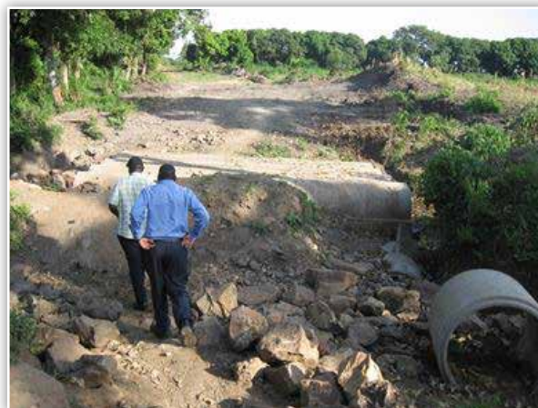
Tororo MC: Culvert installation works on Civic road (1.1km) that was being widened.
