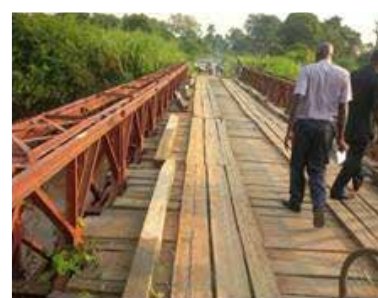
UNRA Arua: A Section of Manibe - Wandu road (L) and Ora Bridges I & II where the timber decks had been replaced in Q1 FY 2015/16
