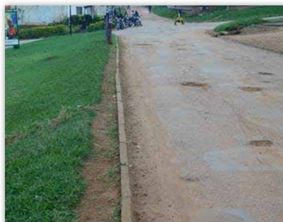
Masaka MC: Grass clearing and grubbing on Hobbart street under Routine Manual Maintenance.
