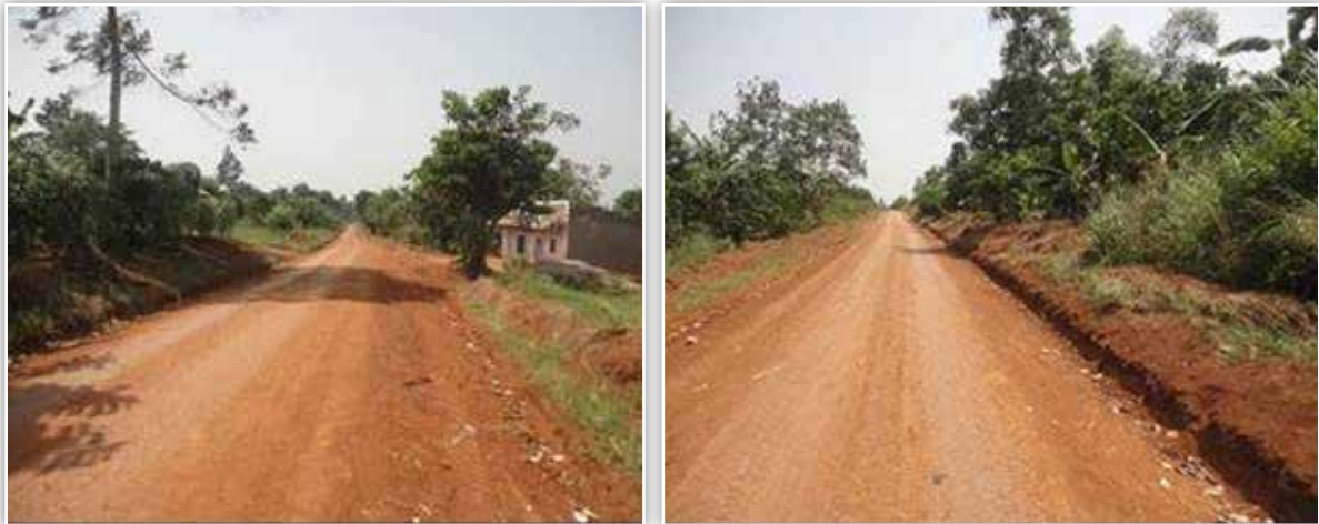
Buikwe DLG: Graded and shaped sections on Lweru – Makindu road (7 km) road completed in Q2- 2015/16.
