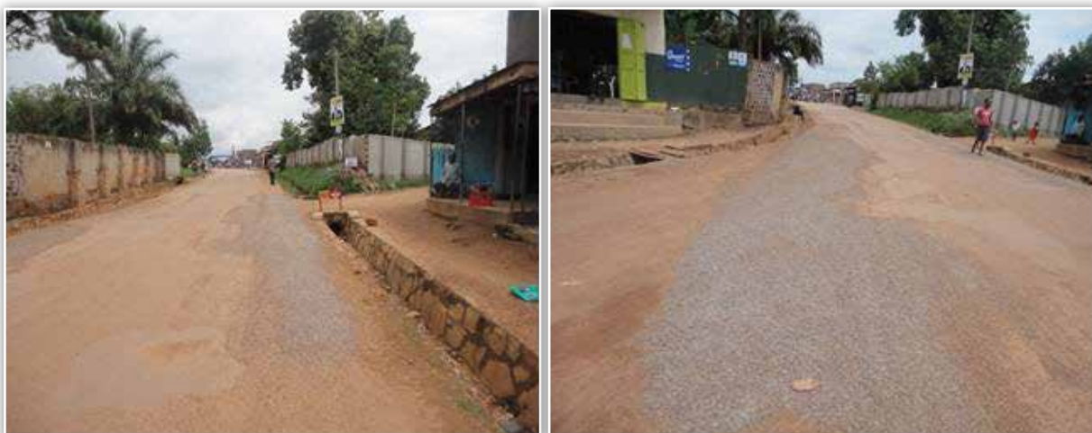
Mukono MC: Pothole patching on paved sections of Ntaawo- Nakabago road (5.3 km) with loose stone chippings.
