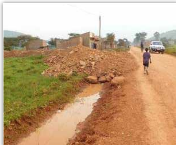
Lwengo district: Building materials dumped in side drain along Bijjaba Road which was undergoing routine mechanised maintenance.
