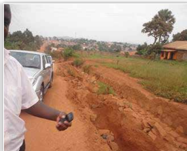
UNRA Kampala: Sections of Kabusu – Wankulukuku- Kitebi- Bunamwaya- Kajjansi (6.1Km) requiring erosion protection measure in the side drains.
