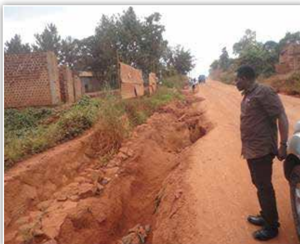
UNRA Kampala: Sections of Kabusu – Wankulukuku- Kitebi- Bunamwaya- Kajjansi (6.1Km) requiring erosion protection measure in the side drains.
