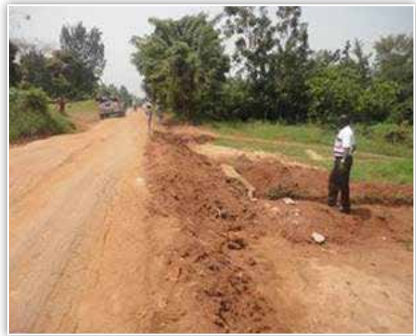
Poorly constructed headwalls that needed raising to the new road level.
