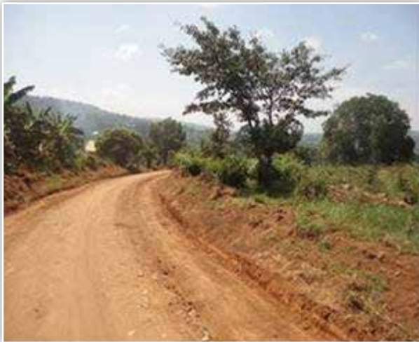
Masaka DLG: Sharp corners on the graded and shaped sections of Bulayi- Kigaato- Kiyimba road (5km) lacking road safety signposts.
