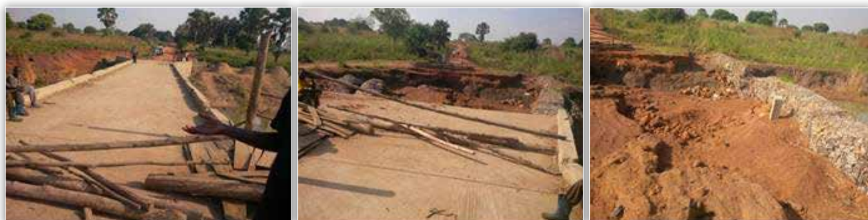
Yumbe DLG: Sections of Kochi Vented Drift Bridge where the guardrails and approaches had been swept following flash floods.
