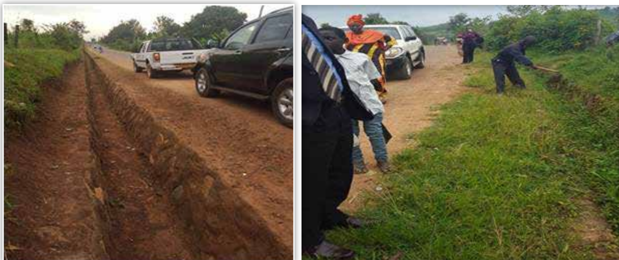
Mbale MC: Inspection of routine manual maintenance contractors carrying out grass cutting and de-silting of side drains of the Municipal network
