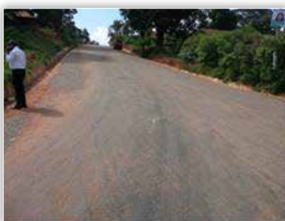
Entebbe MC: Sections of Sewabuga road, which received resealing and lining of side drains. Surface failures were seen (L) and (C) at start of the road.
