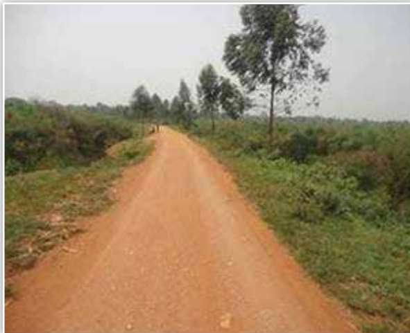
Mukono DLG: Restored section of Sezibwa swamp at ch 6+500 on Kabimbiri- Nkoko- Kyabazala road (12km) that had been washed away by heavy floods.
