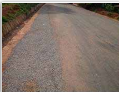
Entebbe MC: Sections of Sewabuga road, which received resealing and lining of side drains. Surface failures were seen (L) and (C) at start of the road.
