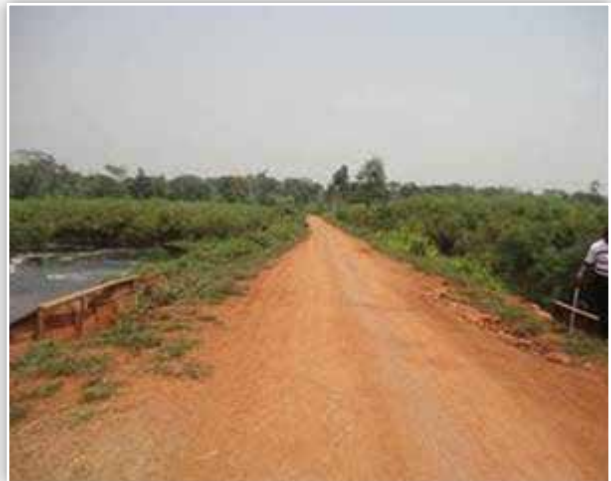
Mukono DLG: Restored section of Sezibwa swamp at ch 6+500 on Kabimbiri- Nkoko- Kyabazala road (12km) that had been washed away by heavy floods.
