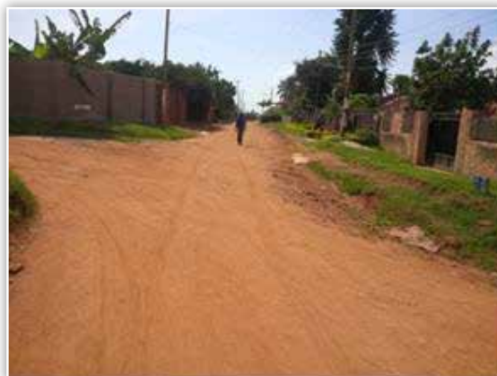
Entebbe MC: Sections of Kiwafu Close, which received routine mechanised maintenance – essentially grading.
