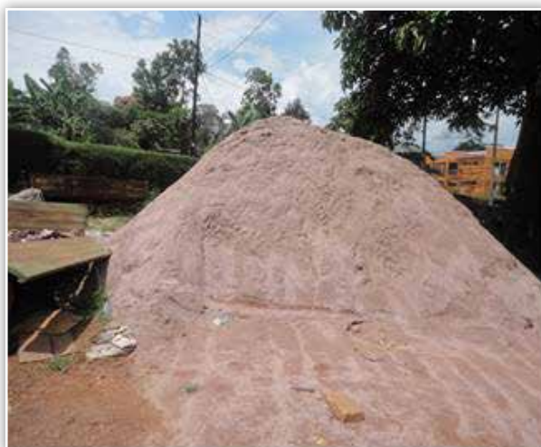
Mukono MC: Sand and stone dust materials procured for the second seal on the 1km section of Nabuti- Nsube road (5km)
