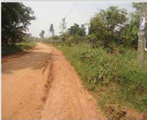
Mukono DLG: Section of Kanana-Nacyeke-Luguje (8km) requiring erosion protection in road side drains.
