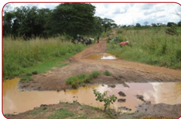
Pader DLG: Pajule – Amoko, 25.5Km; Installing cross culverts required.
