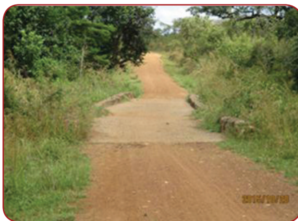
Kitgum DLG: Kitgum Matidi – Mucwini, 19Km; Bridge at Km3.35 requiring warning signs, erection of barriers and river training.
