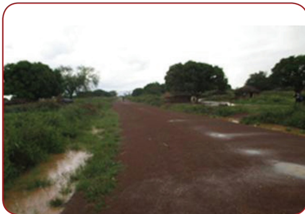
Agago DLG: Agago Town Council roads; Poor drainage requiring improvement.
