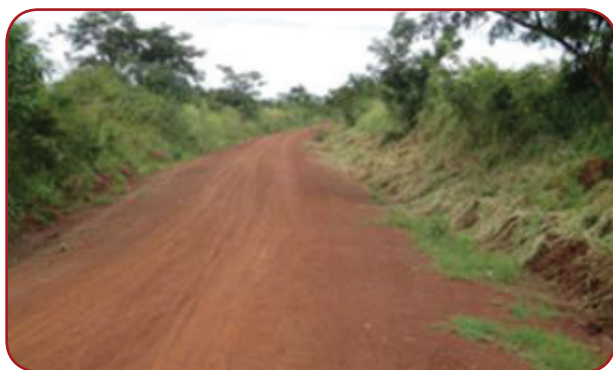
Lamwo DLG: Ogwec – Awenolwiyo, 18.1Km; Road in good condition though windrow left in side drain.
