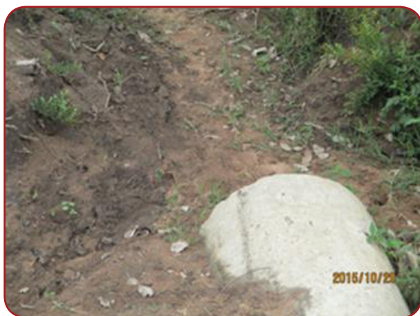
Otuke DLG: Olilim Training Centre – Aluga Primary School, 8Km; Culvert need reinstallation with proper inverts.
