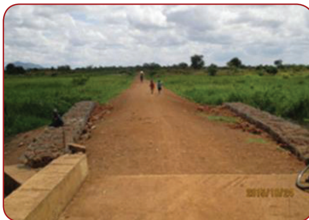
Kitgum UNRA: Padibe – Paloga – Madiope, 35Km; Improved swamp crossings using gabion boxes.
