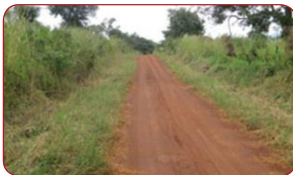
Lamwo DLG: Ogwec – Awenolwiyo, 18.1 Km; On-going grass cutting but width and height need addressing.
