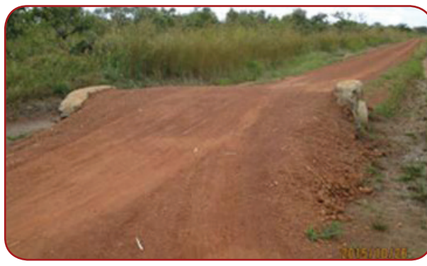
Pader DLG: Lanyatido – Koyo – Lalogi, 27Km; gentle approaches needed for cross culverts.
