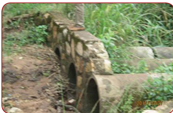
Agago DLG: Kalongo – Lumoi, 30Km; Washed away culvert crossing that need urgent repairs.
