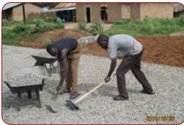
Otuke DLG: Otuke town council roads; Sweeping away loose aggregates after surface dressing Daniel Omara Atubo Avenue.
