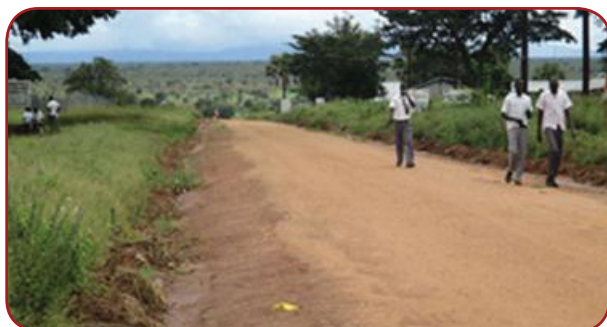
Kitgum UNRA: Namokora - Adilang, 74Km; Windrow left in side drain.
