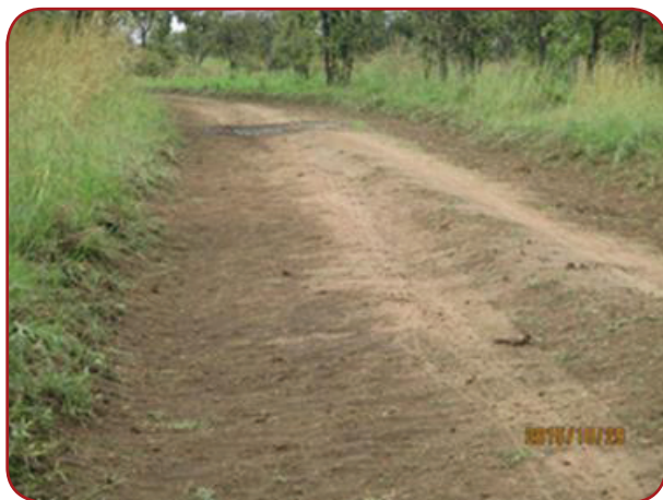
Otuke DLG: Okung Primary School – Aler Primary School, 6Km: Well done grubbing.
