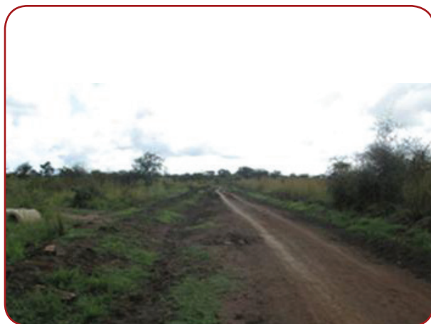
Agago DLG: Agago – Lapono, 20Km; A section made of black cotton soils requiring gravelling.
