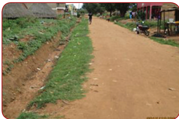
Kitgum DLG: Irene Gleeson road, 2.7Km; Well-maintained side drain
