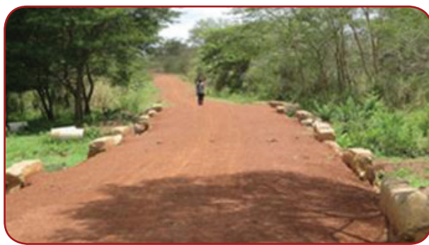
Kitgum DLG: Anyima – Lagot, 12.6Km; Well raised swamp crossing though river training required.
