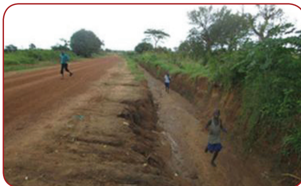
Kitgum UNRA: Kitgum Matidi - Kalongo - Patongo, 77Km; Repaired road section and excavated channel in Kalongo Township.
