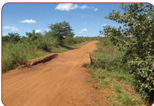
Kitgum DLG: Oryang – Ojuma – Kitgum Matidi, 16Km; Road in good condition, bridge warning signs should be erected.
