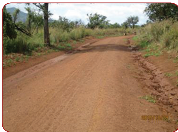
Otuke DLG: Teopok – Alir, 8.5Km; Road well graded but not compacted.
