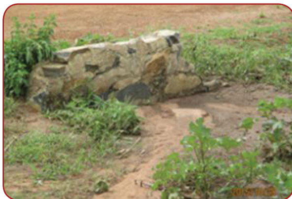
Otuke DLG: Otuke town council roads; Drainage system need correction to avoid easy siltation.
