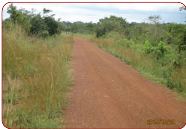
Otuke DLG: Otuke Town council – River Moroto, 8Km; Road in good condition though bushy affecting drainage.
