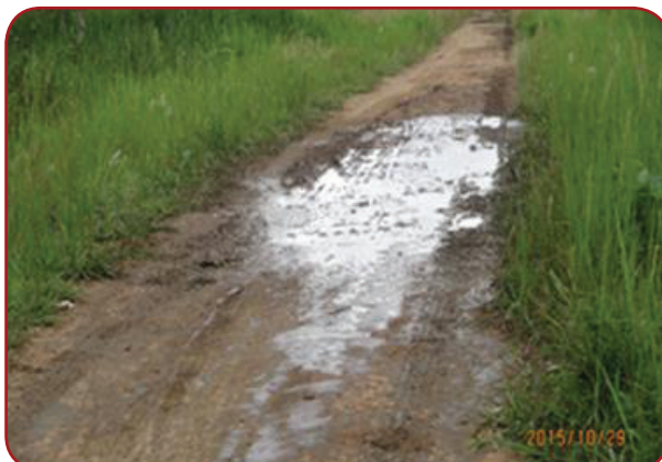
Otuke DLG: Otuke Town council – River Moroto, 8Km; Because of failure of water to get to side drains, road developing potholes.
