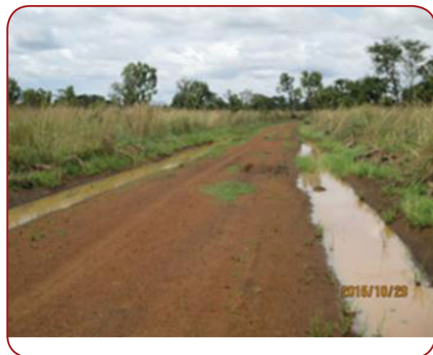
Otuke DLG: Teopok – Alir, 8.5Km; Because of the lack of offshoots, there is stagnation in the side drains.
