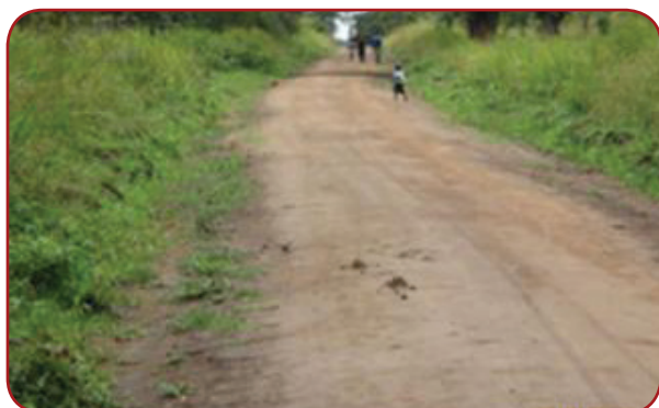
Lamwo DLG: Olebi – Pakalabule Lamwo TC, 2.7km; Road in good condition just requiring routine manual maintenance.
