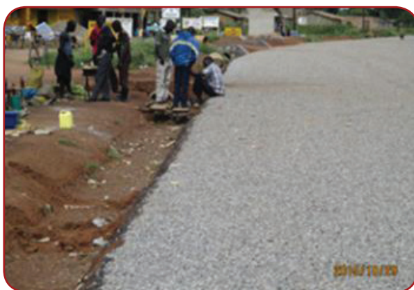
Otuke DLG: Otuke town council roads; A well provided side drain awaiting stone pitching.
