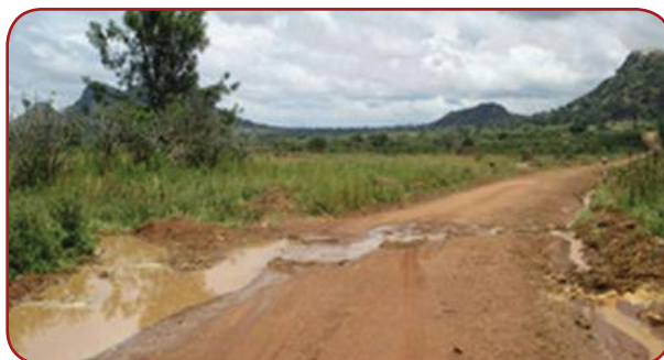
Kitgum UNRA: Namokora - Adilang, 74Km; Drainage improvement required.
