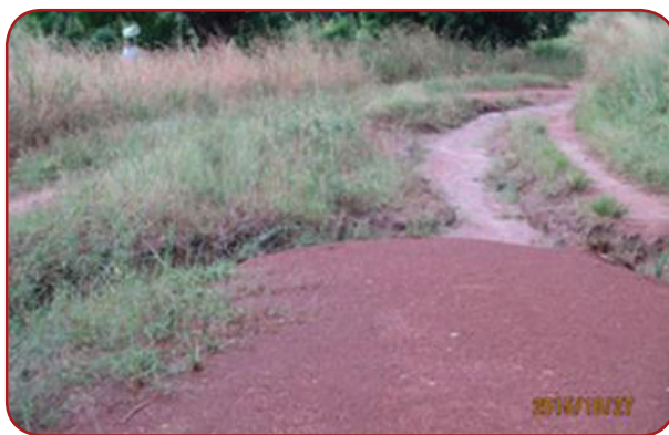
Agago DLG: Kalongo Town Council roads; Need for drainage improvement as to avoid gross erosion.
