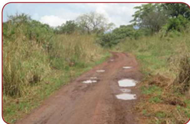
Pader DLG: Pajule – Amoko, 25.5Km; Road in poor condition with many developing potholes.
