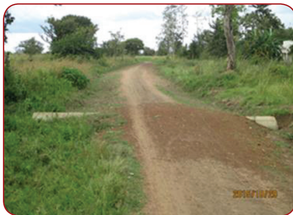
Otuke DLG: Olilim Training Centre – Aluga Primary School, 8Km; Culverts need reinstallation
