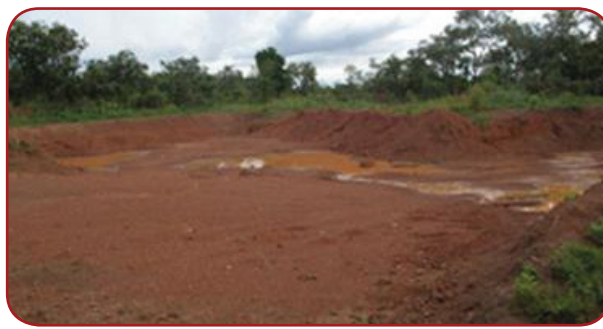
Pader DLG: Lanyatido – Koyo – Lalogi, 27Km; Bor- row pits were not reinstated.
