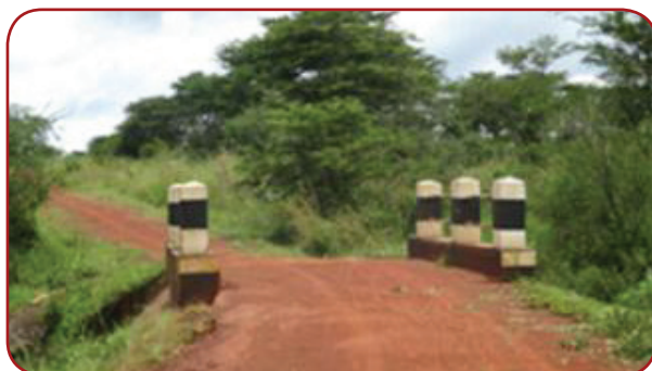
Lamwo DLG: Olebi – Lelapwot, 9.0Km: Pagada bridge requiring warning signs and river training.
