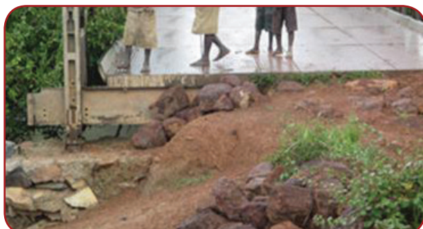
Pader DLG: Atanga – Bolo – Lagile, 38Km; Ocwidia bridge gets submerged approaches grossly eroded.
