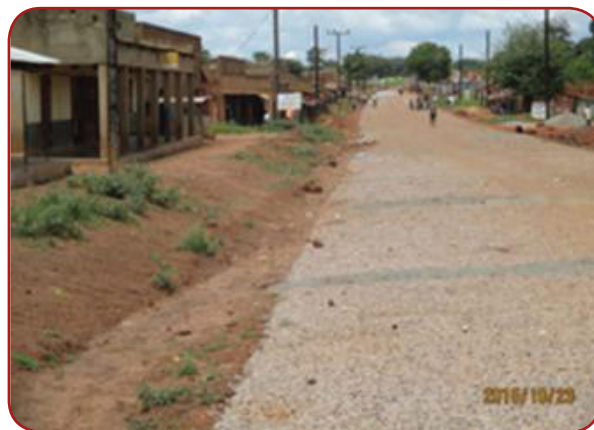
Lamwo DLG: Kitgum – Ngomoromo, Lamwo TC, 450m; Road surface dressed but drainage works not yet carried out.
