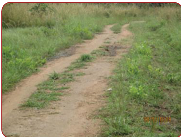
Otuke DLG: Okung Primary School – Aler Primary School, 6Km: Road recently graded but not compacted, need to manage grass growth.
