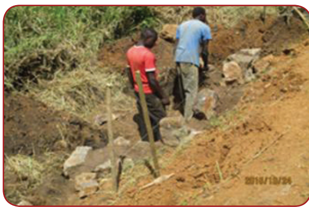
Kitgum UNRA: Potika – Ngomoromo, 37Km; Culvert end structures being constructed.
