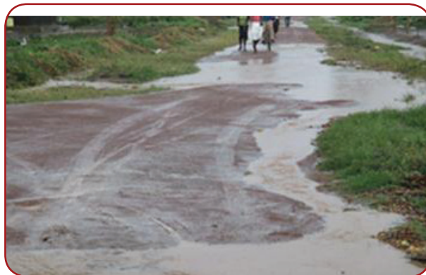
Agago DLG: Patongo Town Council roads; Drainage improvement required.
