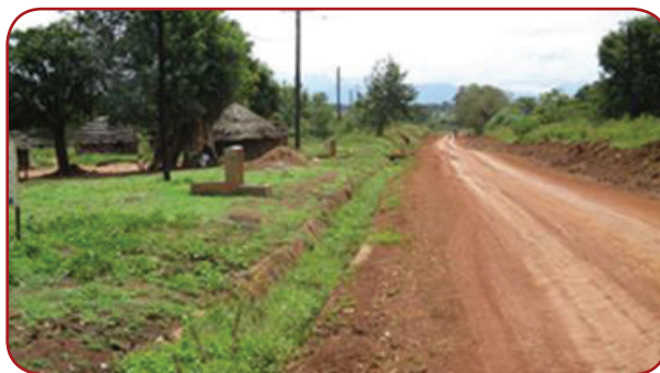
Kitgum UNRA: Kitgum - Orom 90km; Line drains need cleaning.
