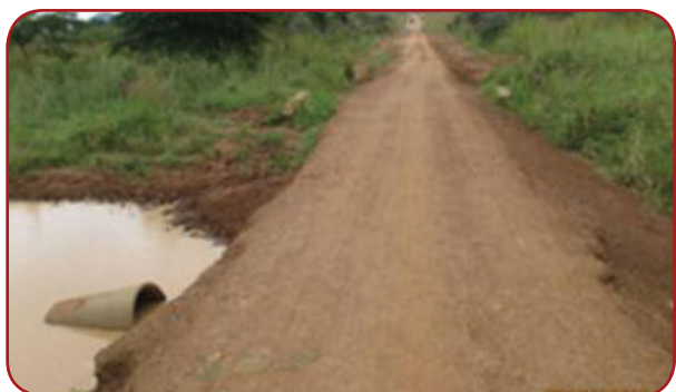
Kitgum UNRA: Namokora - Adilang, 74Km; Swamp crossing embankment at Km41.7 require urgent repair.
