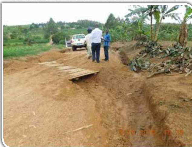
A temporary wooden crossing set up by the community to cope with the damage caused by fast flowing rain water on Igorora – Kigando road.
