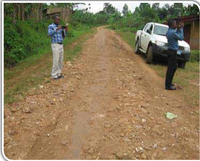
Bududa district: A section on Bududa-Busano road that had received spot gravelling using coarse gravels from Bukibokolo borrow pit.
