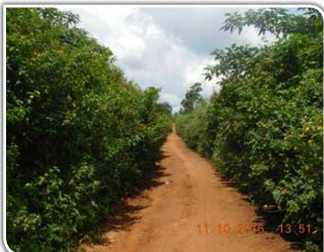
Kiyinja – Lwebyayi road overgrown with vegetation. The road received light grading but no routine manual maintenance intervention during the year.
