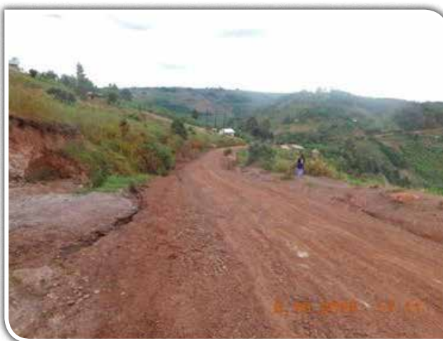
Slippery ash rock covered with gravel on Rwizi – Kikunda – Omukatojo road
