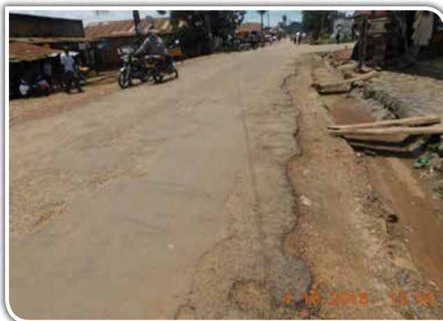
Jubilee Street (1Km) received pothole patching. Potholes are persistent at many sections and the curb/shoulders are worn
