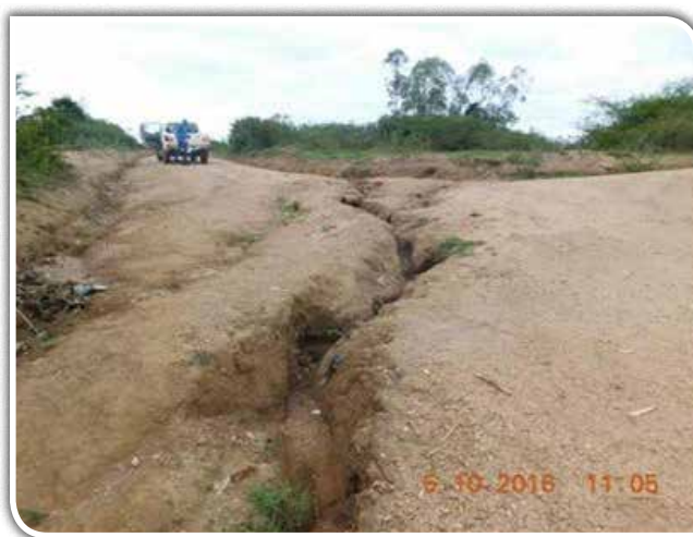
Deep erosion at the beginning of Zaituni Rd in need of a cross culvert.
