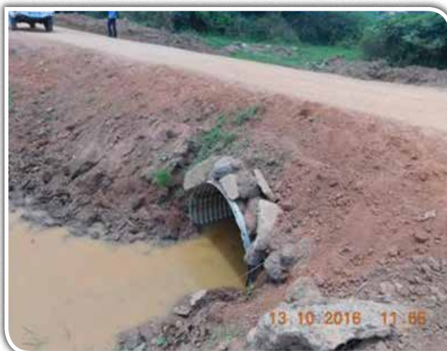
Construction of culvert end structures delayed due to lengthy procurement process which was still ongoing at the time of the field visits.
