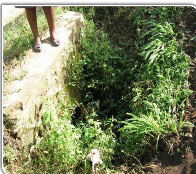
Manafwa district: Culvert end structures overgrown with vegetation on Bututu-Magale road. Road gangs were not in operation as their appointment letters had not yet been signed due to transfer of the CAO.
