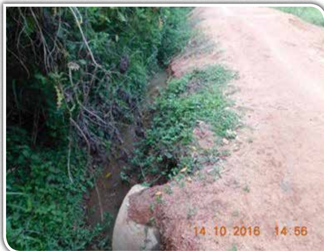
Swamp-raising on Pearl – Kangulumira Rd in Q4 FY2015/16. Construction of culvert end structures and compaction of backfill needed.
