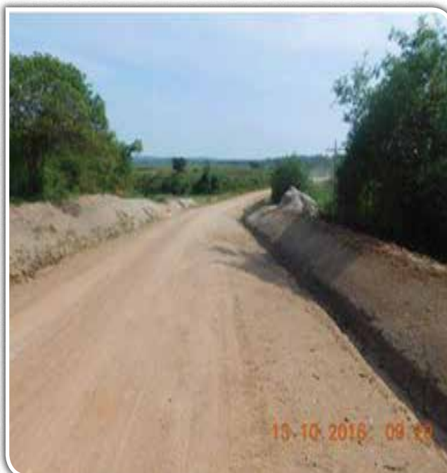
Grading and gravelling was undertaken on 24Km while 14Km received only grading works on Lusarira – Kasambya Road under Term maintenance by Hands (U) Ltd.
