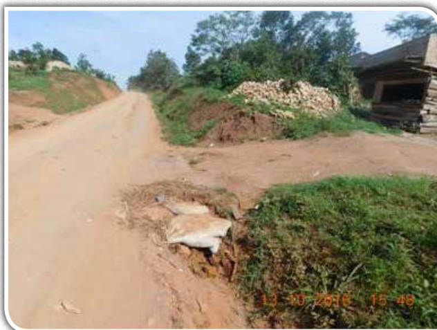
Side drains blocked by residents to create access on Kasanda-Madudu Rd (20Km) which underwent routine mechanised maintenance in Q3-4 FY2015/16 by Force Account.
