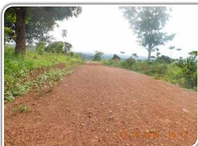
Mirembe – Lwamasanga road after grading, widening and gravelling works in Q4 FY2015/16.
