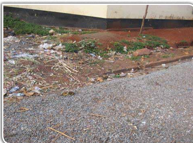
Jinja MC: Parekh road (0.75km) resealed under PM using double surface dressing. There was a challenge of vendors dumping refuse at market areas which was blocking the covered side drains through the road kerb inlets. Wire mesh should be put at the inlets to protect the covered side drains.
