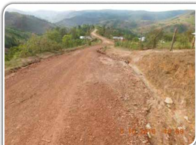
Gravel loss due to rain on a hilly section of Busherewe – Rwentojo – Bugamba road (2km) which underwent grading and gravelling in Q4.
