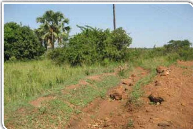
UNRA Soroti: A windrow from graveling operations whose improperly disposed of material was falling into the nearby mitre drain on Arapai-Amuria road (28km).
