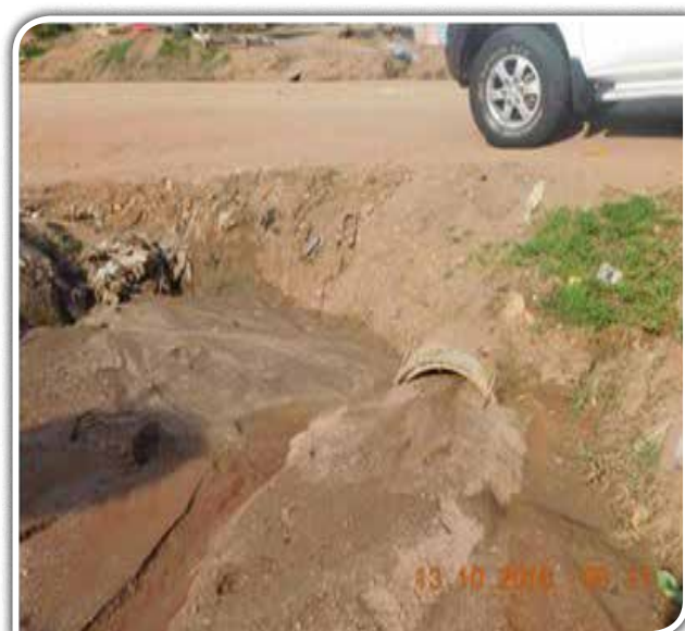
Silted side drains and blocked culverts on Lusarira – Kasambya Rd indicating absence of manual maintenance interventions
