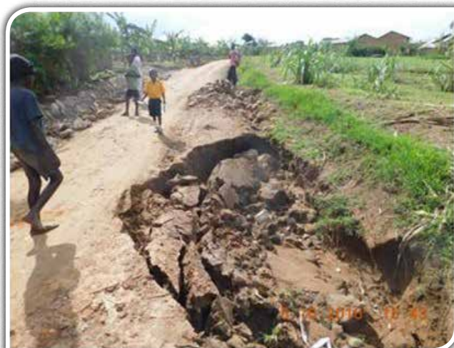
A section of Igorora - Kigando road which collapsed due to rain damage. Stone pitching is to be undertaken in FY2016/17 to strengthen the side drains.
