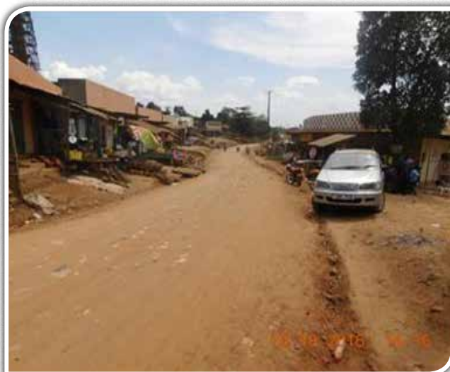
Kirungi – Kangulumira road (1.5 Km) underwent grading and gravelling in Q1 FY2015/16. The side drains on most sections of the road were silted and in need of manual maintenance.
