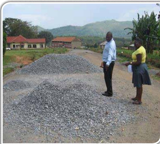
Manafwa TC: Heaps of 14/20mm and 10/14mm aggregate to be used for sealing a primed section on Wesonga road (0.56km)
