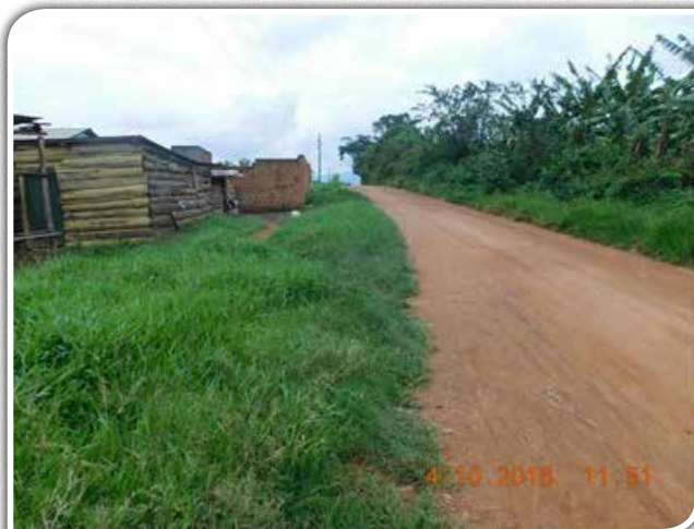
Kasharara road (1.2 Km) received grading and shaping works in Q2. Due to lack of routine manual maintenance, most of the cross culverts are blocked leading to flooding of low lying sections when it rains.
