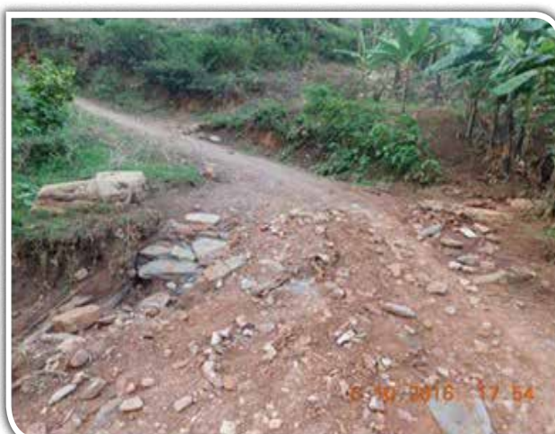
Rock debris deposited on the road by runoff water from the hills on Kashekuro-Nkonkoma-Ikumba road (22km grading in Q4). The capacity of the culvert crossings cannot contain the volume of the runoff during heavy rains.
