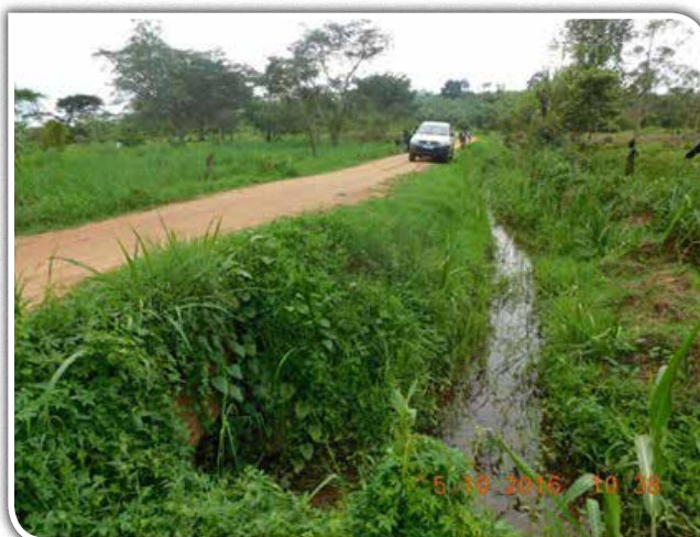
Swamp raising and excavation of side drains on Kakinga – Kololo Rd done by road gangs in Quarter 1 FY2015/16
