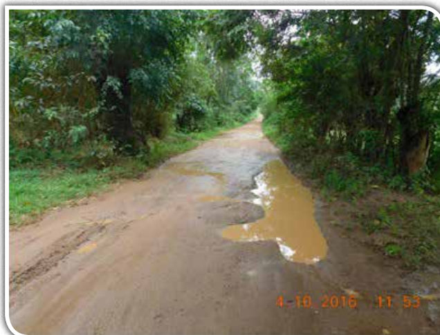
Kasharara road (1.2 Km) received grading and shaping works in Q2. Due to lack of routine manual maintenance, most of the cross culverts are blocked leading to flooding of low lying sections when it rains.
