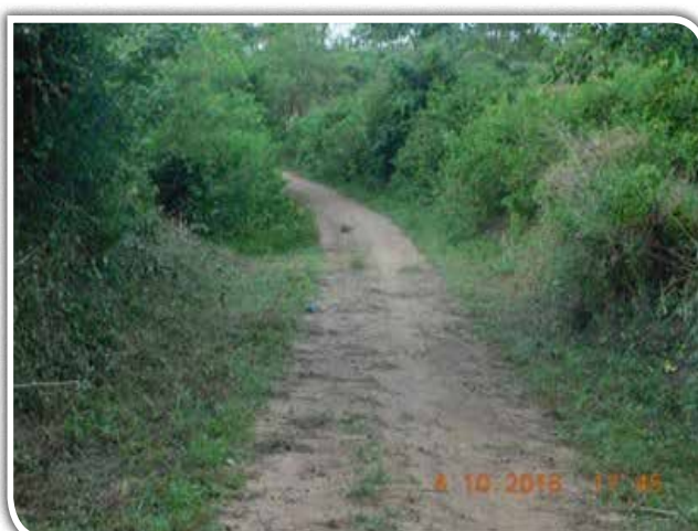
Katikamwe-Rushango P/S-Karokarungi (4.2Km) received grading and spot gravelling. Sections of the road were bushy and in need of bush clearing.
