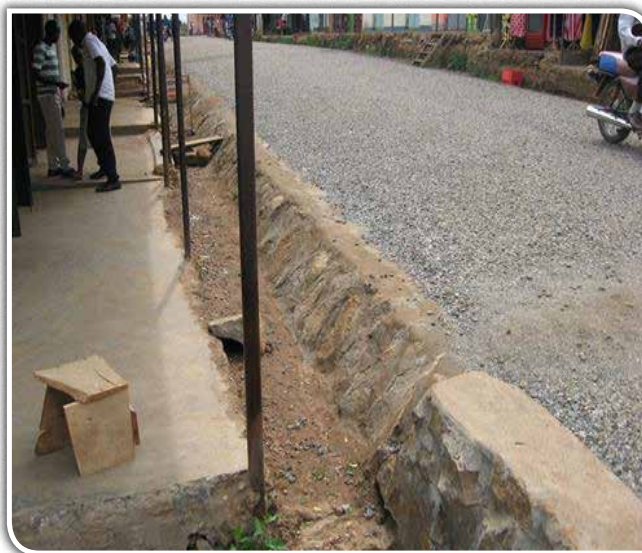
Manafwa TC: A fully sealed section (double surface dressing) on Market road (0.19km) including stone pitching.
