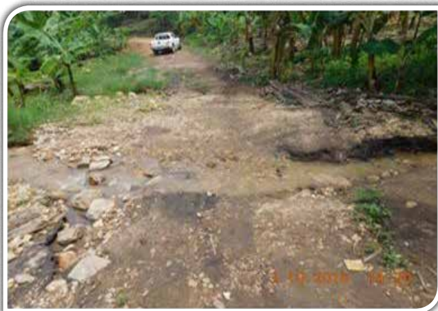
Rocks excavated during gold mining are later washed onto the road damaging it.
