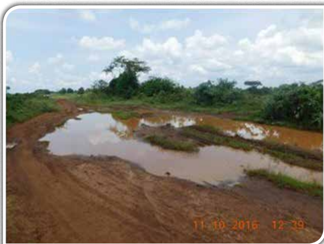
Water logged section of Butta – Namuguxa road due to lack of provision for drainage during periodic maintenance.
