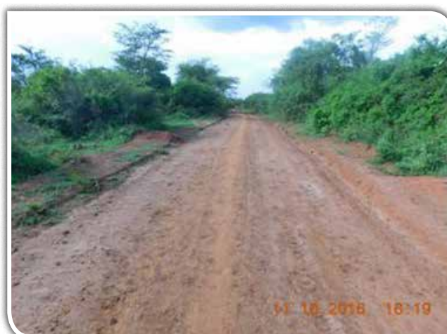
A section that was graded and widened pending release of additional funds for gravelling works.
