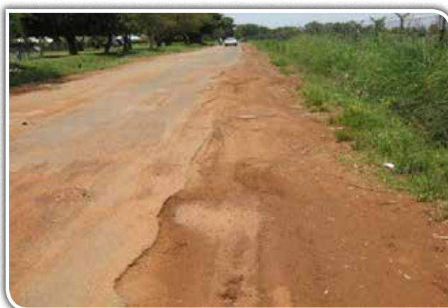
UNRA Soroti: Base and edge failures on Soroti-Arapai Railway Station road (10km). The pothole patches were so extensive and recurrently done pointing to a weakened pavement structure.
