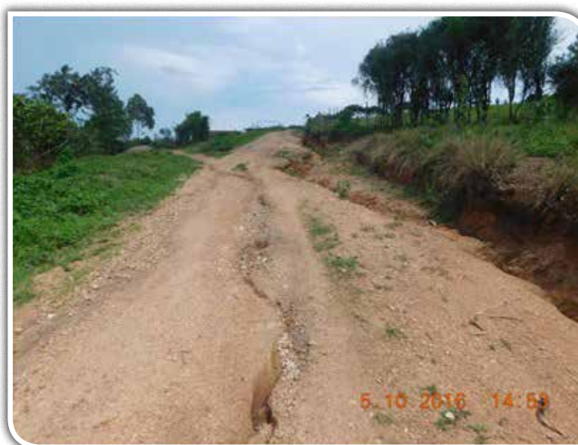
A gullied section of Igorora – Kabobo Road. The road received grading and spot gravelling in Q1 FY2015/16
