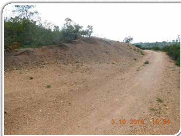
Gravel stockpile of Rushango-Omukahate road (11 km) under periodic maintenance. Due to delayed implementation, some of the stockpiled gravel was washed away during rains.
