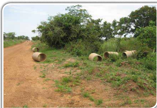
UNRA Soroti: Culvert pieces deposited on Arapai-Amuria road (28km) by a periodic maintenance contractor called KOL Services Ltd. Culvert installation works stalled as a result of the contractor attending to other roads under UNRA concurrently.
