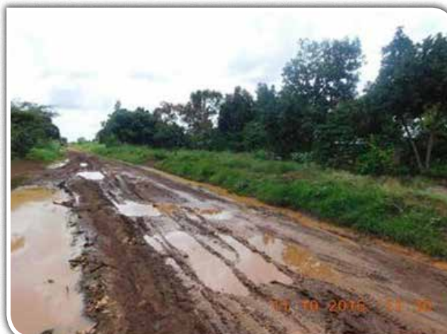
Waterlogged section of Butta-Namuwunguza. Planned culvert line was not installed because the landowner was against water draining into his land.
