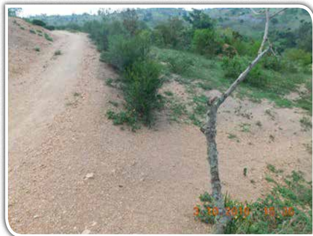
Gravel stockpile of Rushango-Omukahate road (11 km) under periodic maintenance. Due to delayed implementation, some of the stockpiled gravel was washed away during rains.
