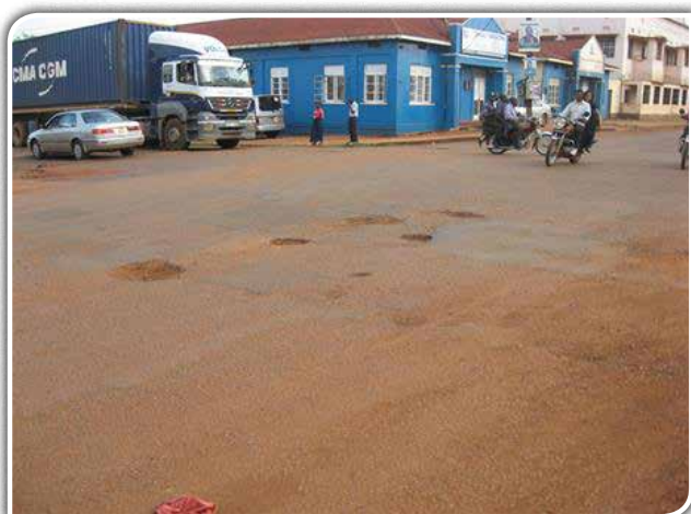
Jinja MC: A major junction on Gabula road (0.9km) that had received extensive recurrent pothole patching under RMeM. There was glaring need to use a cement concrete surface at the junction to withstand the heavy loading imposed by slow moving trucks.
