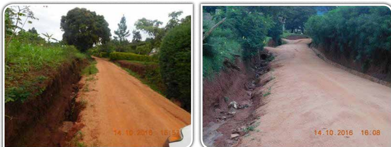
Kikoona-Katawa Rd (left) and Church Road (right) which received grading and spot gravelling in Q1 FY2015/16 need stone pitching of side drains to prevent erosion of road edges by runoff during the rainy season.
