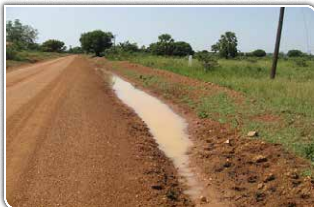
UNRA Soroti: Water ponding in the side drain on Arapai-Amuria road (28km) as a result of difficulty in locating point of free disposal of mitre drains. The road is located in flat terrain typical of such drainage difficulties.
