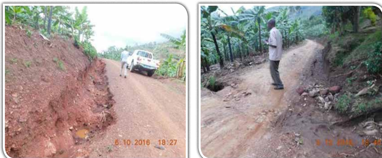
Some of the sections of Kashekuro-Nkonkoma-Ikumba (22Km) which were damaged by runoff. The road was graded in Q4 FY2015/16.
