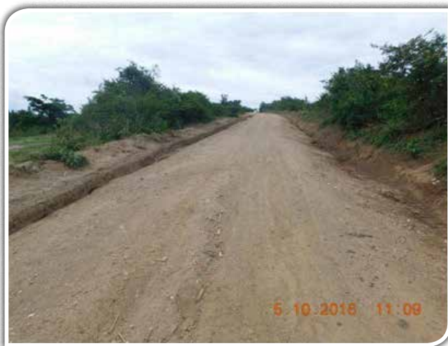
Zaituni Rd (2.8Km) received bush clearing, spot gravelling and grading works in Q1 FY2015/16
