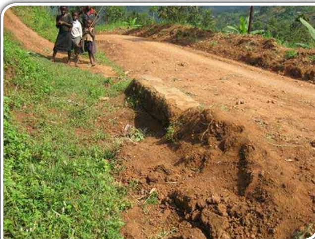
Bududa district: Deliberate blockage of cross culvert inlets on Nalufutu-Shanzou road (11.1km) by locals to prevent water from being discharged into their gardens at the outlet side.
