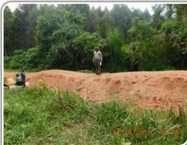
Swamp-raising on Pearl – Kangulumira Rd in Q4 FY2015/16. Construction of culvert end structures and compaction of backfill needed.
