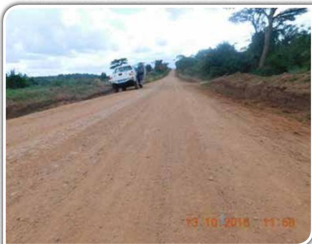
Grading, road widening, spot gravelling, swamp filling were undertaken on Kitenga – Musozi Rd (18Km) under Force Account in Q1 & Q4 FY2015/16.
