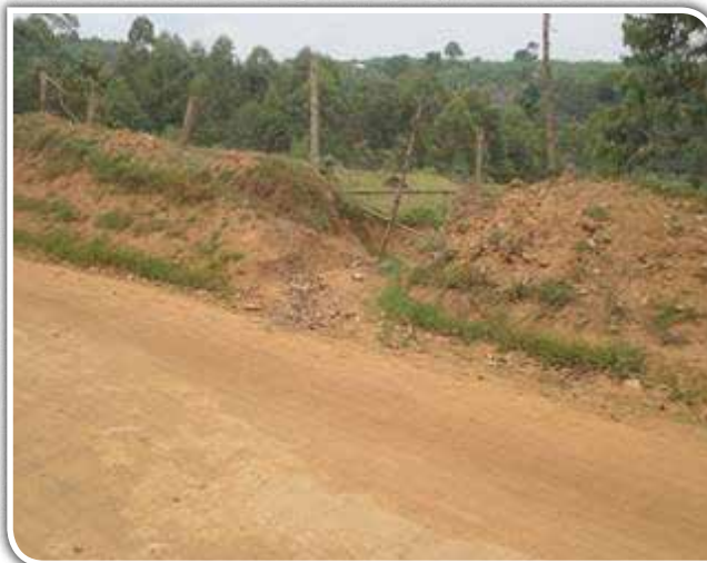
Poorly excavated offshoots headwalls that rise above the carriageway
