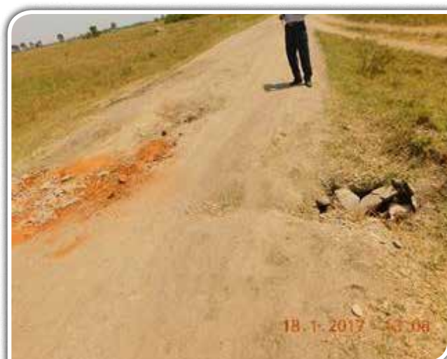
Ntoroko district: A broken culvert crossing on Rwebisengo-Rwangara road for which procurement was ongoing
