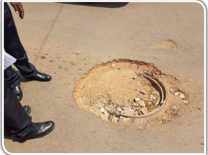
KCCA Central Division: William Street – a section received an overlay but NWSC Sewerage loose manhole in the middle of the road presents a weak point which keeps damaging the carriageway.
