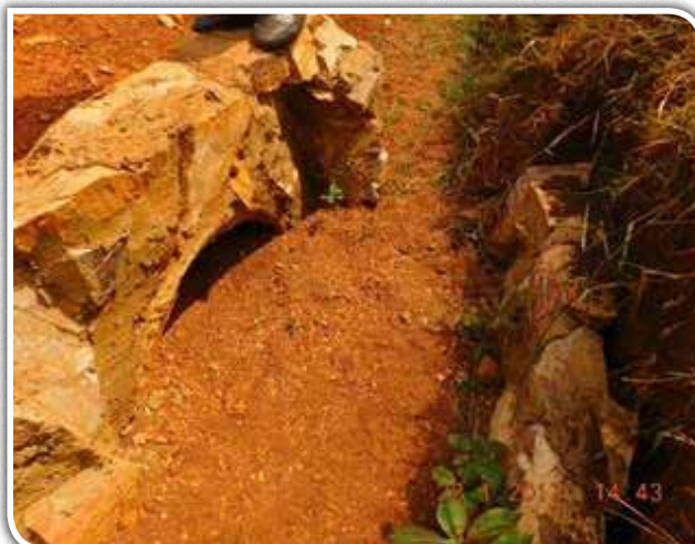
Kyarusozi Town Council: A silted culvert inlet due to challenges in channeling water to private land at the outlet
