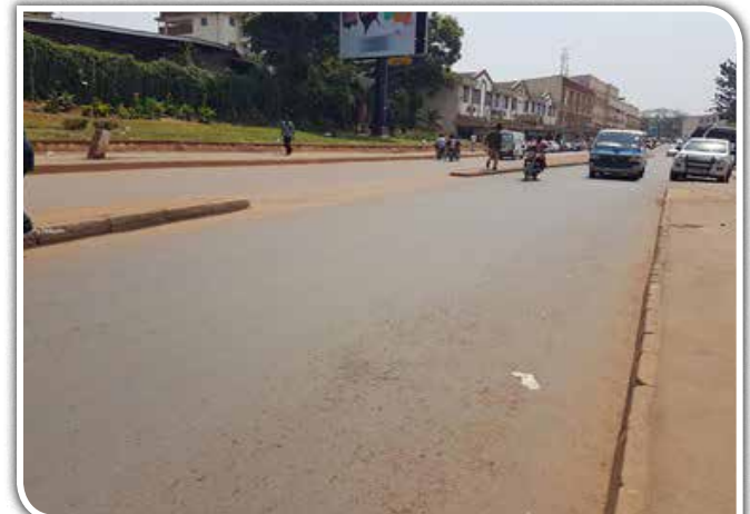
KCCA Central Division: Sections along Bombo Road which received an asphalt overlay as part of the mechanised maintenance
