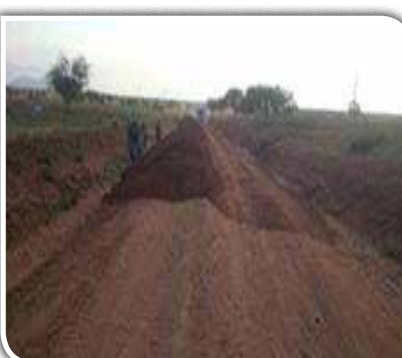
UNRA Moroto: Sections of Iriri - Nadunget road which was undergoing regravelling using term maintenance contracts.
