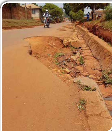
KCCA Nakawa Division: Ismail lane – narrow carriage way and inadequate drainage. Works planned for Q3 of FY 2016/17
