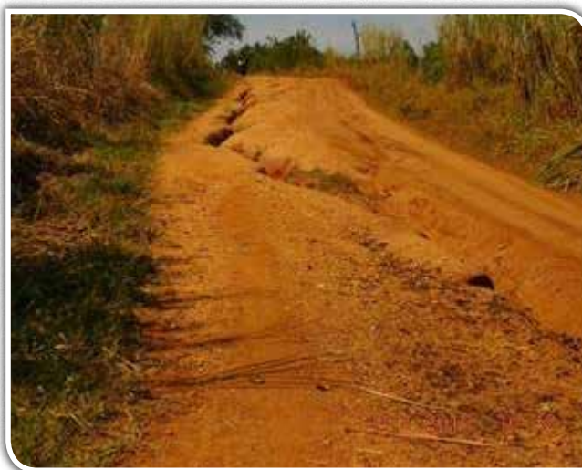
Kyegegwa district: Gulleys developing along Kyakabara – Hapunyo road due to lack of routine maintenance
