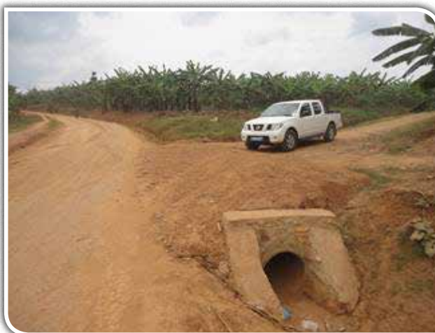
Newly constructed 600mm diameter culvert line 12m at the junction with a district road.
