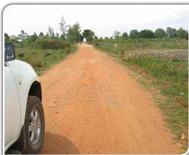
Mbale district: A section on Doko-Kabwangasi road (6.0km) that was reshaped under RMeM.
