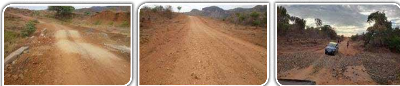
UNRA Moroto: Sections of Moroto – Rupa - Nakabat road, which was worked on using force account. (L) Newly installed culverts; (R) a typical non-vented drift with rubble deposits along the road
