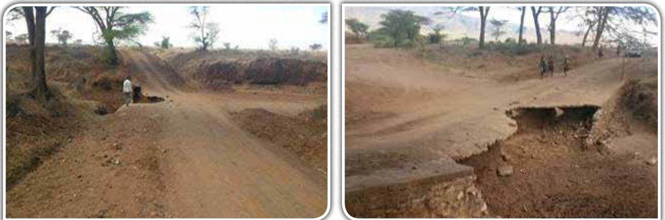
Moroto DLG: A collapsed drift at 3.2Km along Naoi – Lokisilei – Kobebe road, which was too dangerous to traffic on the road.
