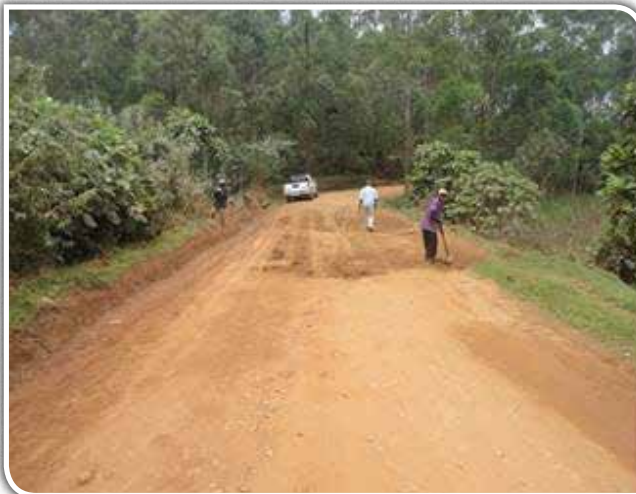
Bushenyi DLG: Completed sections of Nyakasiro – Nyarugote – Butare (11.5km) undergoing routine manual maintenance.
