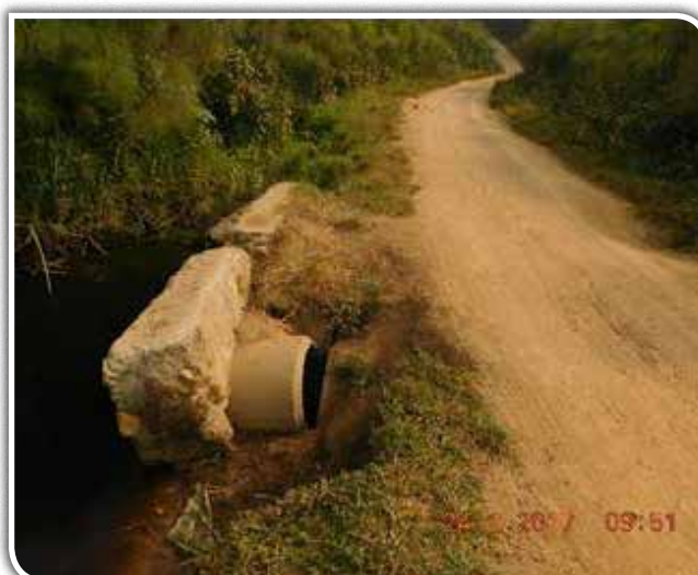
Kyegegwa district: Broken culvert headwall on Rwabategura swamp road
