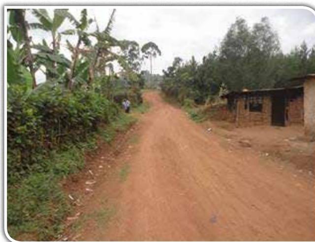
Kabale DLG: Sharp corners on the graded and shaped sections of Kitumba-Habuhasha road (6km) lacking road safety signposts.
