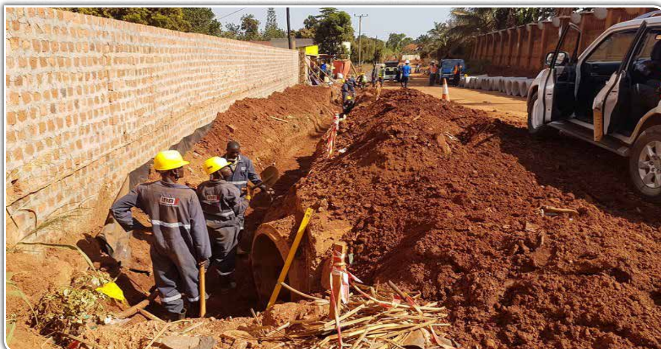
KCCA Makindye Division: Excavation for drainage works along Kalungu Road (2.5km) – Contracted out to IBBI International Ltd and Supervising Consultant is UB Consulting Engineers
