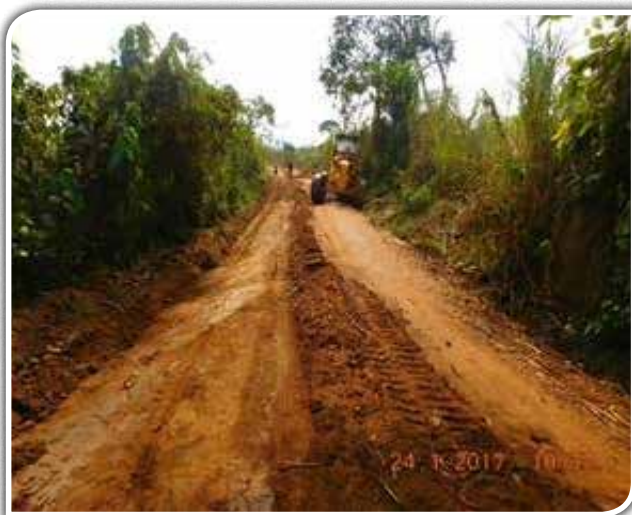
Kyegegwa district: Ongoing mechanised maintenance on Kyamanya-Kyanyambali road. The work was deferred from Q1
