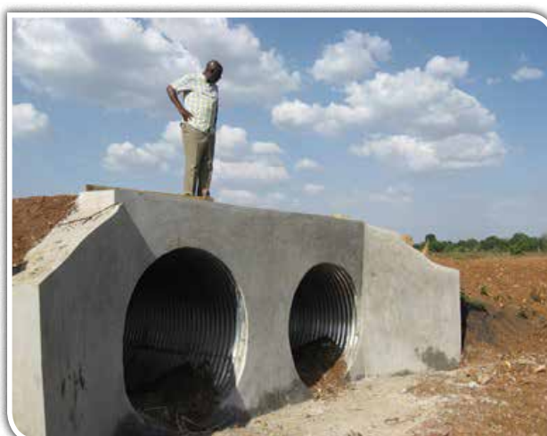
Iganga district: Spot improvement at a swamp on Mwendafuko community access road (10km). A double line 1,800mm diameter culvert was installed.
