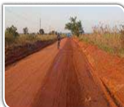
UNRA Moroto: Sections of Iriri - Nadunget road which was undergoing regravelling using term maintenance contracts.
