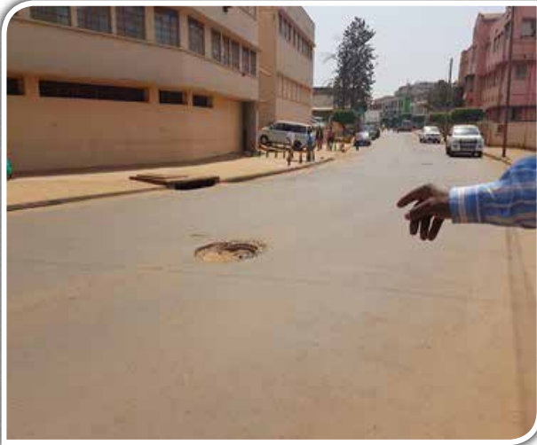
KCCA Central Division: William Street – a section received an overlay but NWSC Sewerage loose manhole in the middle of the road presents a weak point which keeps damaging the carriageway.
