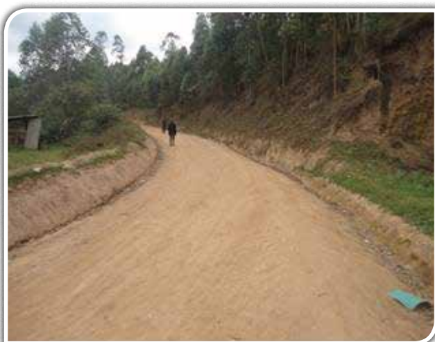
Kabale DLG: Sharp corners on the graded and shaped sections of Kitumba-Habuhasha road (6km) lacking road safety signposts.
