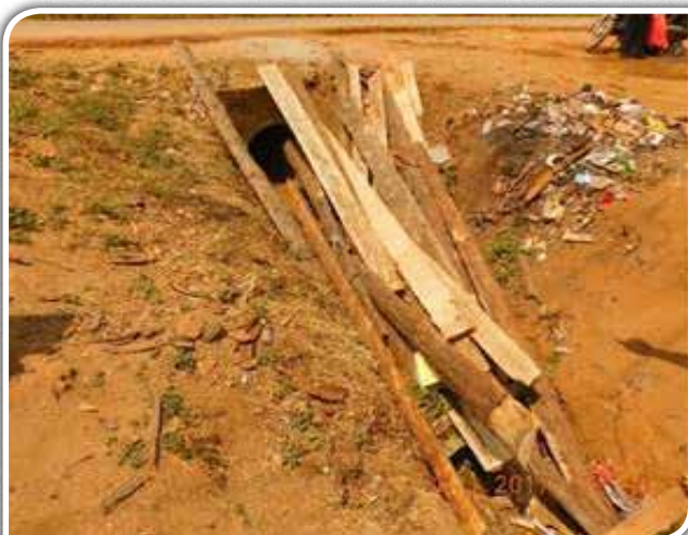
Kyenjojo Town Council: Culvert crossing on Kyenjojo-Kagadi road. Dumping is common in the TC and this blocks drainages
