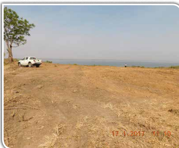
UNRA Fort Portal: A re-instated gravel borrow pit in Kanara Town Council. The gravel was used for F/A works on Karuguto – Ntoroko road using hired equipment.
