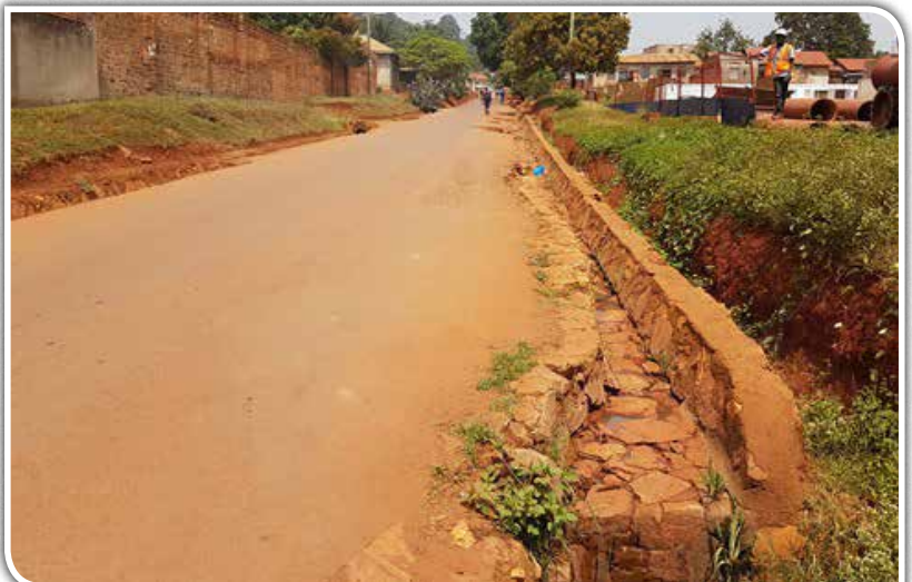
KCCA Nakawa Division: Ismail lane – narrow carriage way and inadequate drainage. Works planned for Q3 of FY 2016/17
